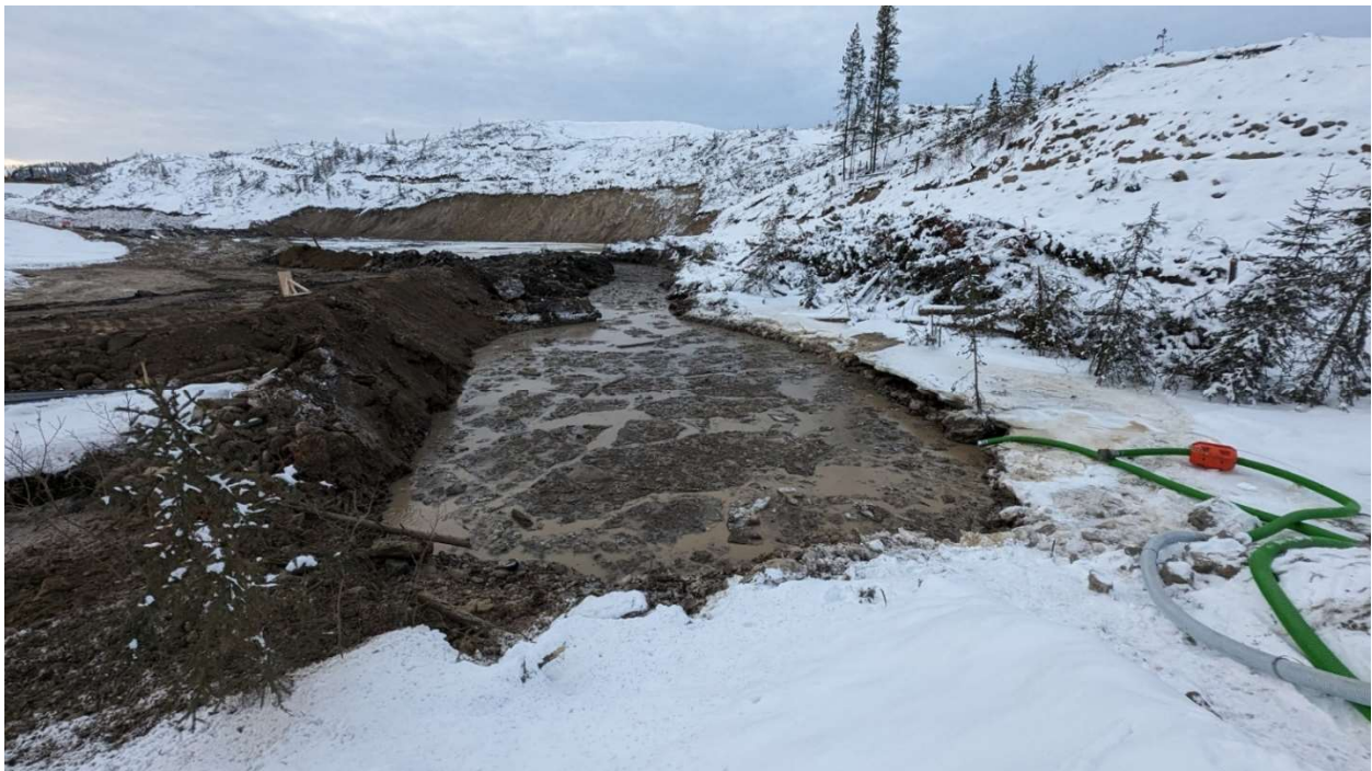
Photo 2: Source of sediment laden water at the TSF work front.
