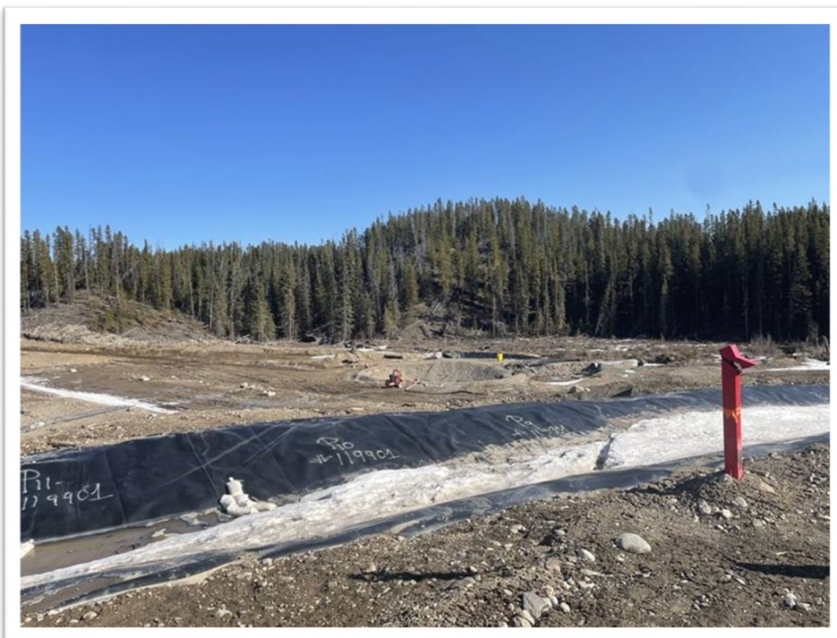
Photo 21: Interim Environmental Control Dam Emergency Flow Spillway
