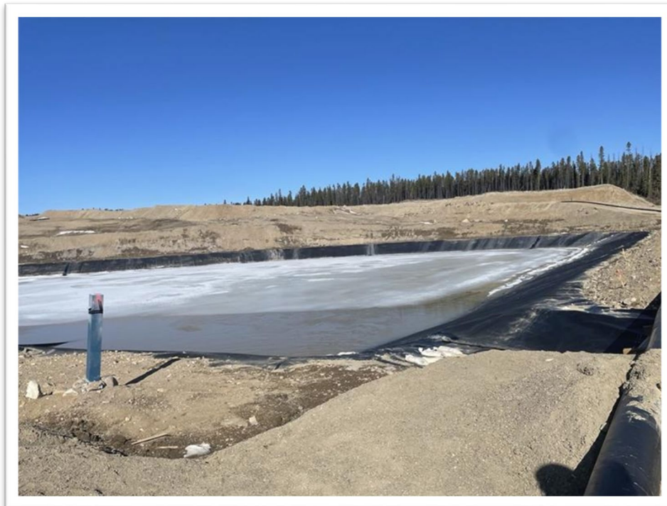
Photo 19: Interim Environmental Control Dam
