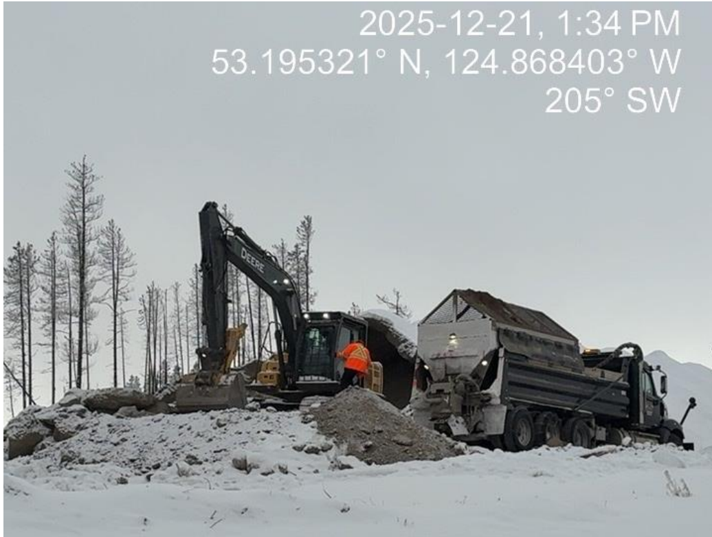
Photo 16: Excavator Loading a Sand Truck
