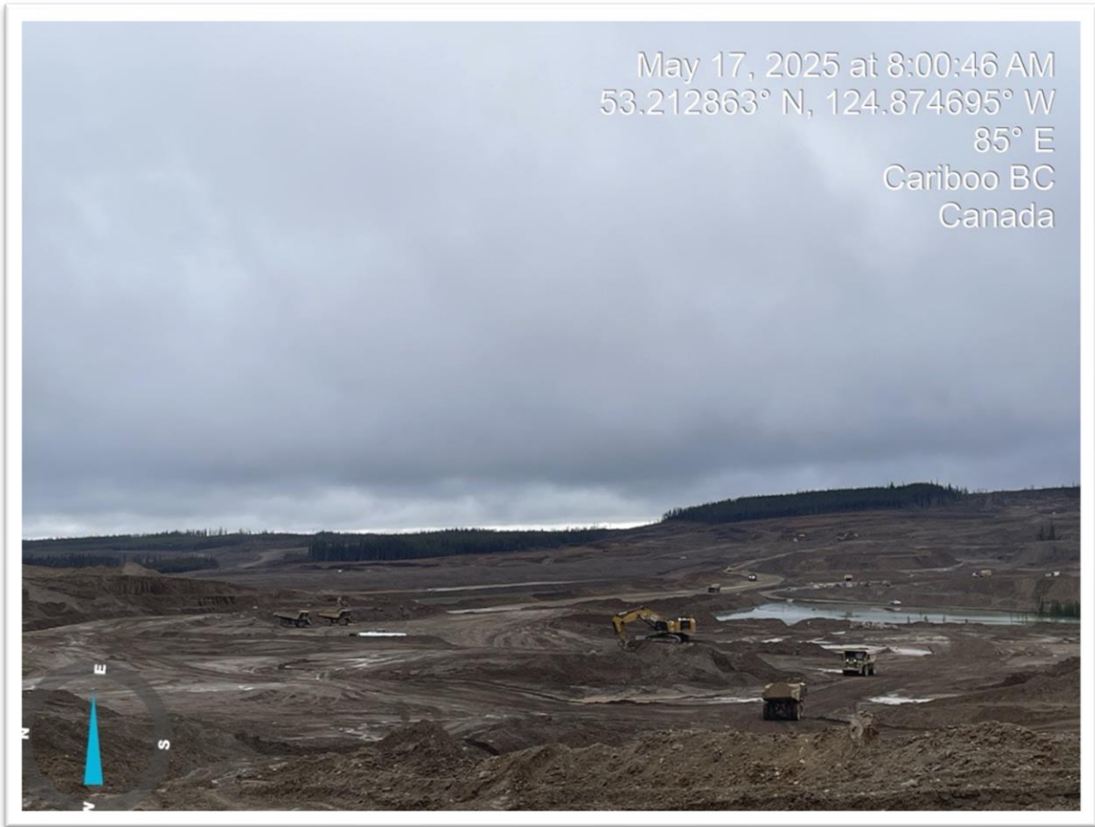
Photo 45: Tailings Storage Facility
