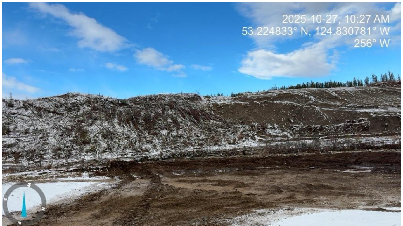
Photo 16: Fresh Water Reservoir
