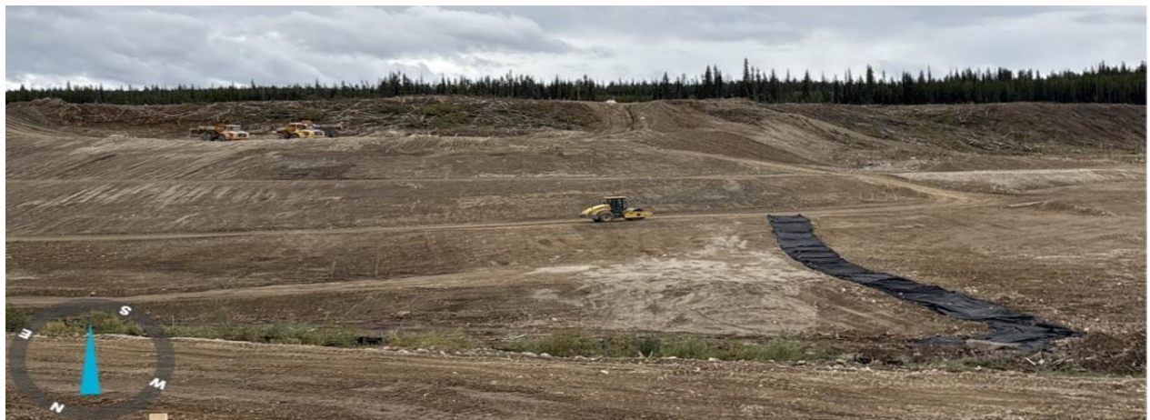
Photo 4: Fresh Water Reservoir
