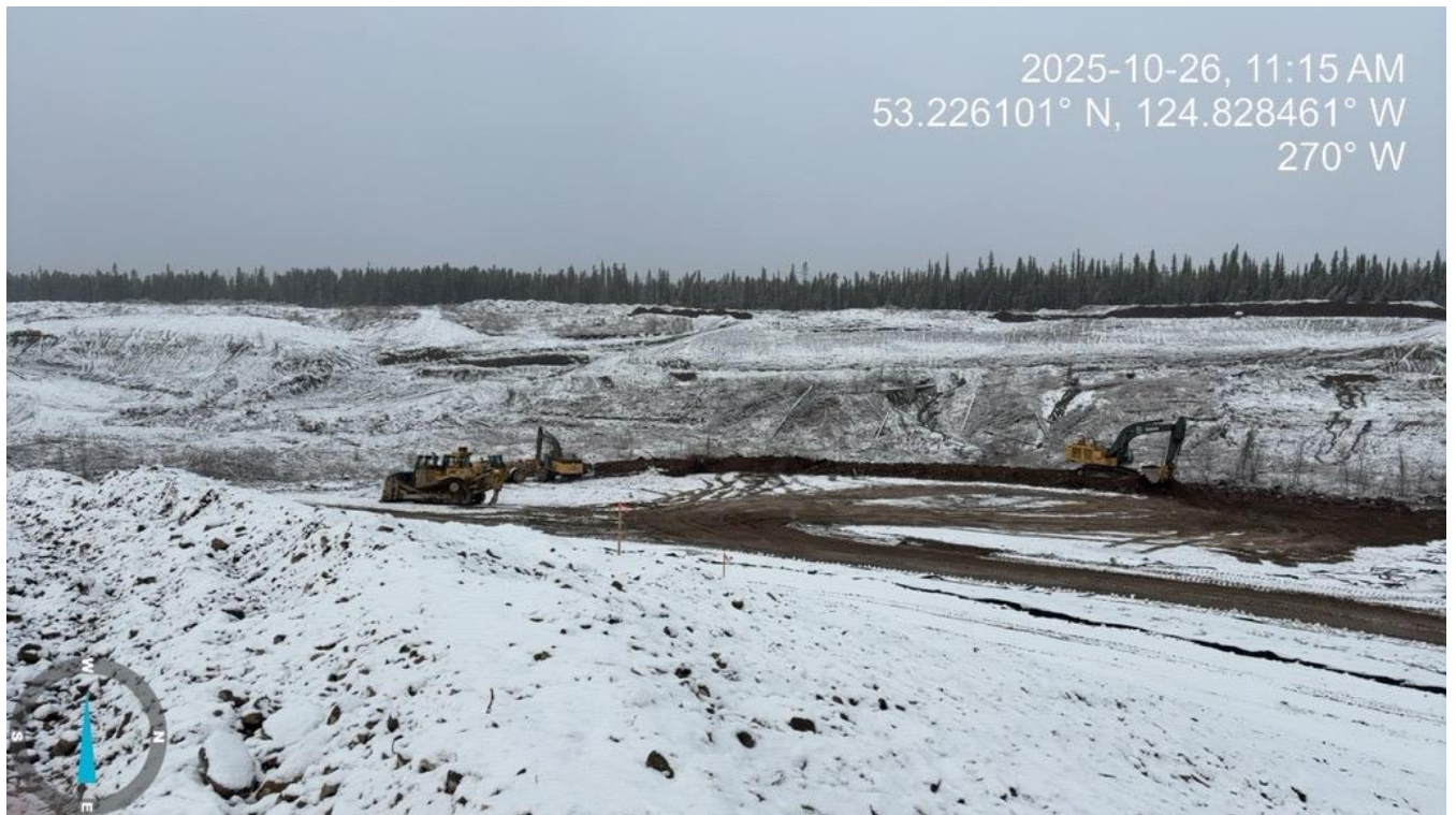
Photo 14: Excavator cleaning material to be hauled to the stockpile.
