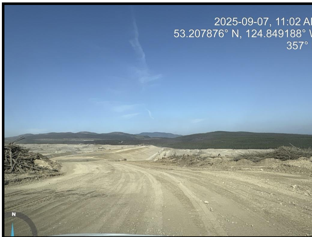
Photos 33 & 34: The Dam
