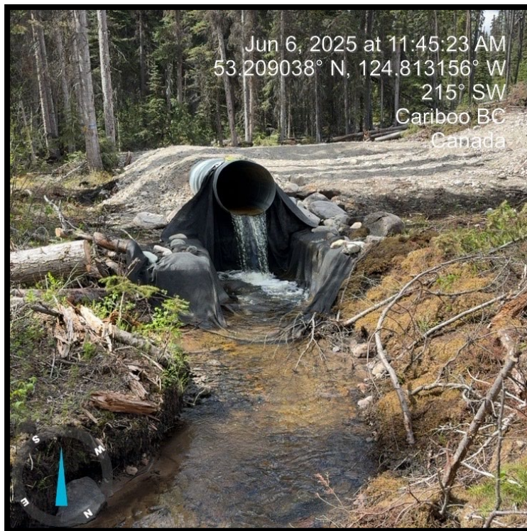
Photo 7: Creek 661-05 Drop Structure
