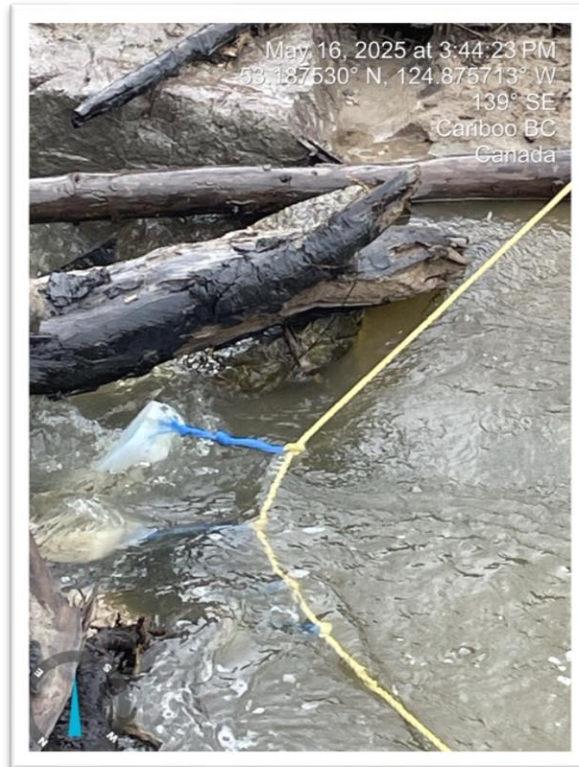
Photo 40: Installing Flocculant Blocks at Mine Creek
