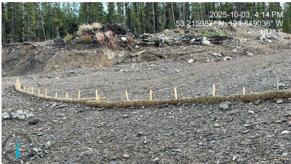
Photo 32, 33, & 34: Erosion and Sediment Control (ESC) Straw Waddle
