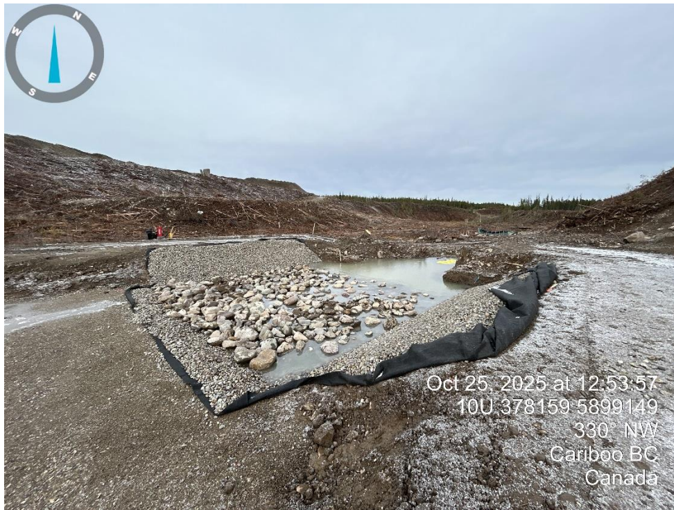
Photos 19 & 20: Fresh Water Reservoir
