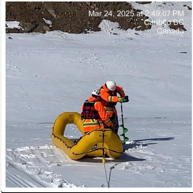
Photo 15: Drilling Holes at CWTP Pond
