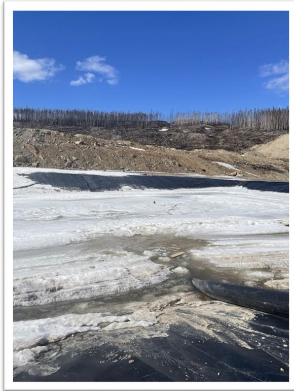
Photo 8: Central Water Transfer Pond
