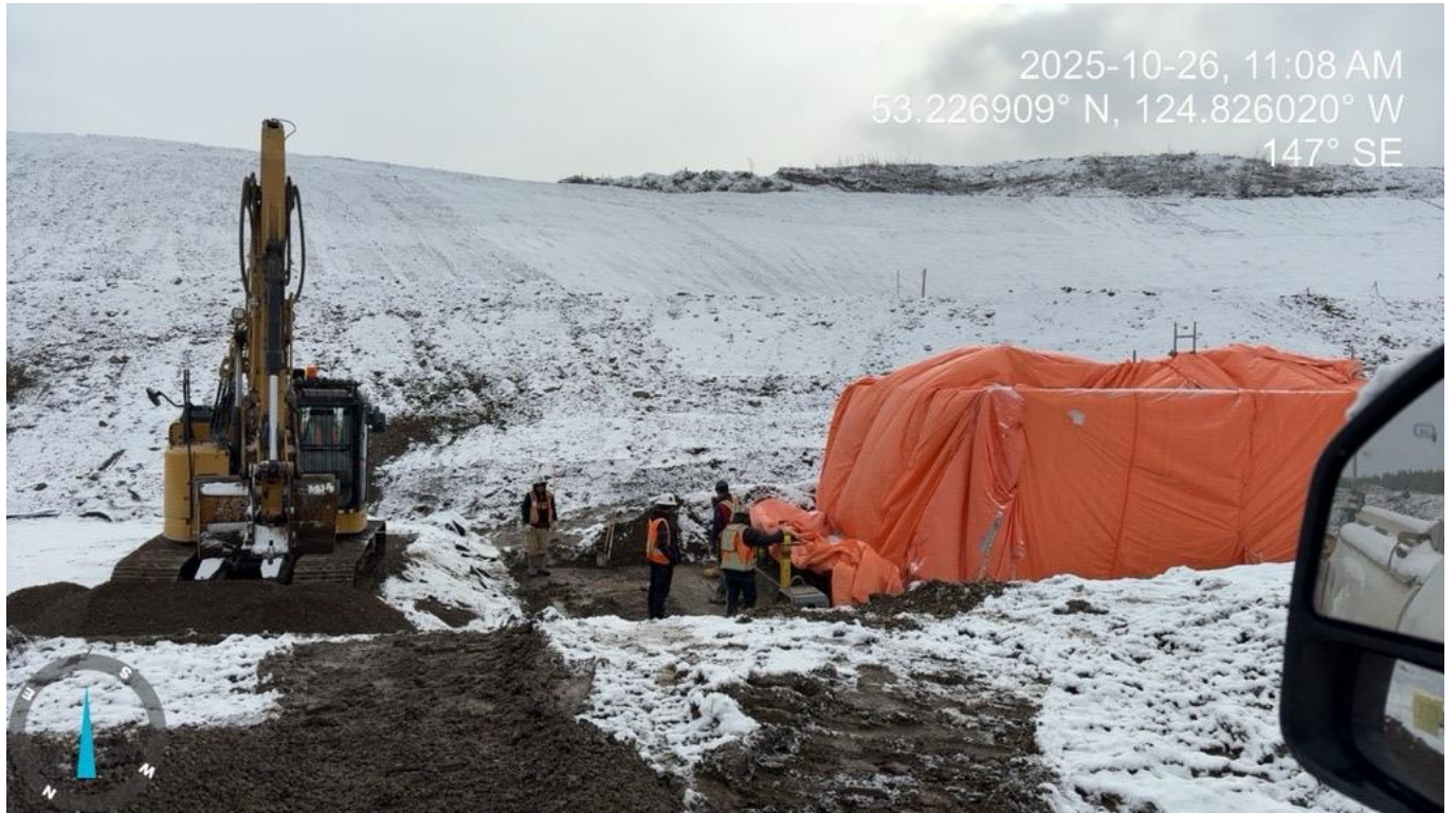
Photo 11: Concrete Flow Chamber Structure (FWR)
