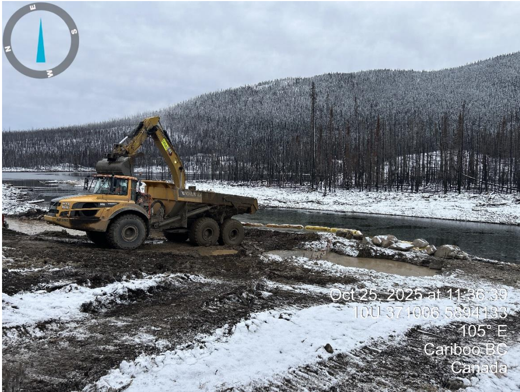
Photos 21 & 22: New channel at Lakes 15 & 16
