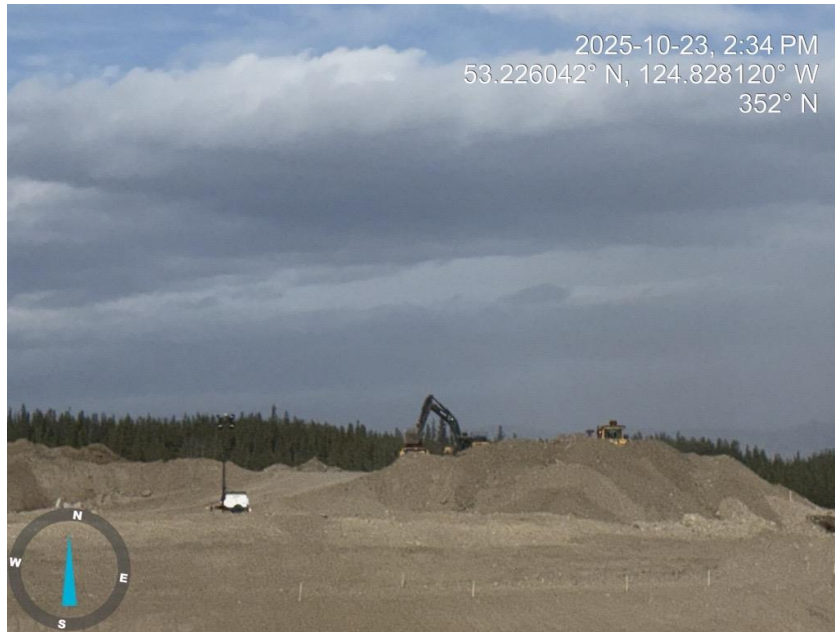
Photo 7: Hauling from the West side.
