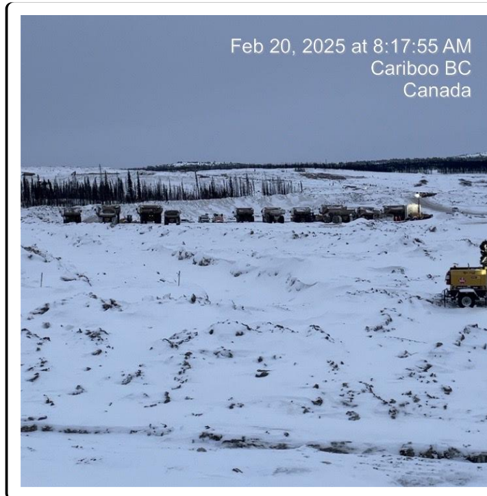
Photo 11: Low Grade Ore (LGO) Stockpile Pad
