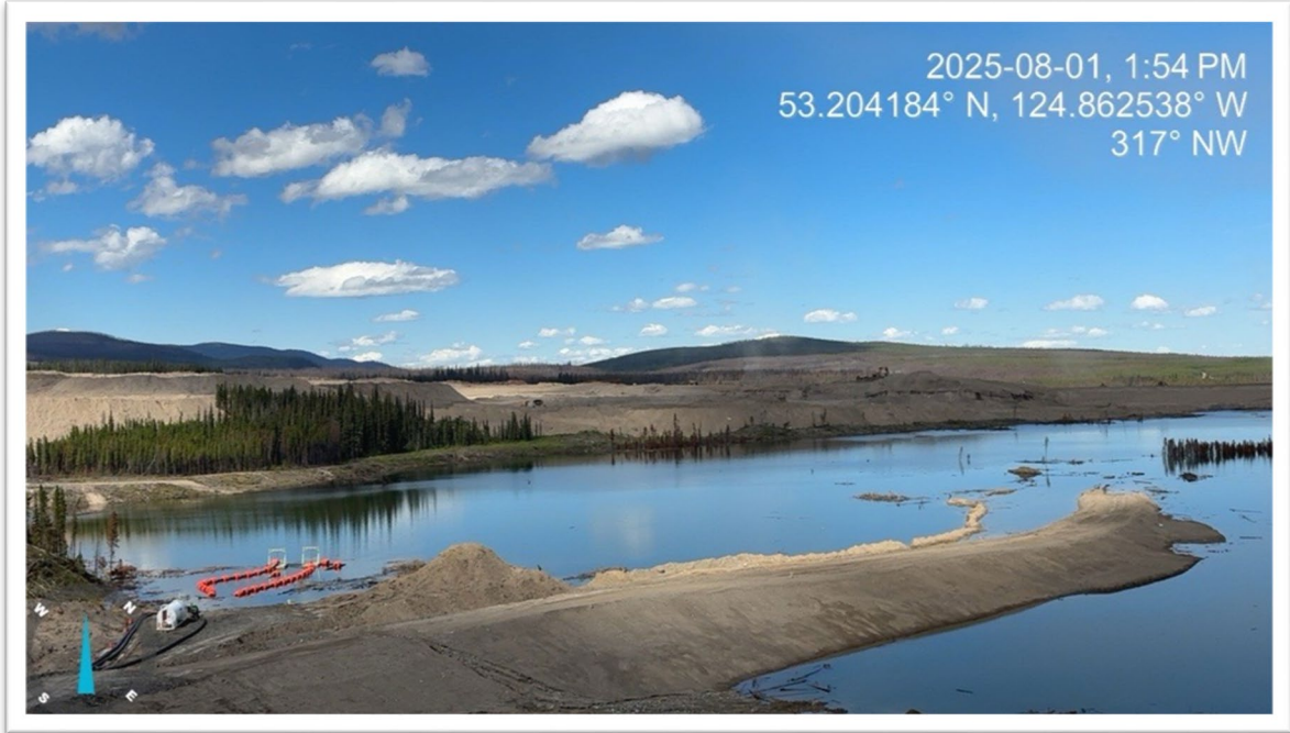
Photo 8: Tailing Storage Facility
