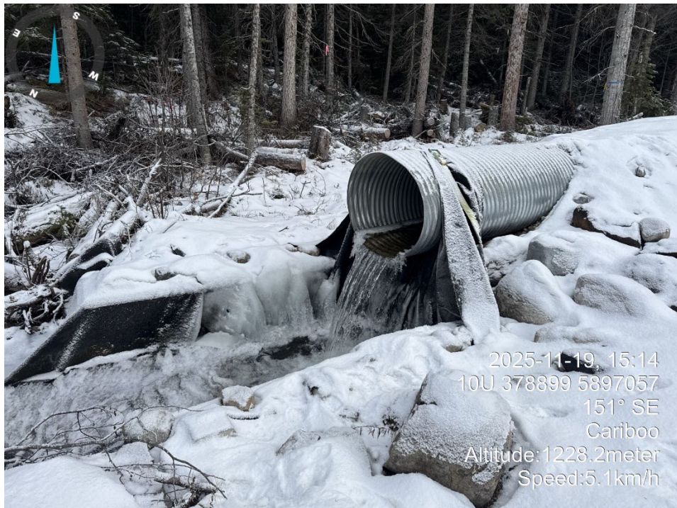
Drop structure inspection
