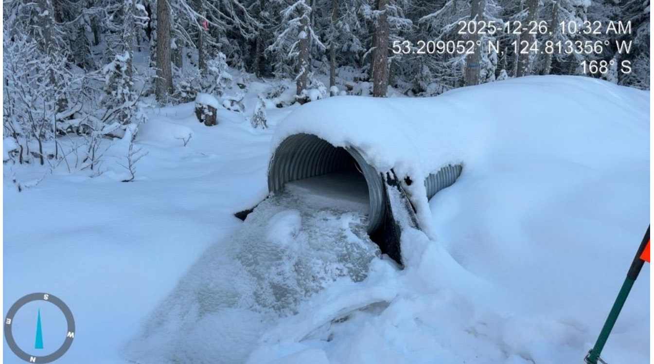
Photo 26: Drop Structure at Creek 505
