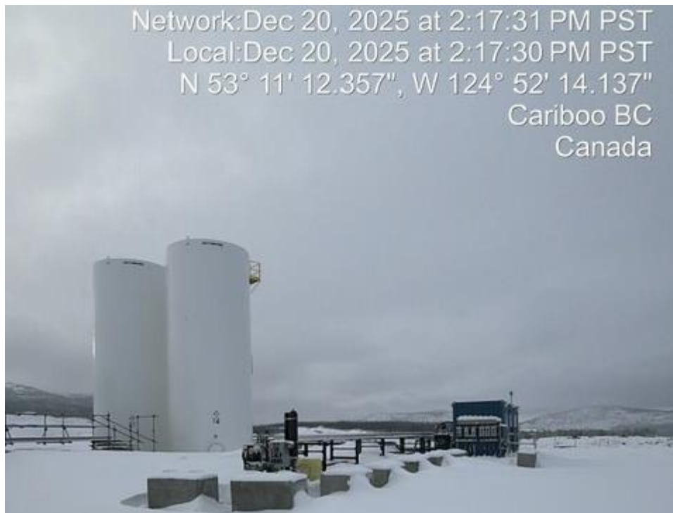
Photo 9: New Fuel Bay at 15.5 Km
