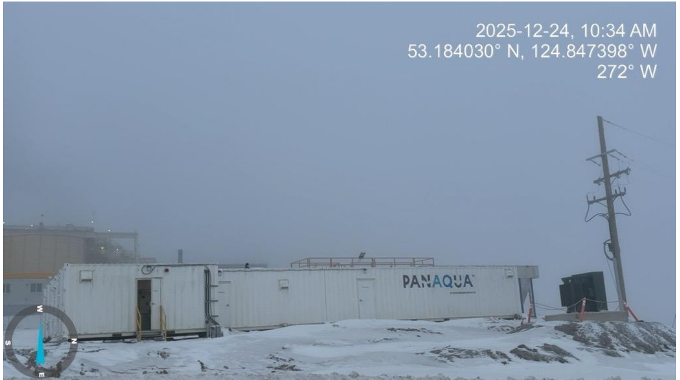
Photo 22: The Metals Treatment Plant
