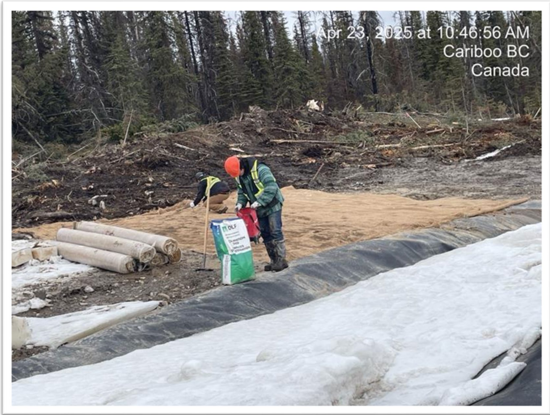
Photo 34: Installing Coco matting and Seeds
