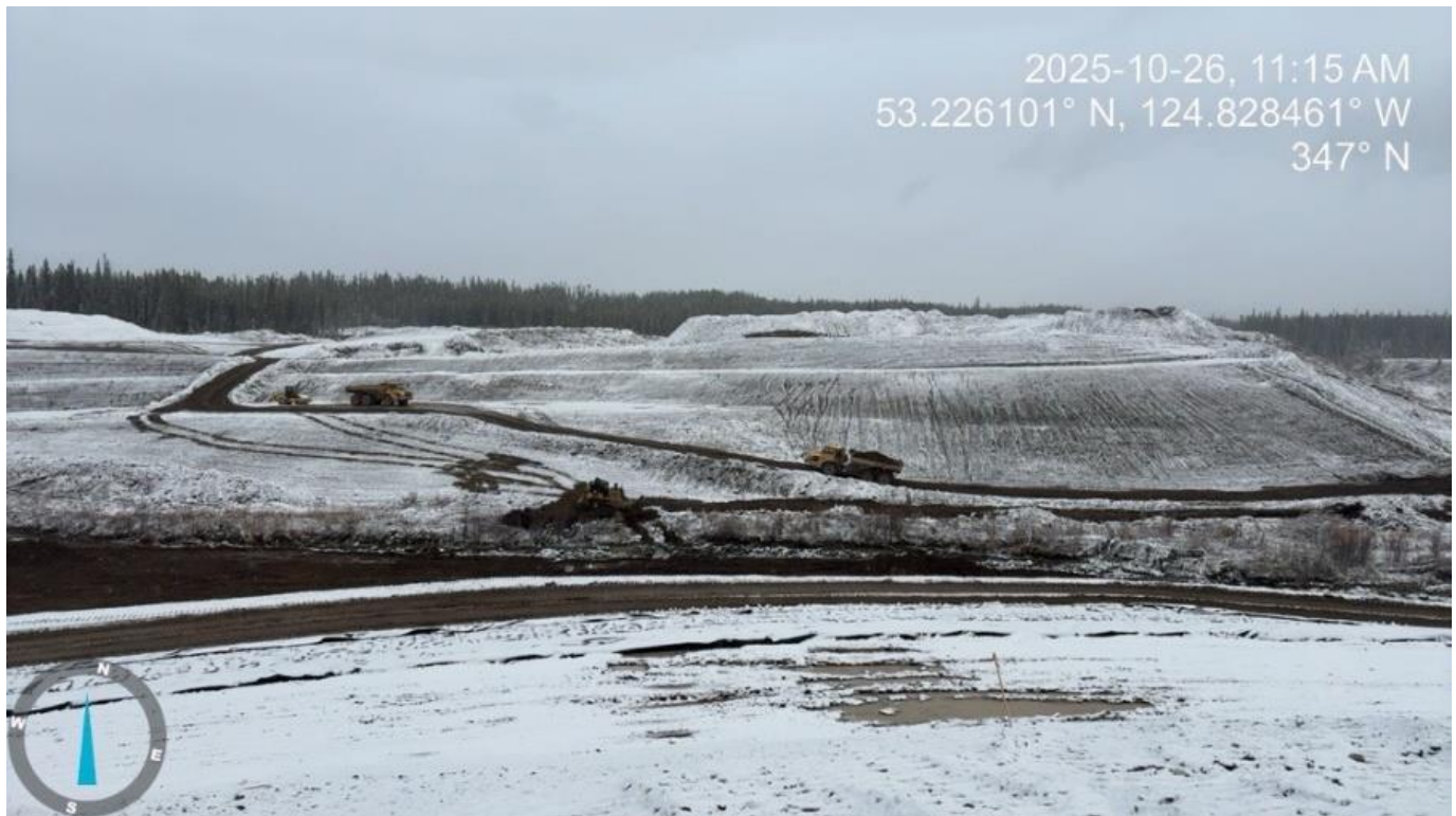
Photo 12: Trucks Hauling to shape the bottom.
