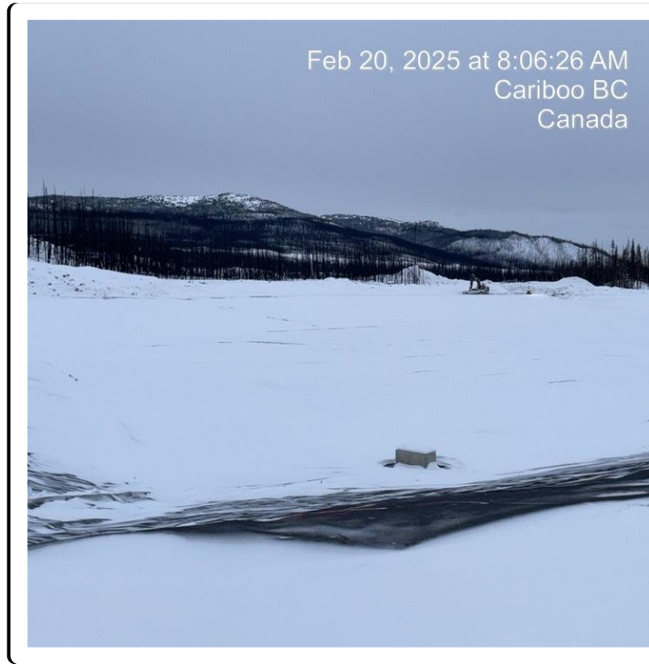
Photo 9: Low Grade Ore (LGO) Pond with HDPE Liner
