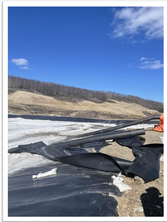
Photo 6: Central Water Transfer Pond
