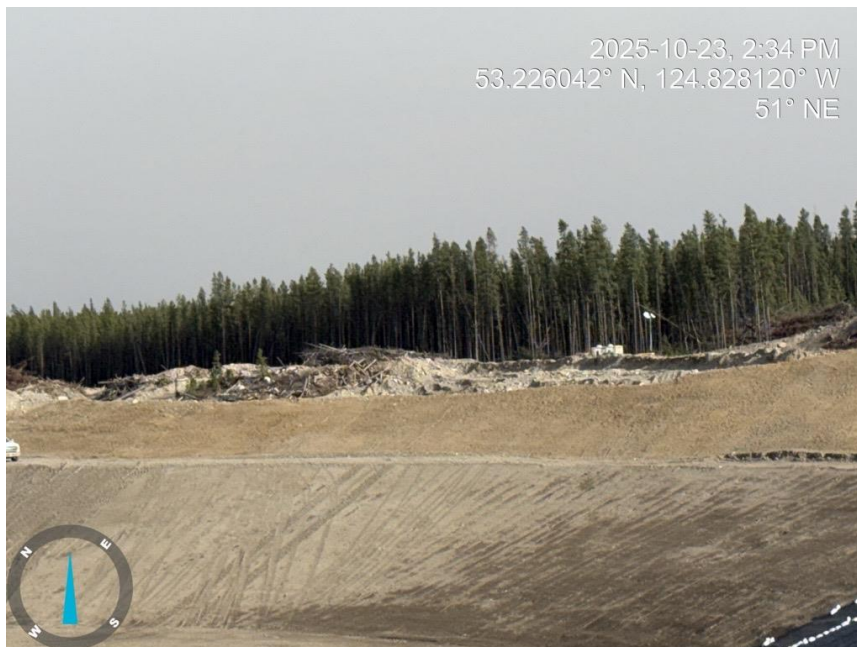
Photo 6: Shaping of Western Basin Slope
