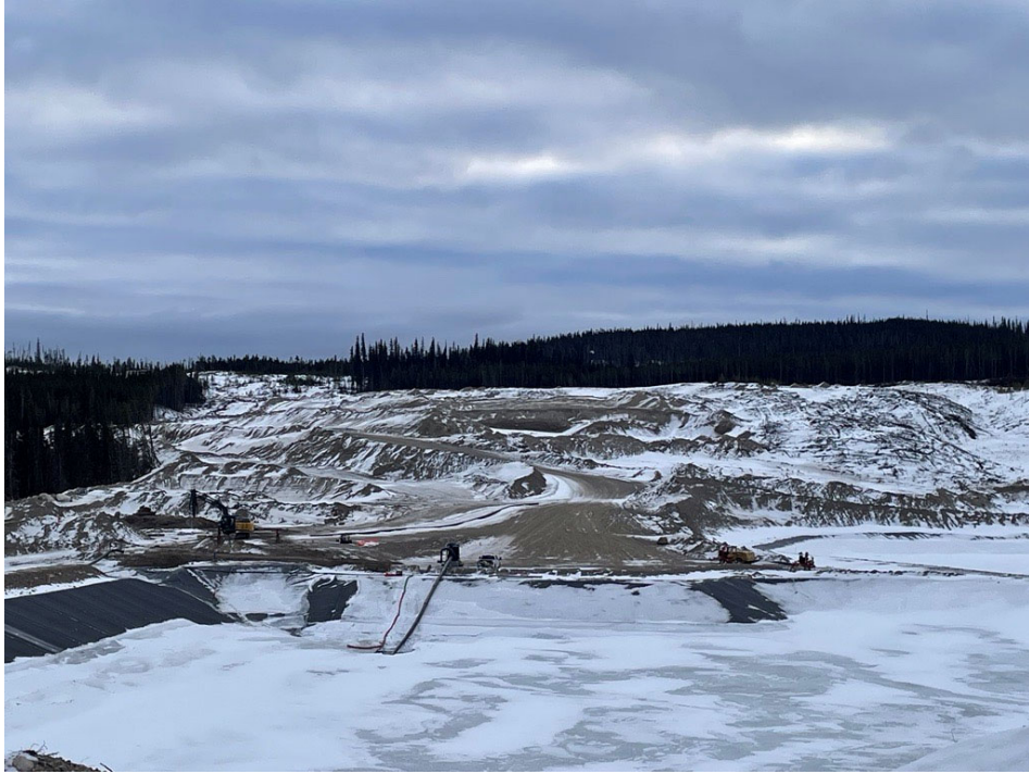
Photo 9: Interim Environmental Control Dam
