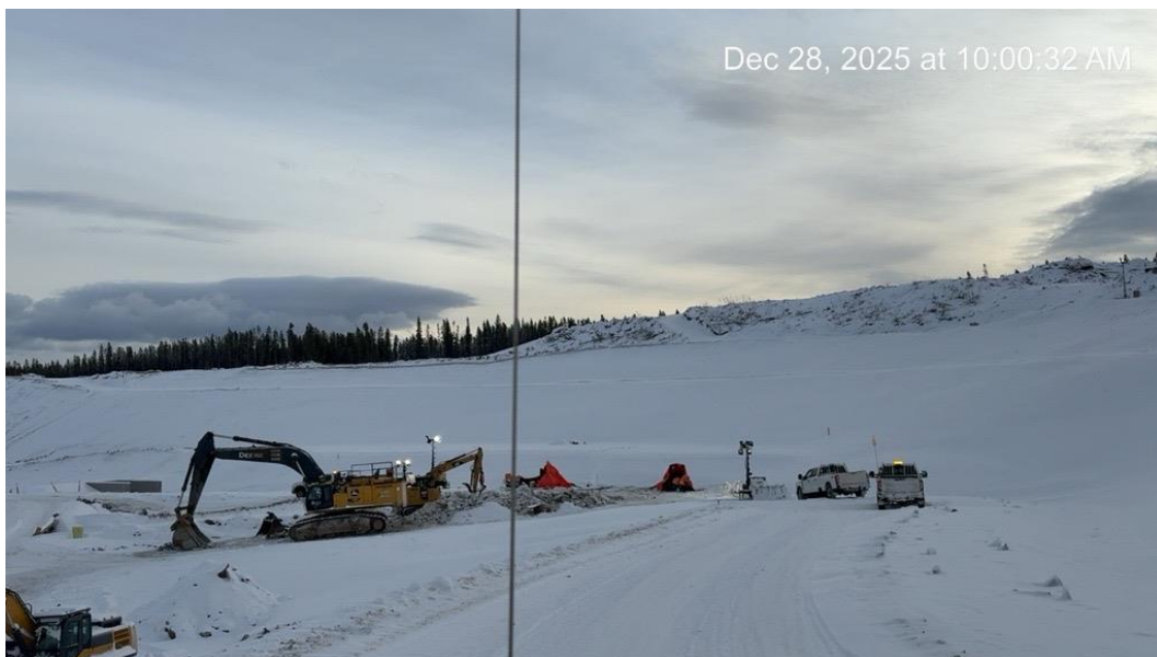
Photo 32: Crew working on the Diversion Channel.
