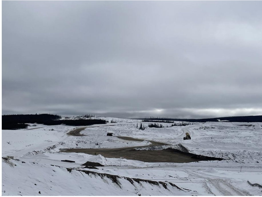
Photo 3: Potential Acid Generating (PAG) Dump at Tailings Storage Facility
