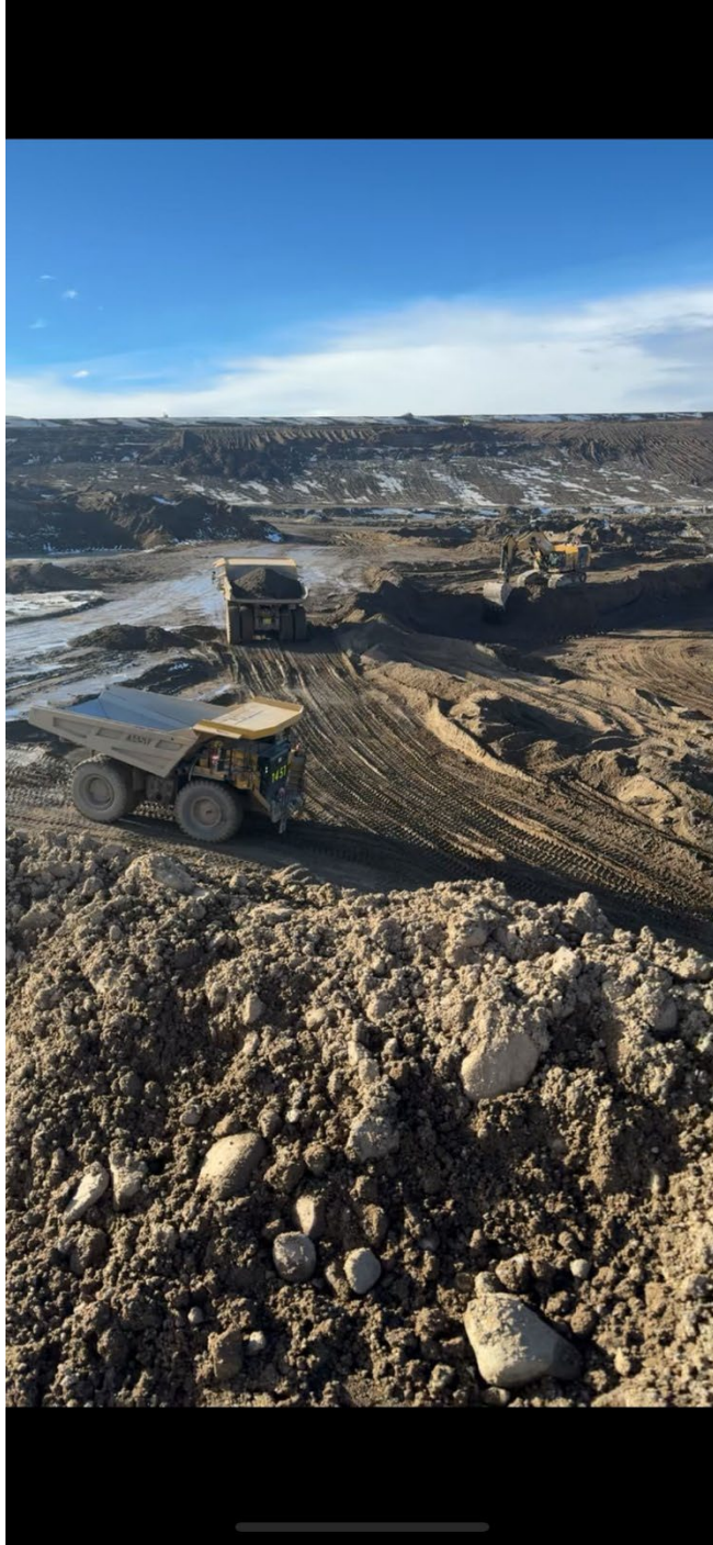
Earthworks activity on the tailings dam.
