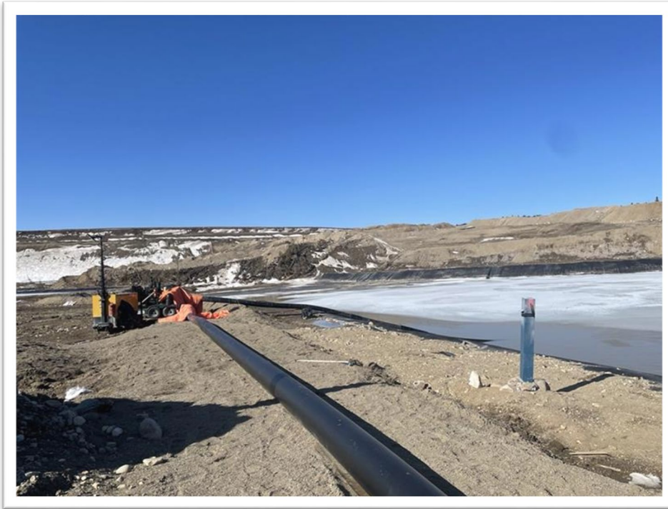
Photo 20: Interim Environmental Control Dam
