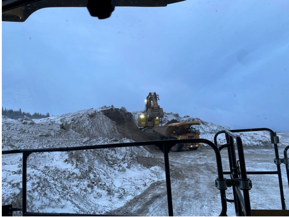
Photo 7: 790 Rock Truck Loading up With Ore
