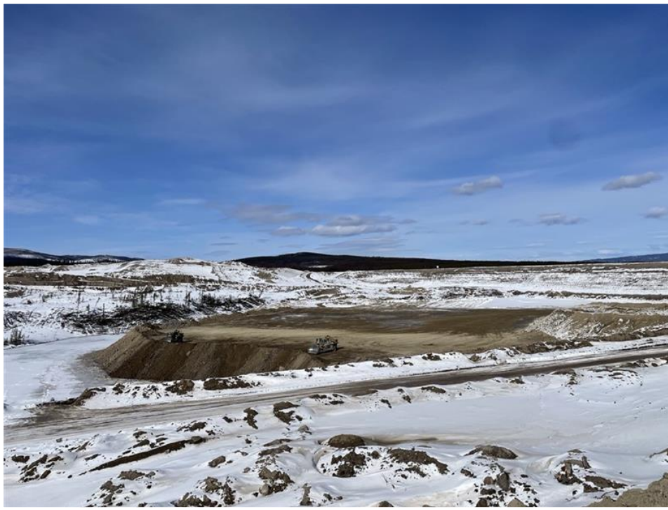
Photo 7: Potential Acid Generating (PAG) Dump at Tailings Storage Facility
