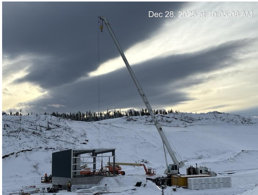
Photo 34: Construction of the Pump House
