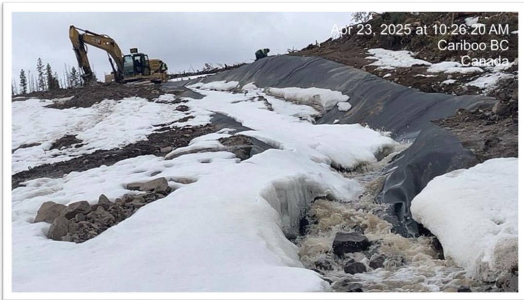
Photo 33: Northern Diversion Channel
