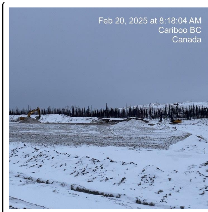
Photo 12: Low Grade Ore (LGO) Stockpile Pad
