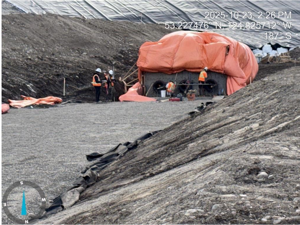
Photo 3: Concrete Flow Chamber Structure (FWR)
