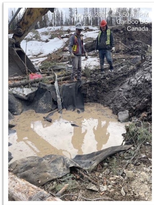
Photo 36: Installing Sump at Northern Diversion Channel
