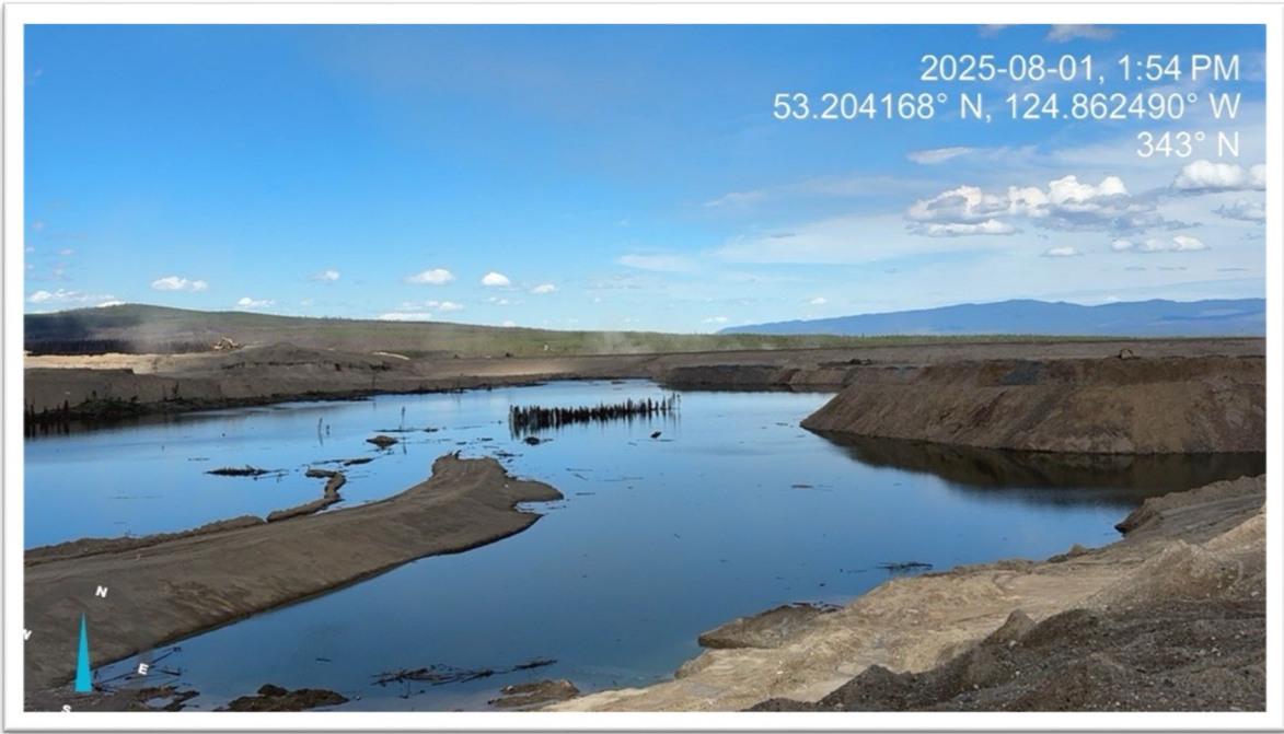
Photo 7: Tailing Storage Facility
