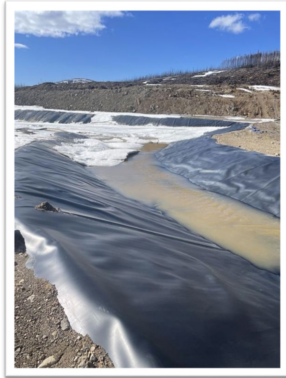
Photo 10: Central Water Transfer Pond Overflow
