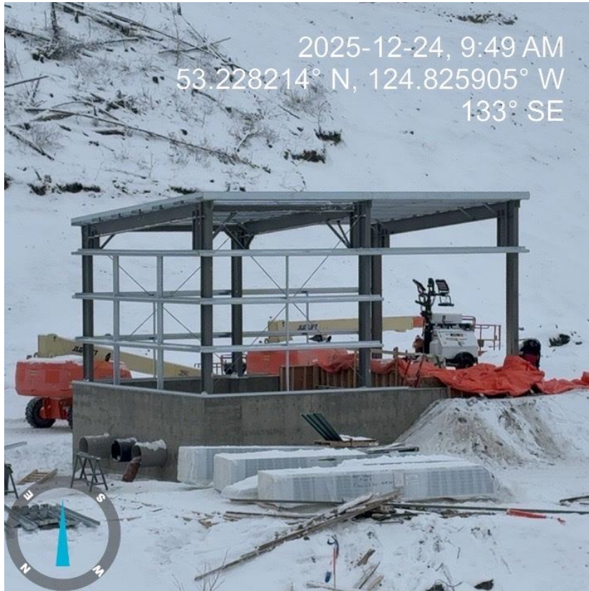
Photo 33: Construction of the Pump House
