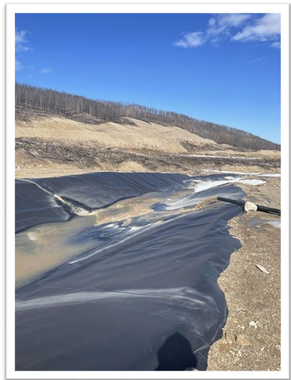
Photo 9: CWTP Overflow with North/South Collection Channel diversion pumps into TSF
