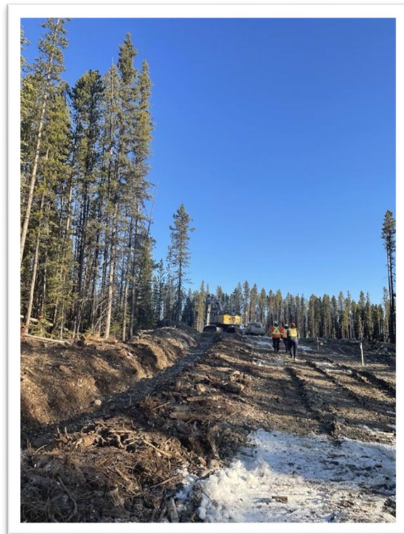
Photo 11: Trench to Divert Runoff
