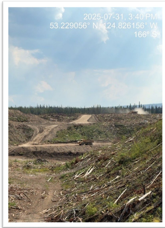
Photo 1: Davidson Creek Fresh Water Reservoir
