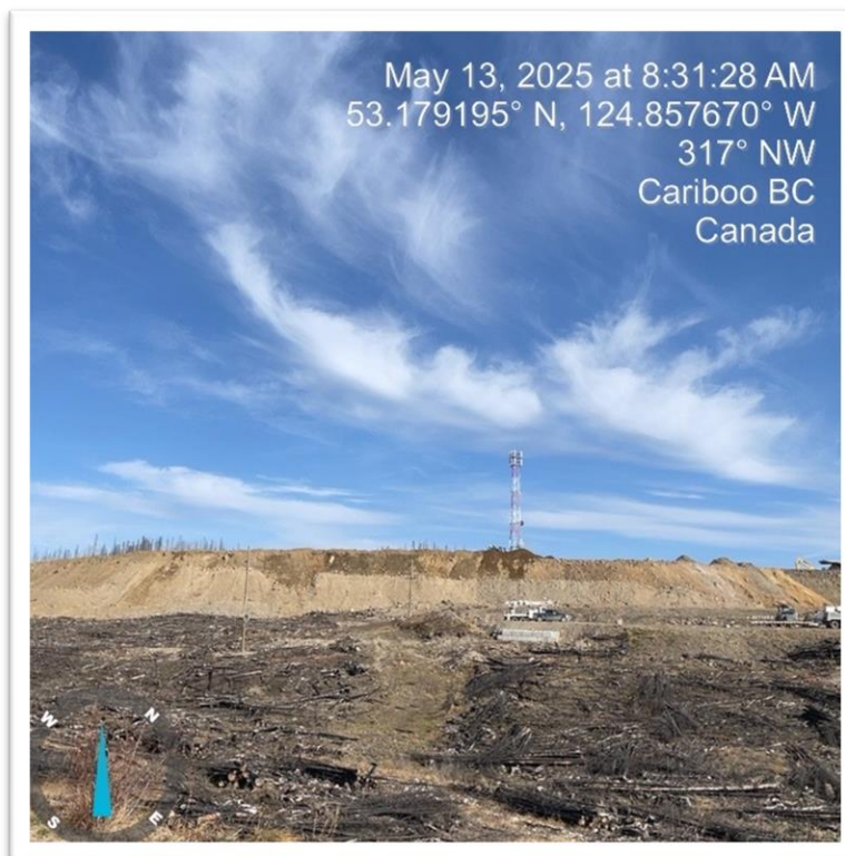
Photo 29: Extending Run of Mine (ROM) Pad
