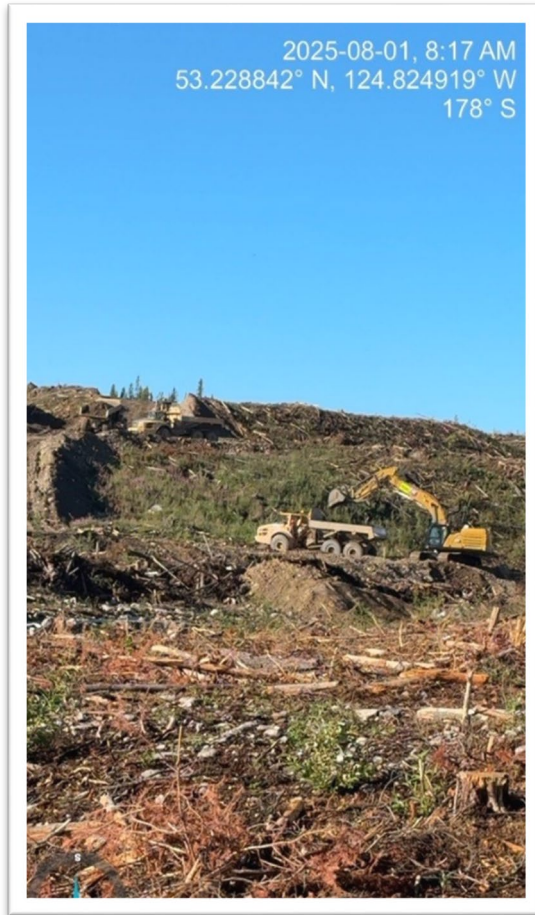
Photo 5: Davidson Creek Fresh Water Reservoir
