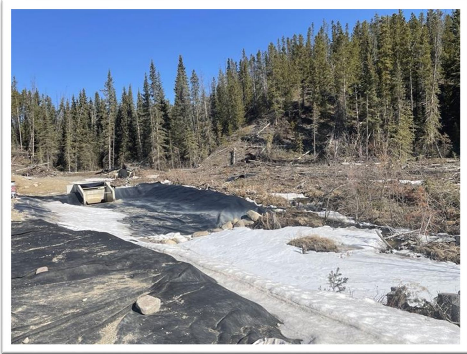
Photo 22: Old Davidson Creek Diversion System Impact Spillway Near Creek 668
