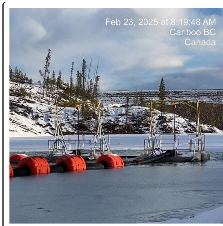
Photo 18: Tailings Storage Facility – Reclaim Barge
