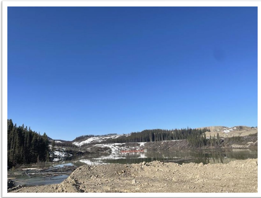
Photo 17: TSF Reclaim Barge Intake
