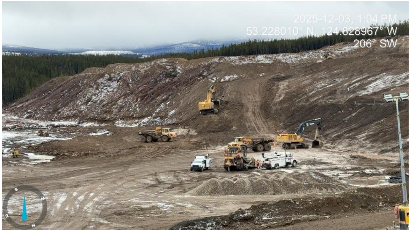
Photo 5: Fresh Water Reservoir
