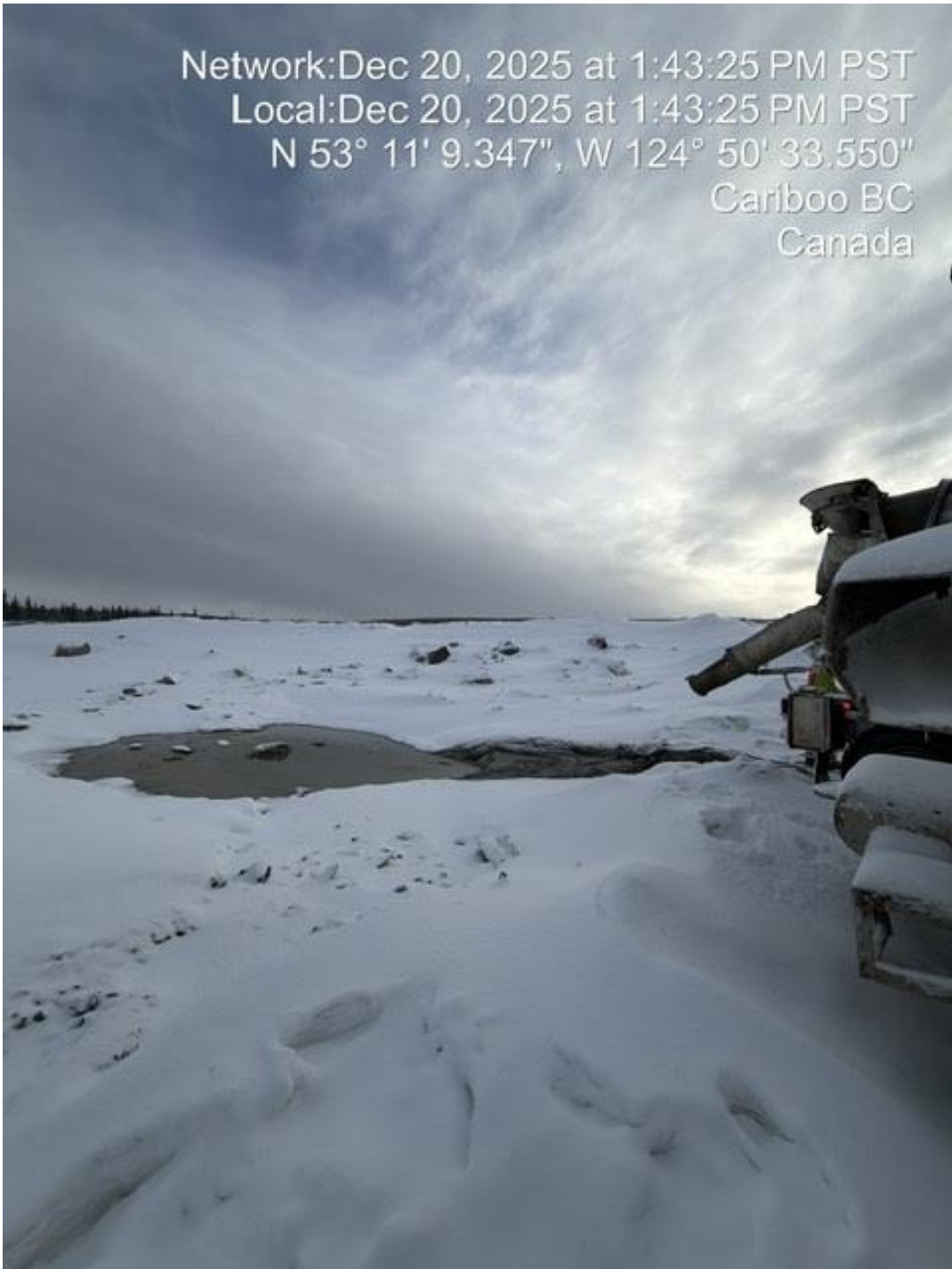
Photo 28: CIF cement waste was disposed of in a lined sump with a protective berm, confirmed for compliance. The material will be transferred to the tailings facility once the sump reaches capacity.
