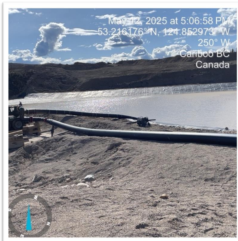
Photos 24 & 25: Interim Environmental Control Dam and pump back to TSF
