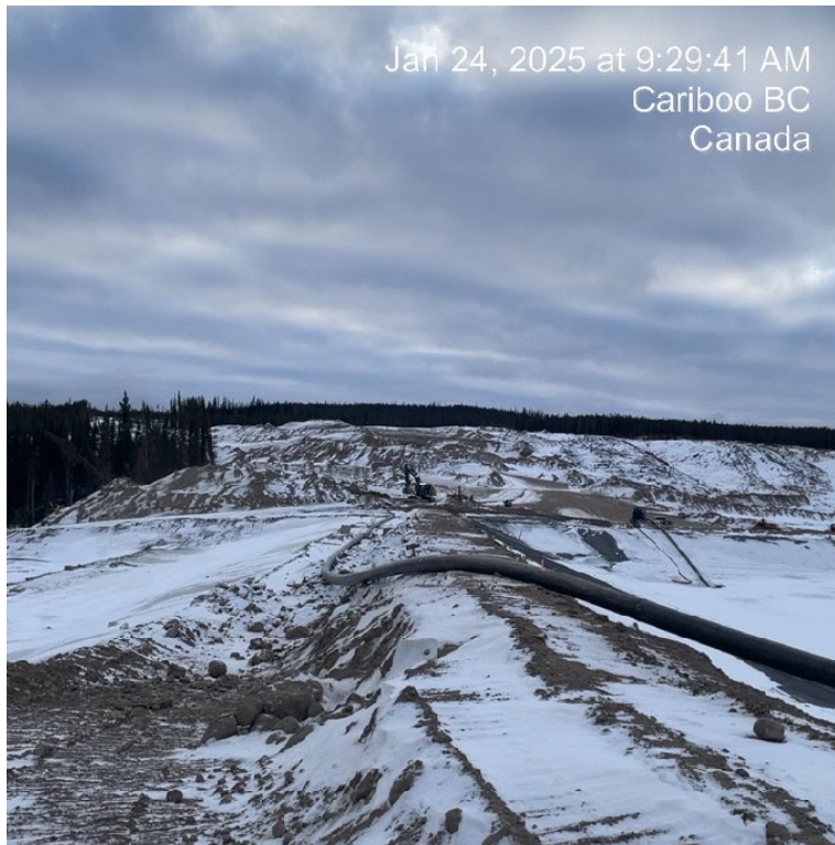
Photo 10: Interim Environmental Control Dam
