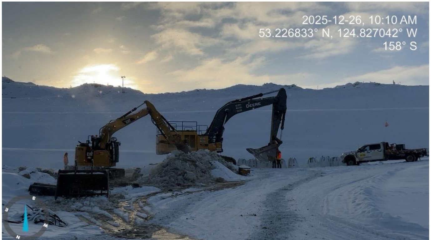
Photo 25: Two excavators clearing ice from the diversion channel
