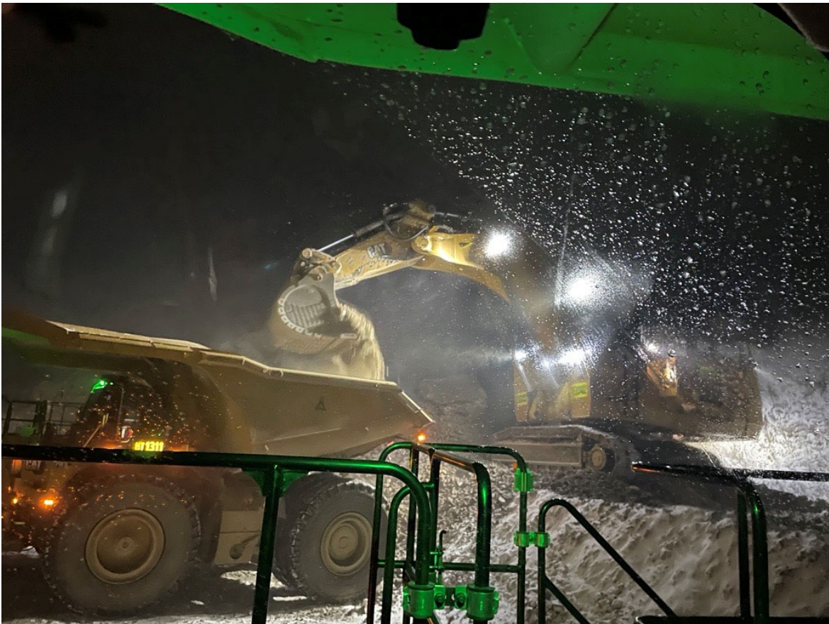
Photo 6: 790 Rock Truck Loading up With Ore
