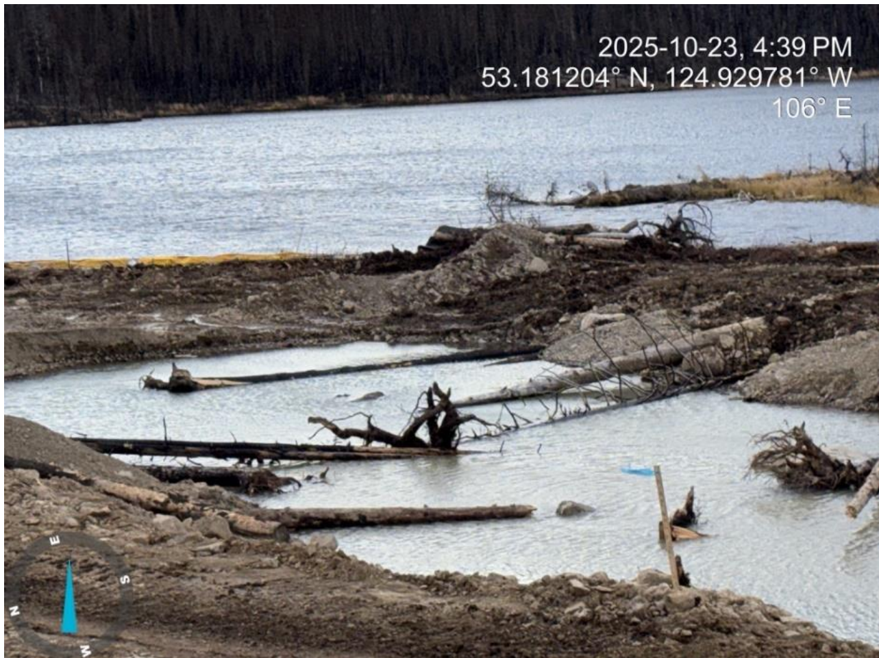
Photo 8: New channel at Lakes 15 & 16.
