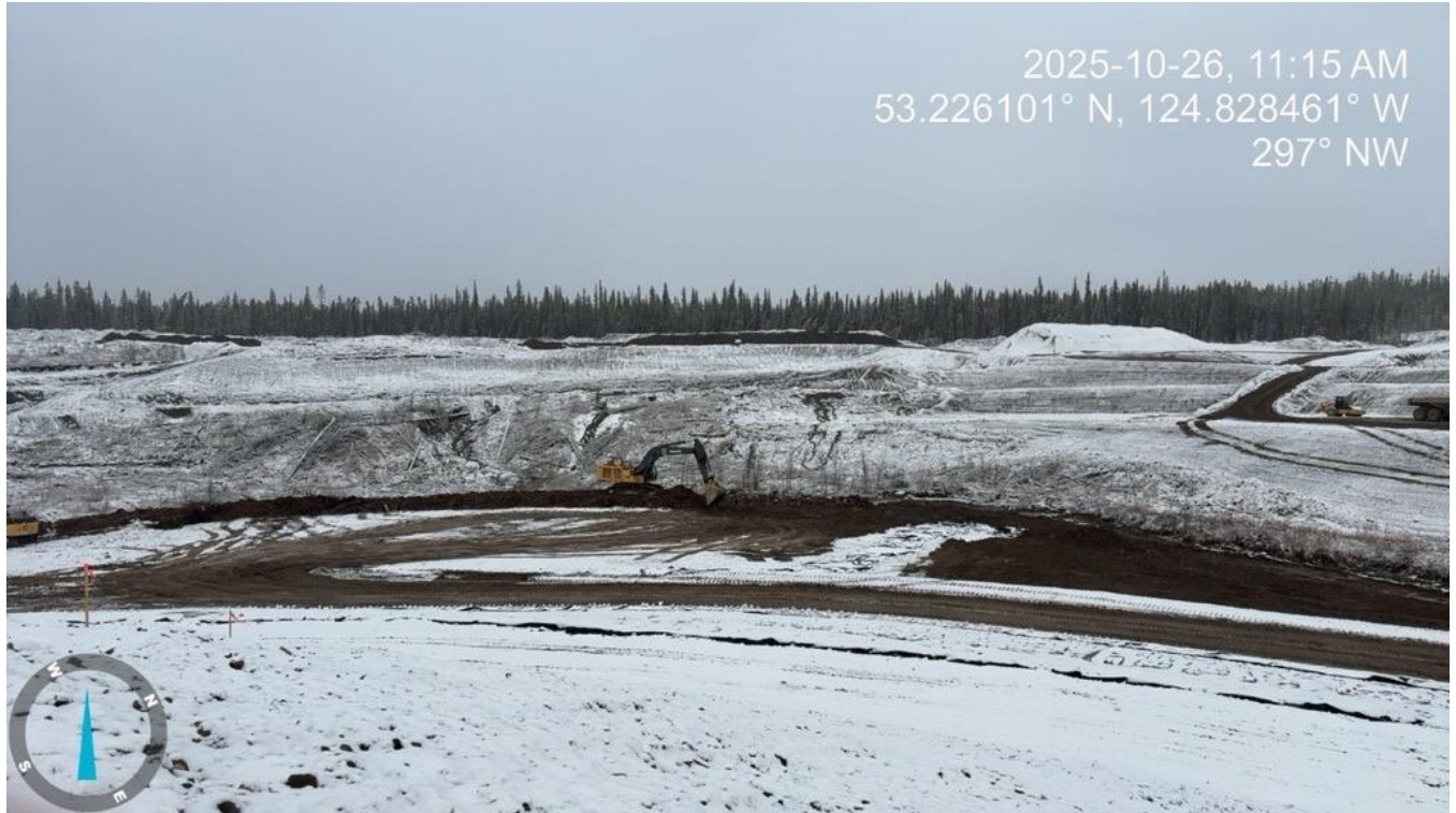
Photo 13: Excavator digging up material to haul away.
