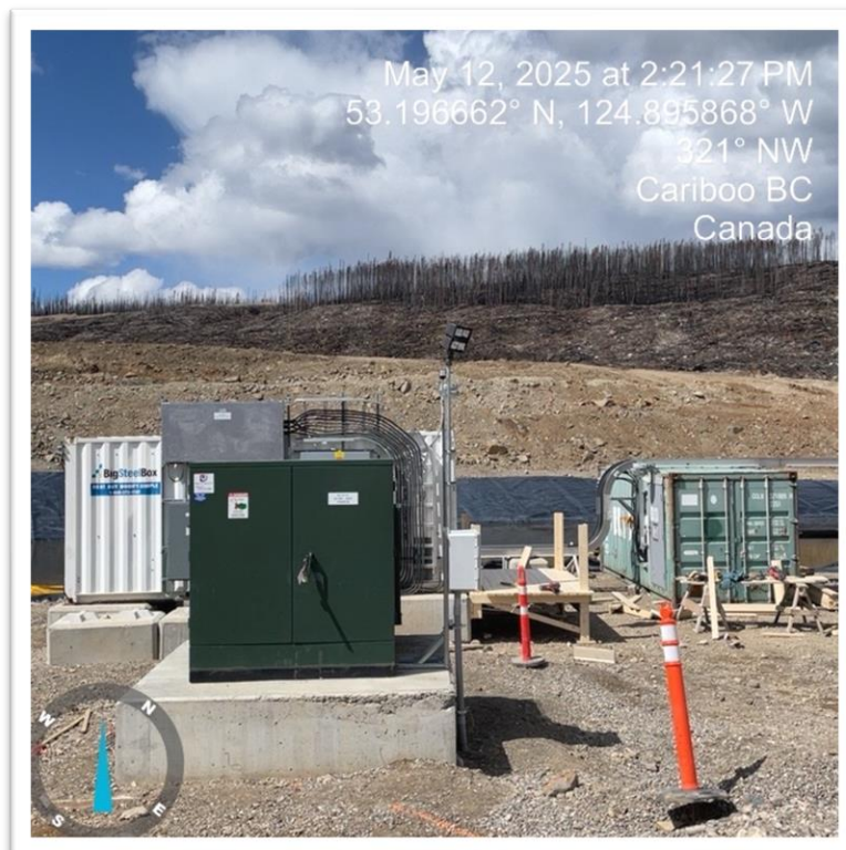
Photo 15 & 16: Permanent Electrical Pump Pad Central Water Transfer Pond
