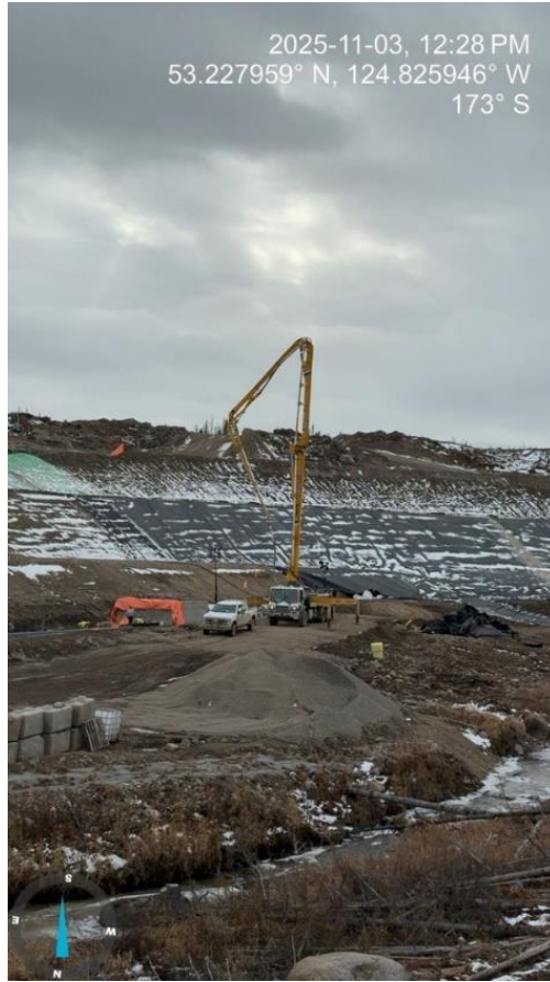
Photo 42: Pouring Concrete for the Flow Chamber
