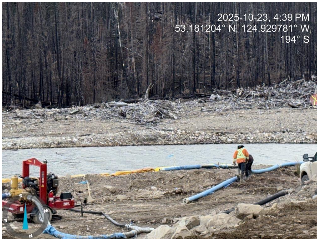
Photo 9 & 10: New channel at Lakes 15 & 16
