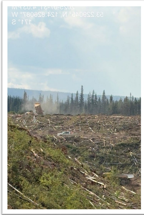
Photo 3: Davidson Creek Fresh Water Reservoir
