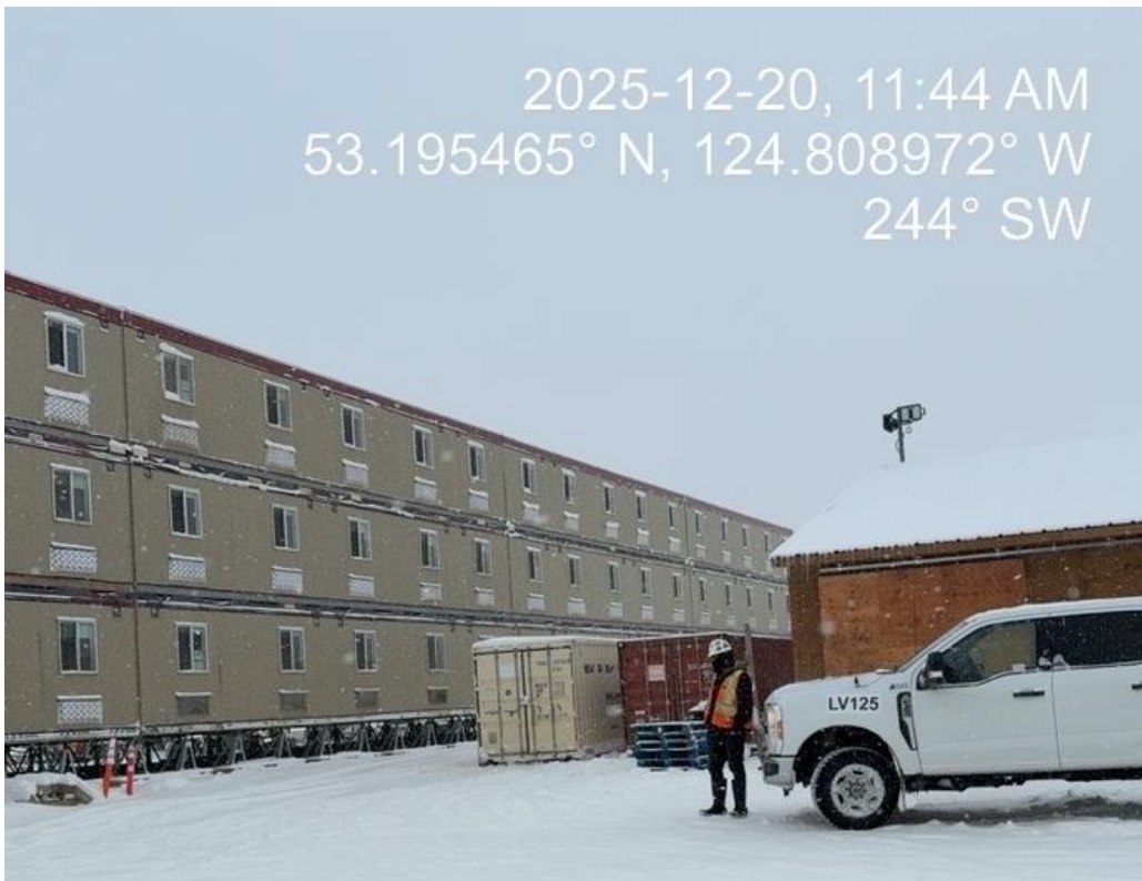
Photos 4 & 5: New Dorms Being Constructed
