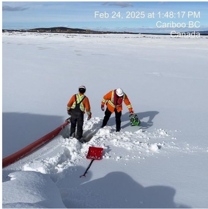
Photo 21: Drilling Holes at WMP Pond
