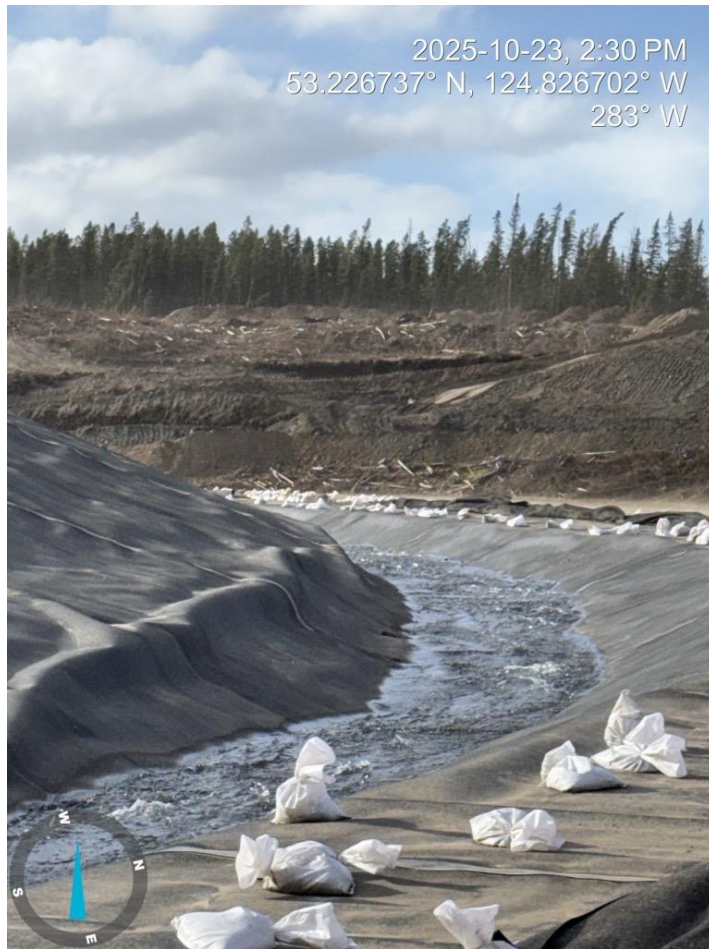
Photo 5: Diversion channel for Davidson Creek
