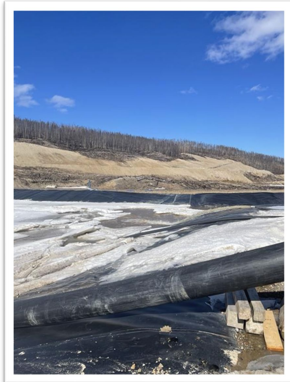
Photo 7: Central Water Transfer Pond
