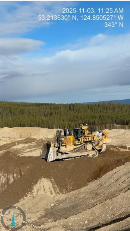
Photo 41: Dozer Pushing Material
