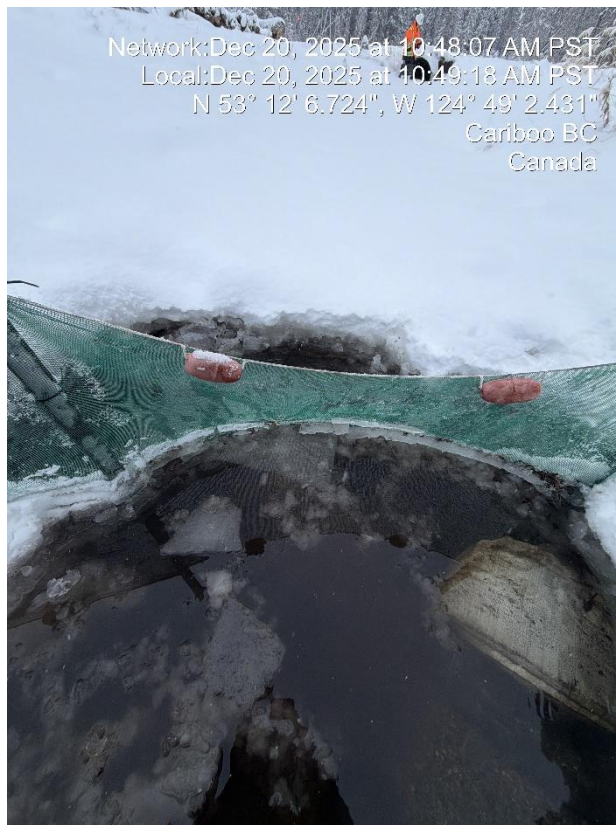
Photo 20 & 21: Creek 146 Fish Fence
