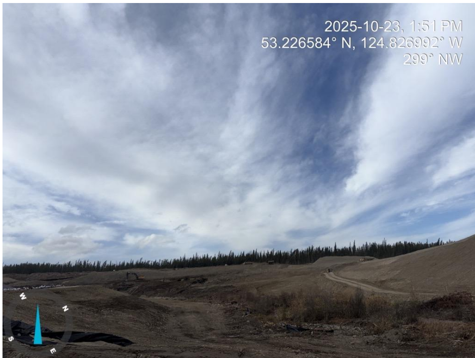
Photos 1 & 2: Fresh Water Reservoir (FWR)
