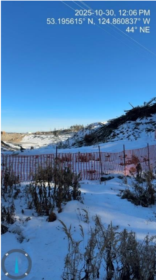
Photos 29 & 30: Wildlife Fence at WMP
