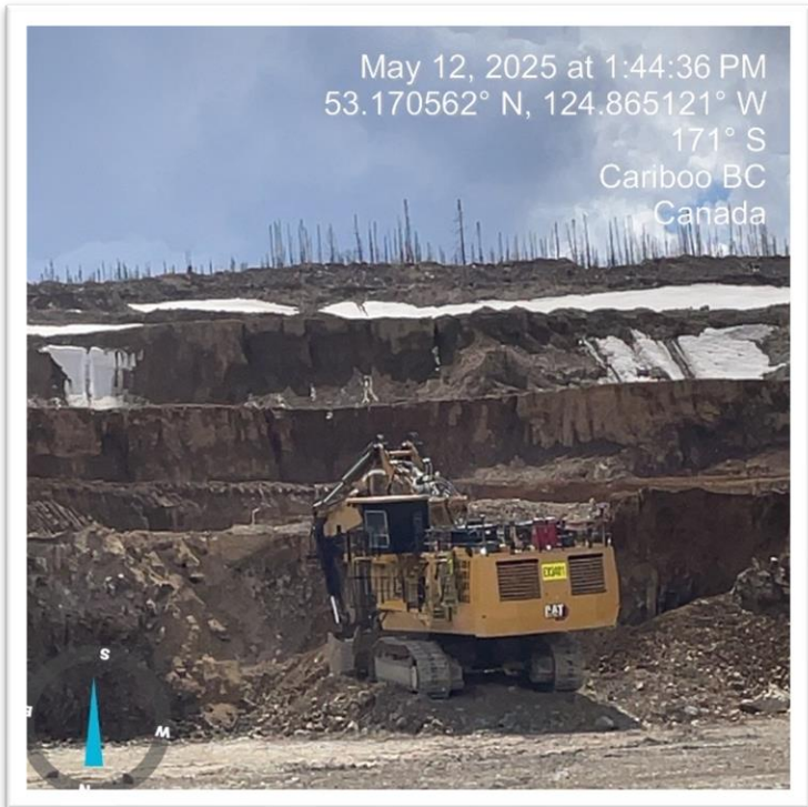
Photo 7 & 8: Excavator in the Pit
