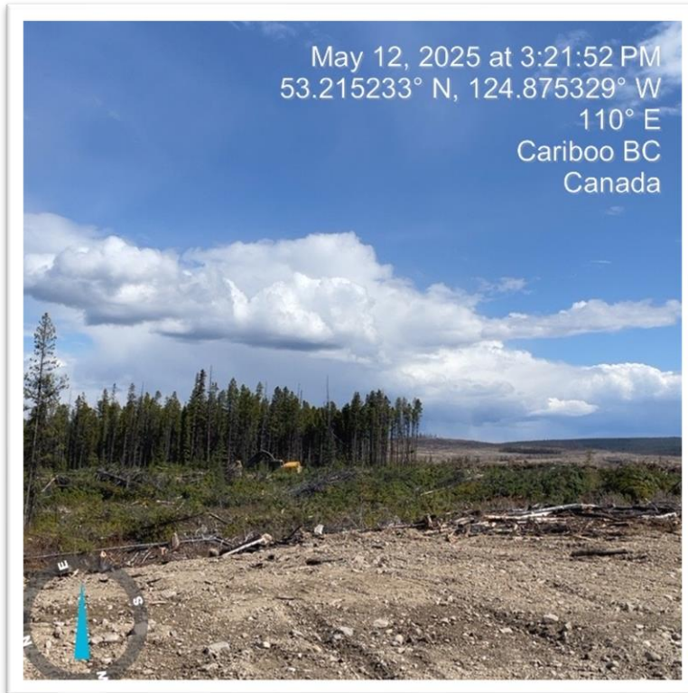
Photo 17: Clearing Tailings Storage Facility East Expansion
