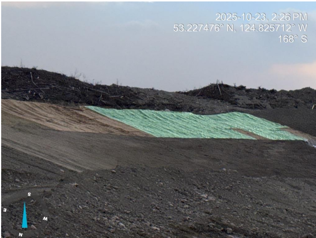
Photo 4: Laying coco mats for Erosion Sediment Control
