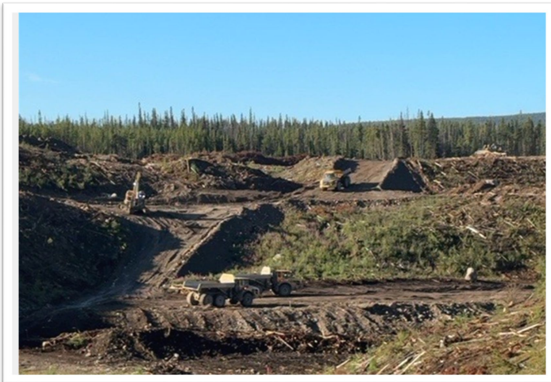
Photo 4: Davidson Creek Fresh Water Reservoir
