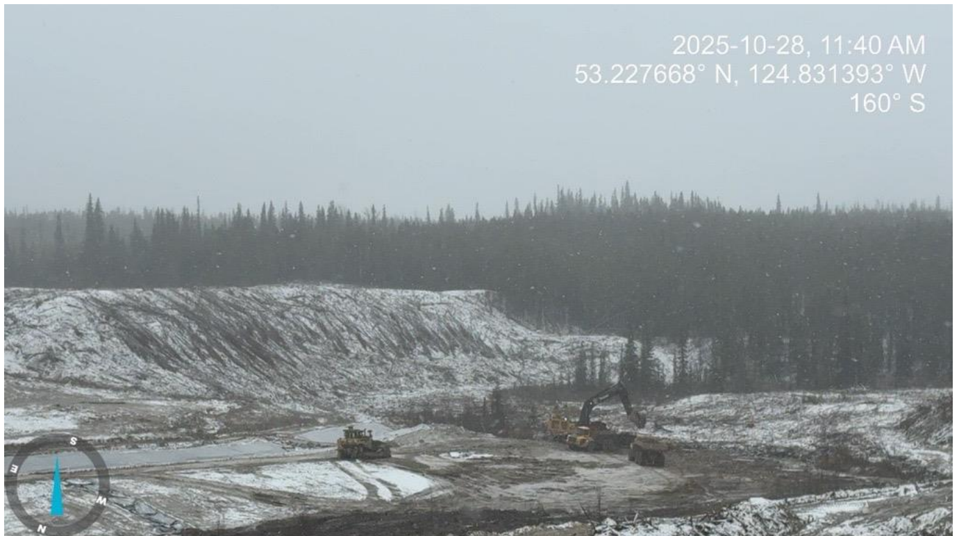
Photos 17 & 18: Fresh Water Reservoir
