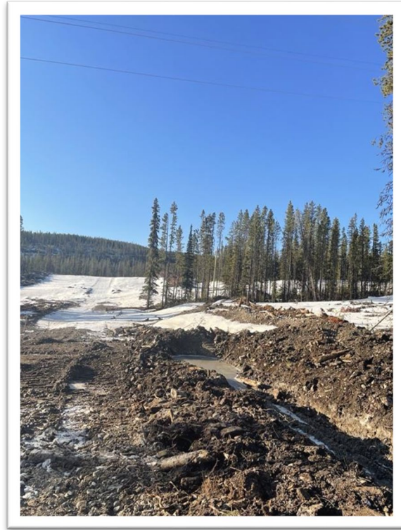
Photo 12: Trench to Divert Runoff
