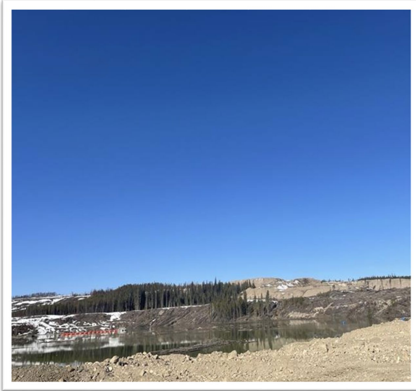
Photo 18: TSF Reclaim Barge Intake
