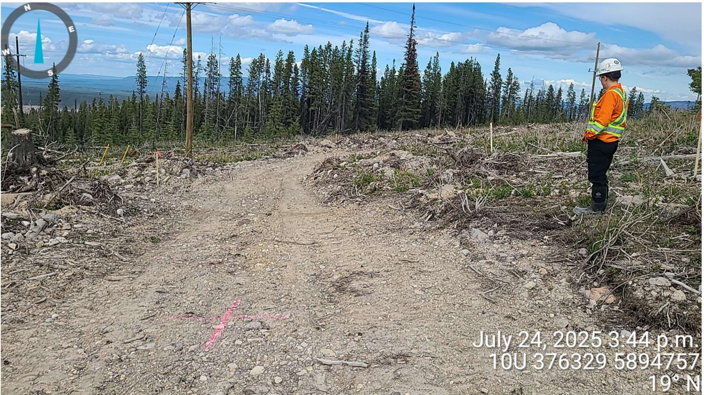
Photo 1. Overview of the stripping limit stakes.
