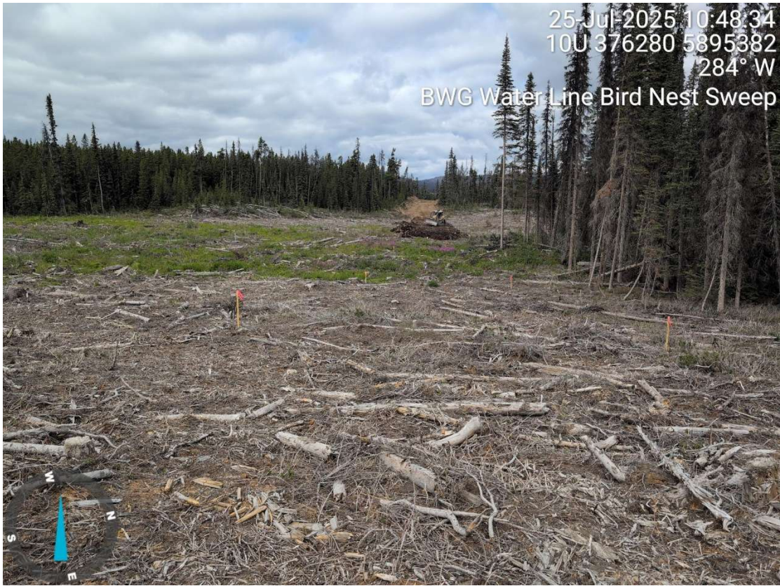
Photo 2. End of survey area where bulldozer had begun works.
