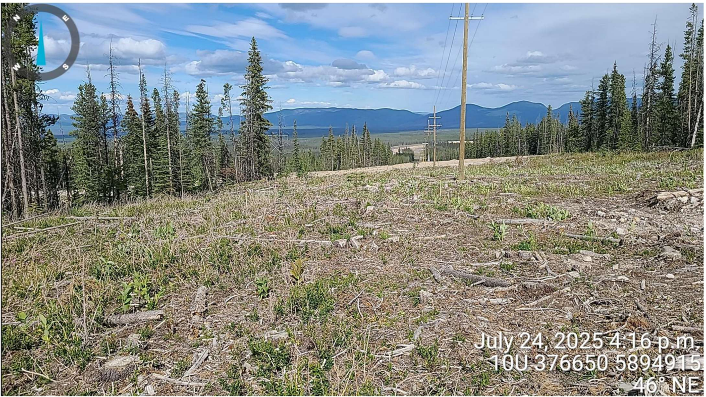
Photo 3. Overview of the stripping limit area, with minimal vegetation.
