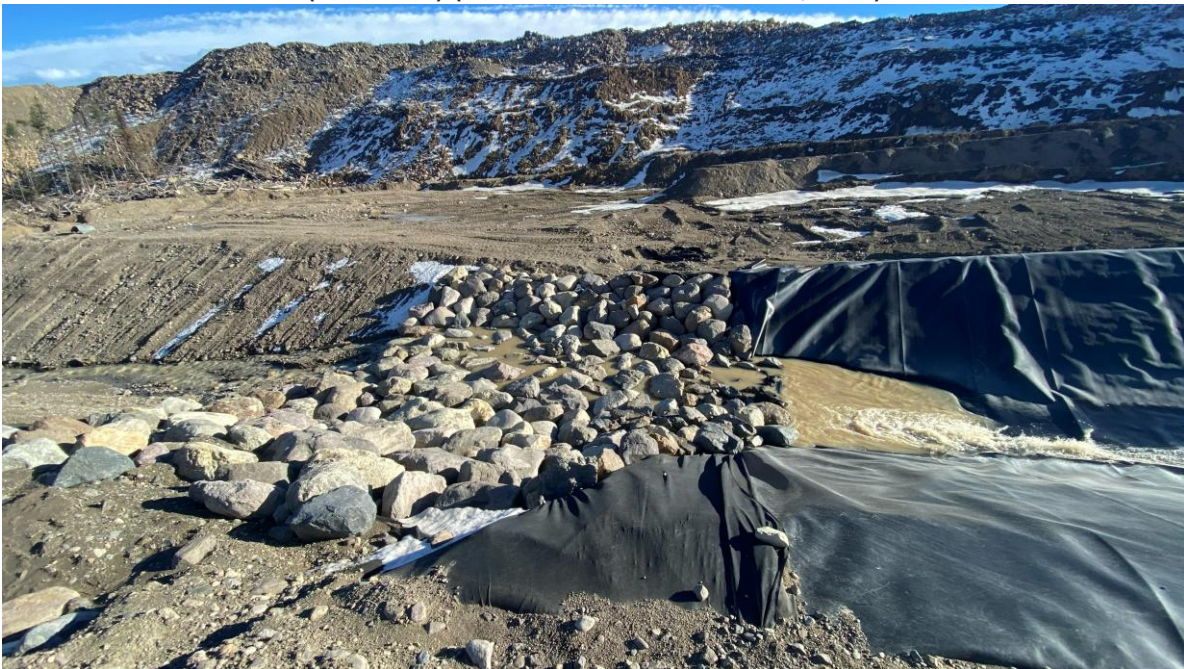
PHOTO 8 – Spillway outlet riprap apron, looking east (Photo taken on October 31, 2025)
