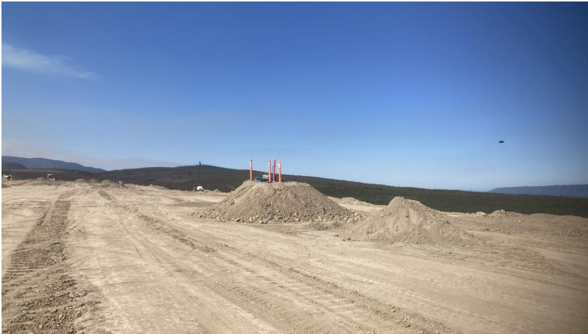
PHOTO 37 – MDC-S1E-PZ3 inclinometer and VWPs (Photo taken on September 16, 2025)
