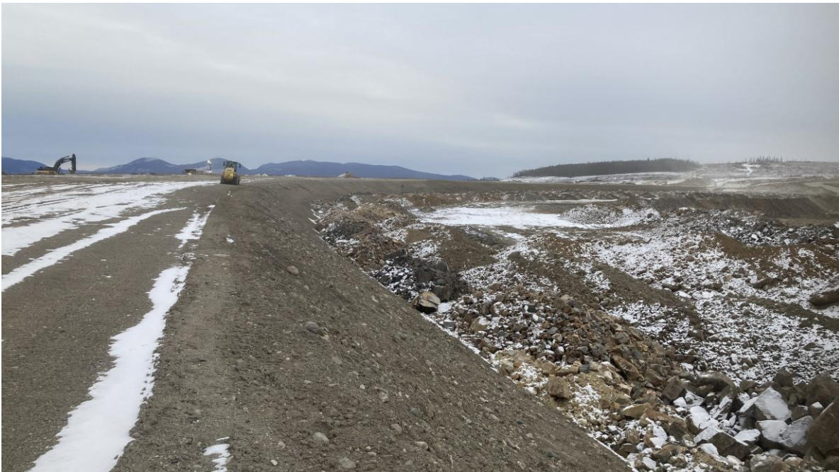
PHOTO 10 – MDC crest and upstream face and PAG waste rock dump, looking east (Photo taken on November 28, 2025)
