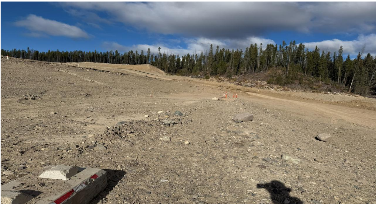
PHOTO 12 – IECD downstream bench, looking northwest (Photo taken on October 12, 2025)
