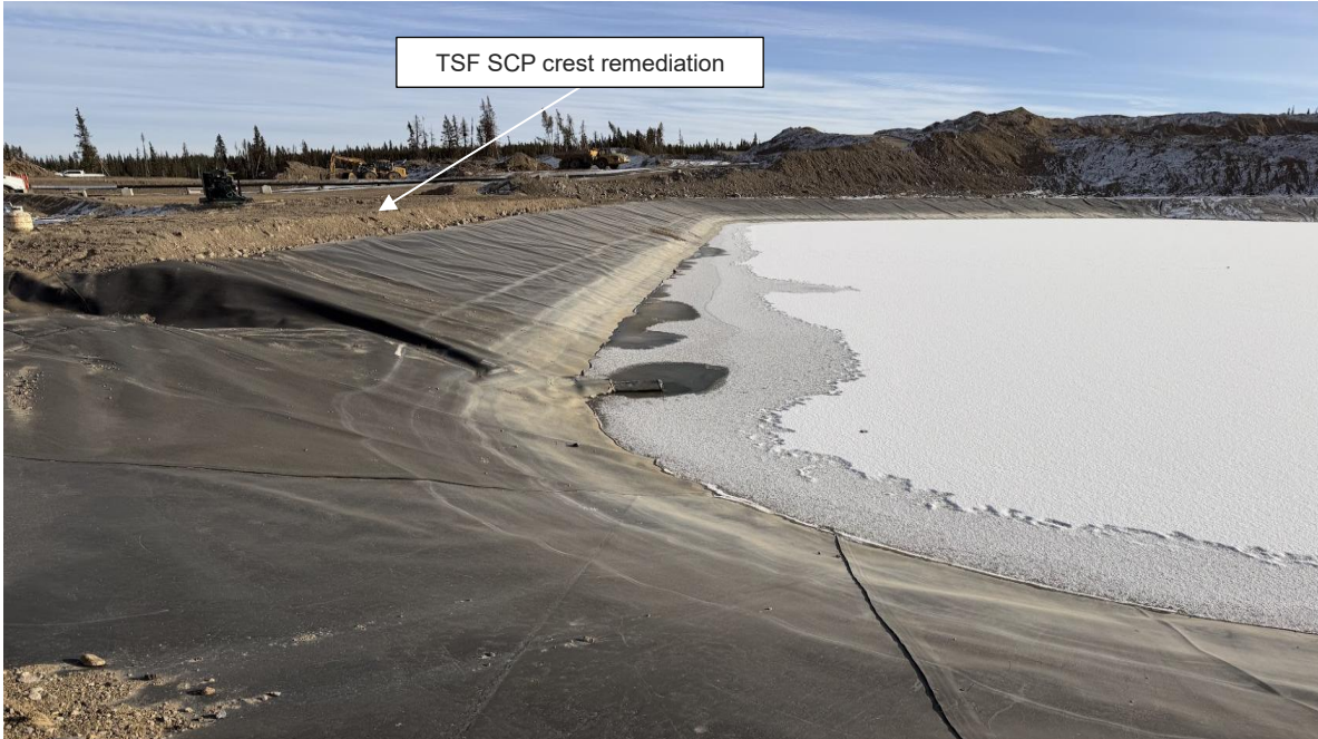
PHOTO 25 – TSF SCP north crest upstream slope and remediated north crest, looking east (Photo taken on November 28, 2025)
