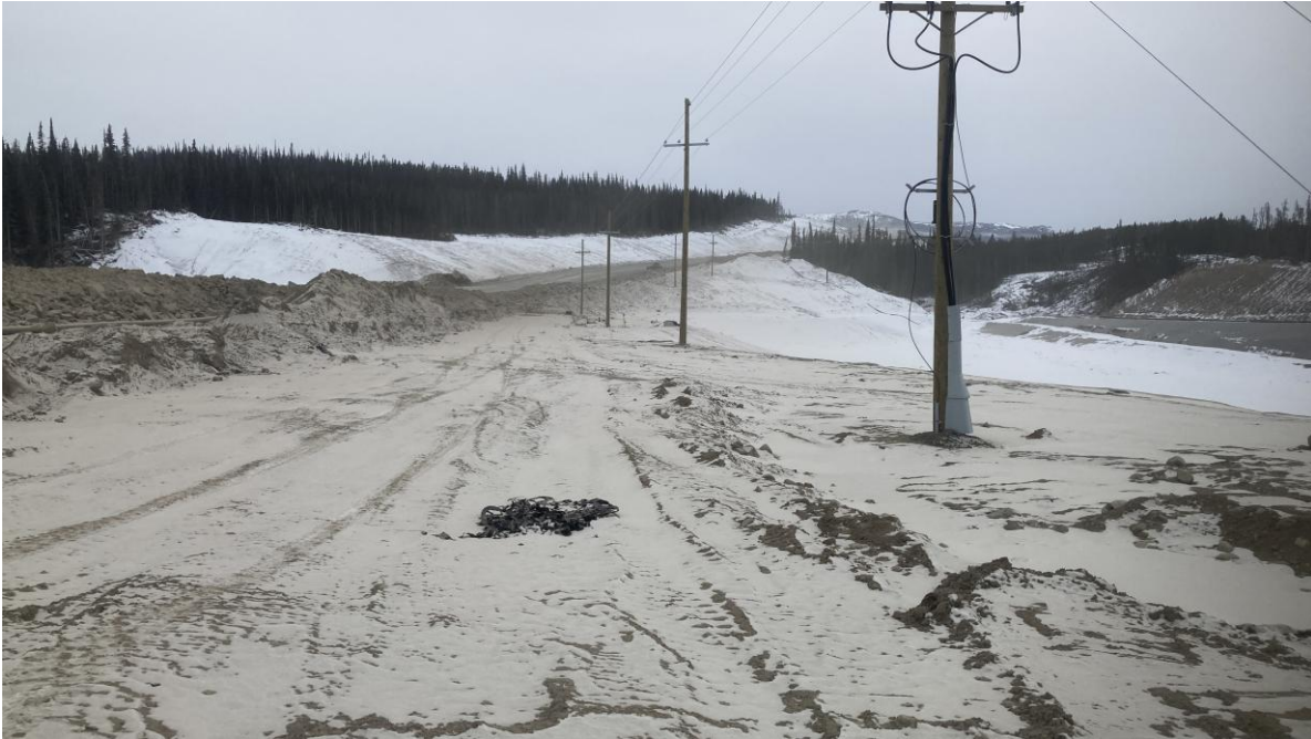
PHOTO 13 – East Berm crest, looking south (Photo taken on November 28, 2025)
