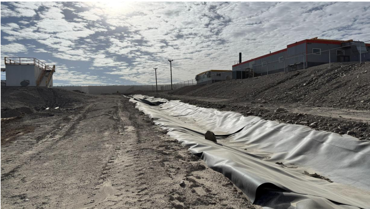
PHOTO 16 – SCC looking up-channel, looking south (Photo taken on October 13, 2025)
