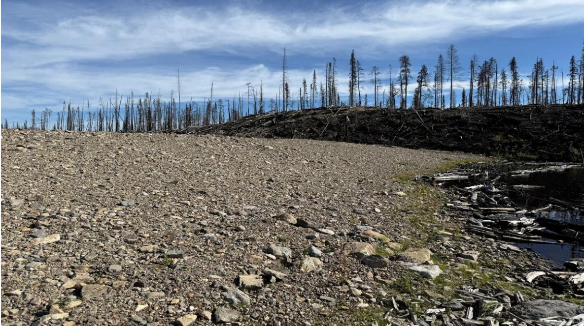
PHOTO 3 – Upstream slope, looking east (Photo taken on September 15, 2025)
