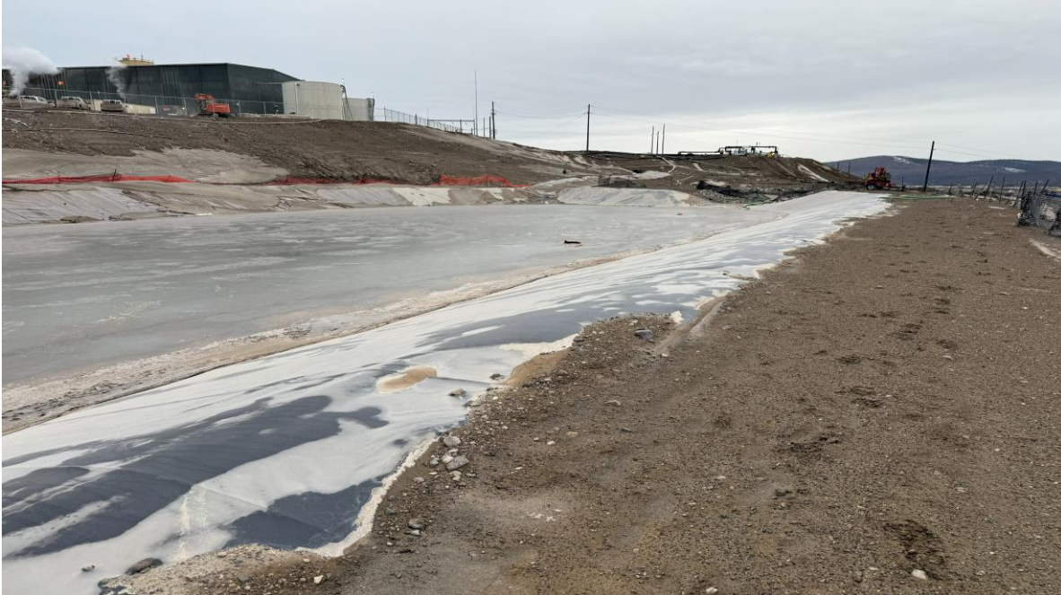
PHOTO 11 – SCP fill crest upstream slope, looking west (Photo taken on November 12, 2025)
