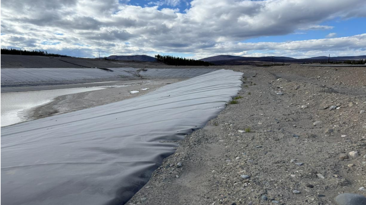
PHOTO 3 – Natural crest and upstream slope between North Berm and West Berm, looking west (Photo taken on October 11, 2025)
