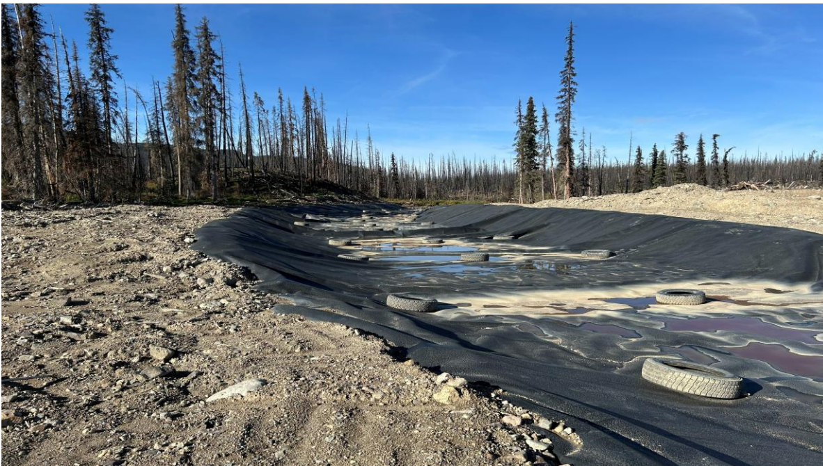
PHOTO 16 – LGO CP spillway, looking west from left side of spillway prior to liner replacement (Photo taken on September 19, 2025)
