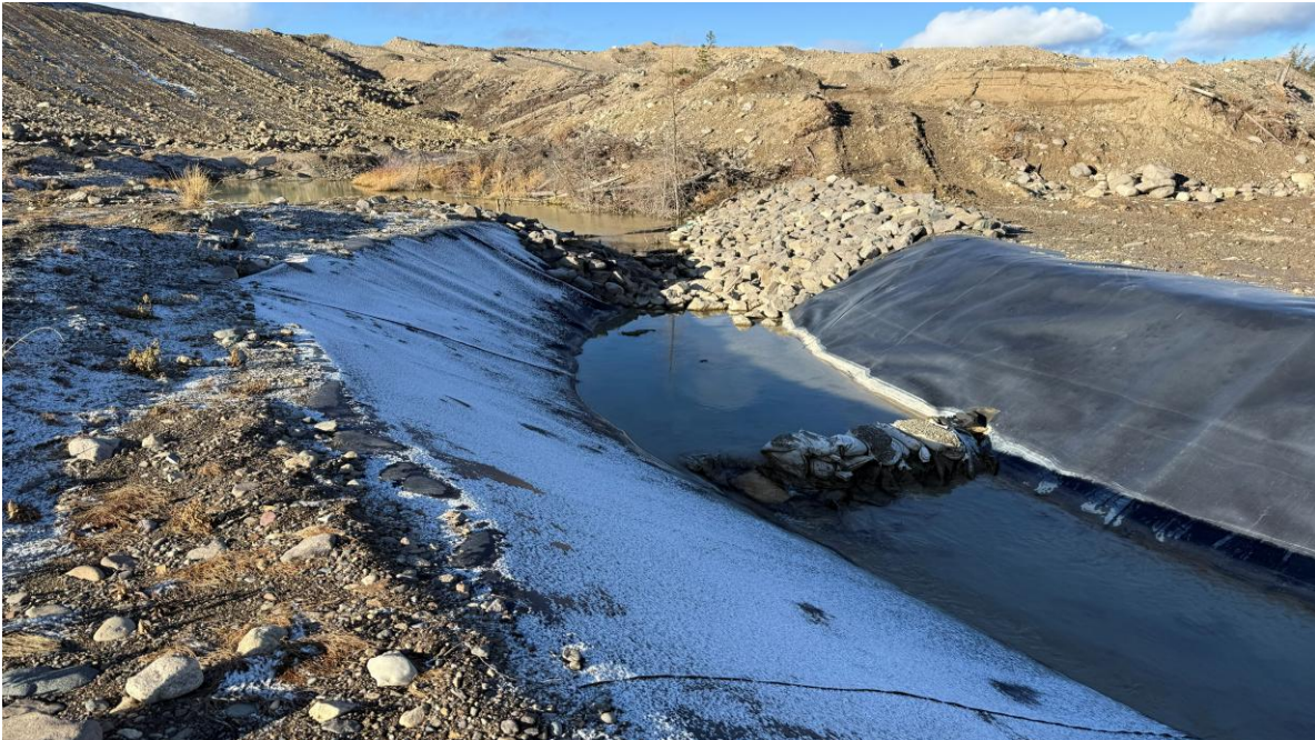
PHOTO 36 – TSF SCP inlet channel, looking west (Photo taken on November 11, 2025)
