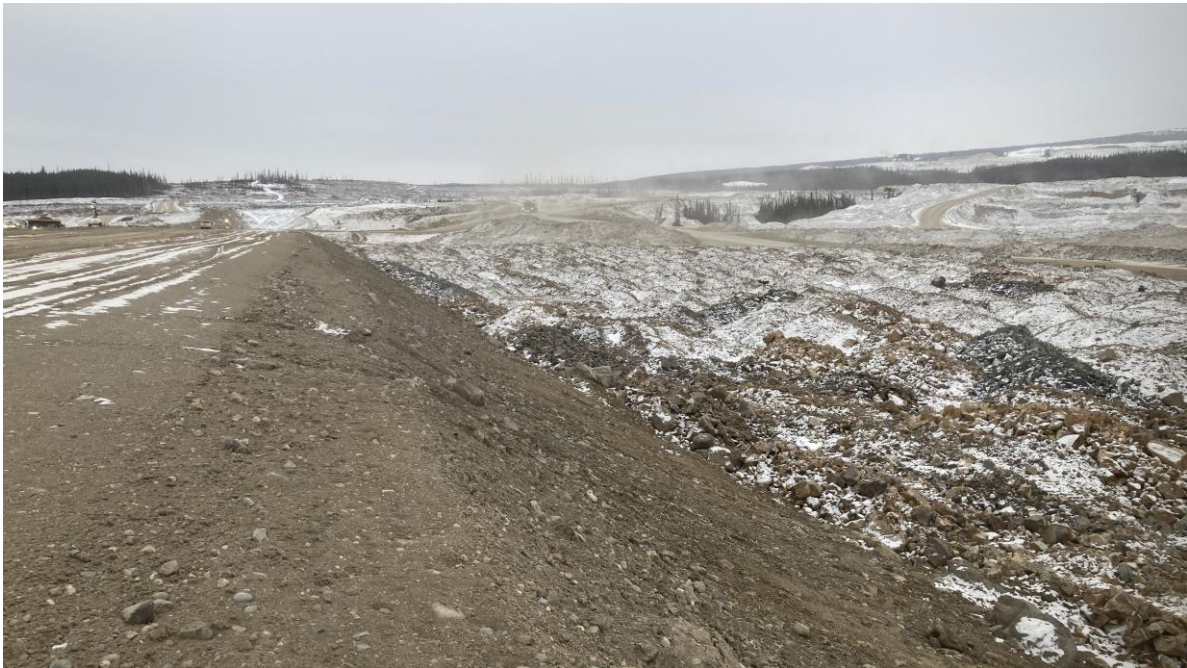
PHOTO 12 – MDC crest and upstream face and PAG waste rock dump, looking southeast (Photo taken on November 28, 2025)
