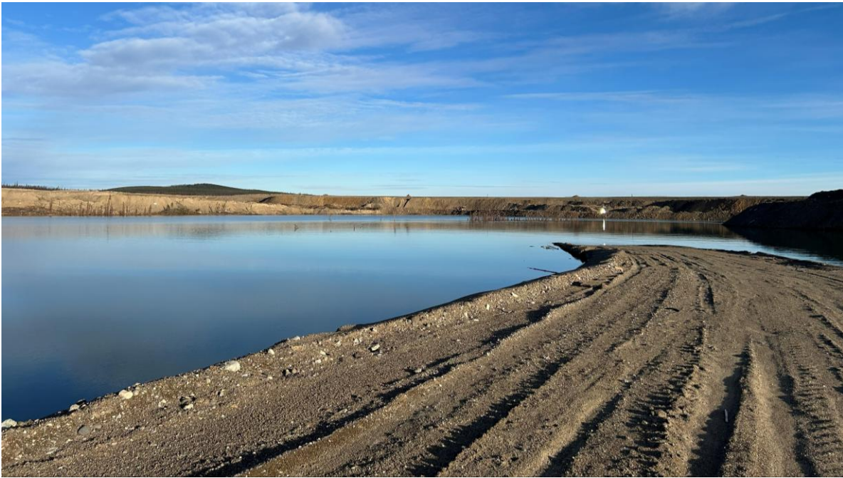
PHOTO 7 – Supernatant pond, PAG waste rock dump, and MDC upstream face, looking north near reclaim pump station (Photo taken on November 3, 2025)
