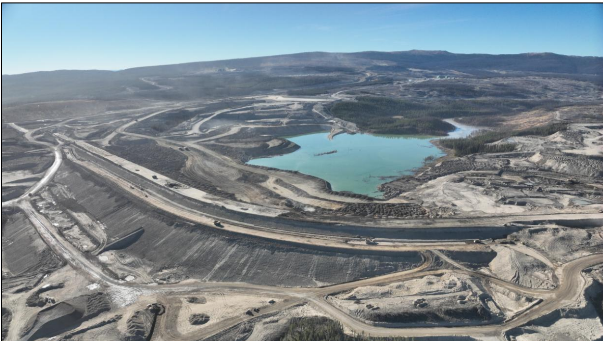
PHOTO 2 – TSF C overview, looking south (Photo taken on October 14, 2025)
