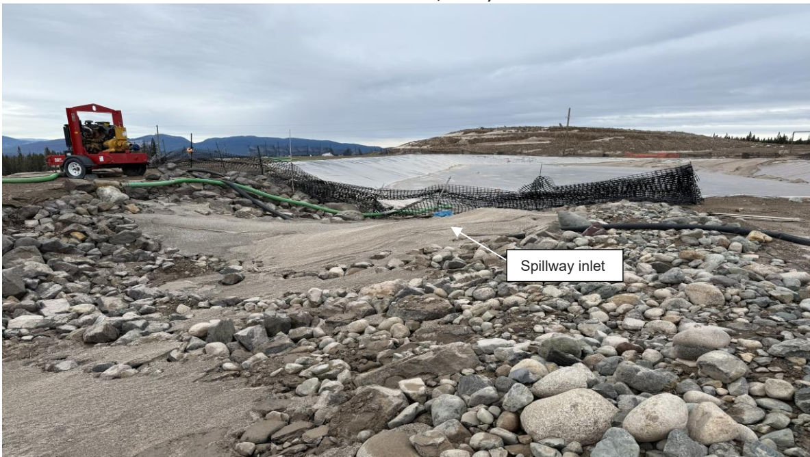
PHOTO 6 – SCP spillway inlet, looking east (Photo taken on November 12, 2025)
