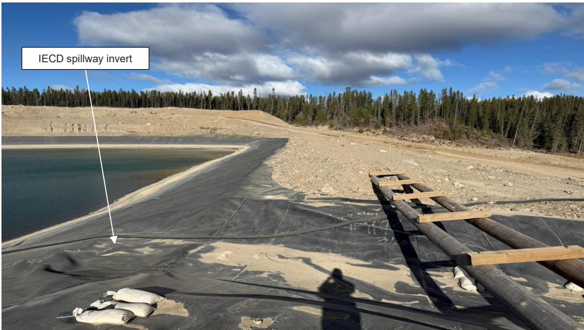
PHOTO 4 – IECD spillway inlet, looking northwest (Photo taken on October 12, 2025)
