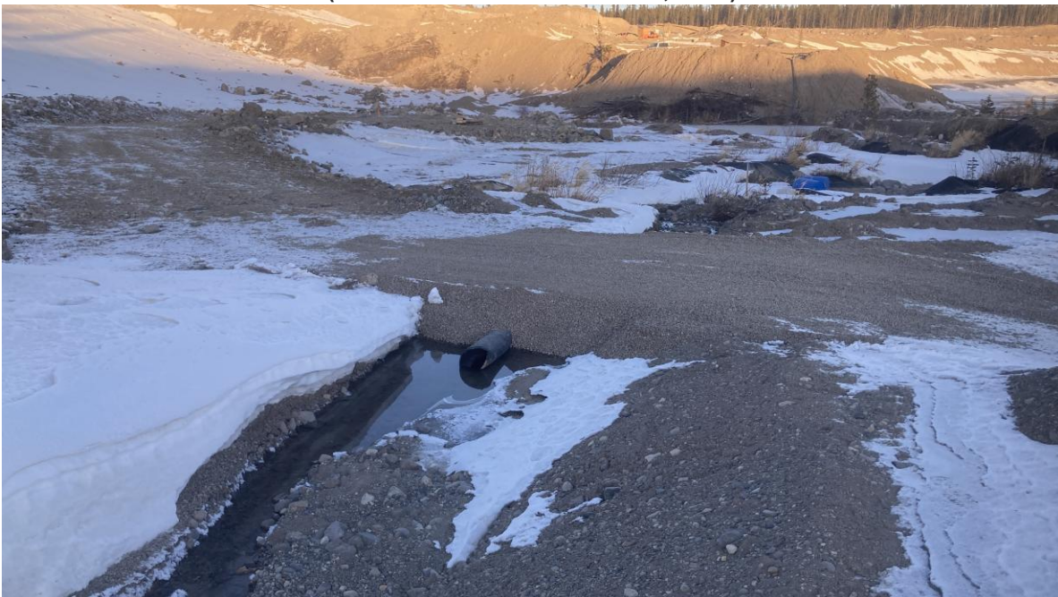
PHOTO 32 – Culvert crossing over the east foundation drain outlet channel (Photo taken on January 24, 2026)
