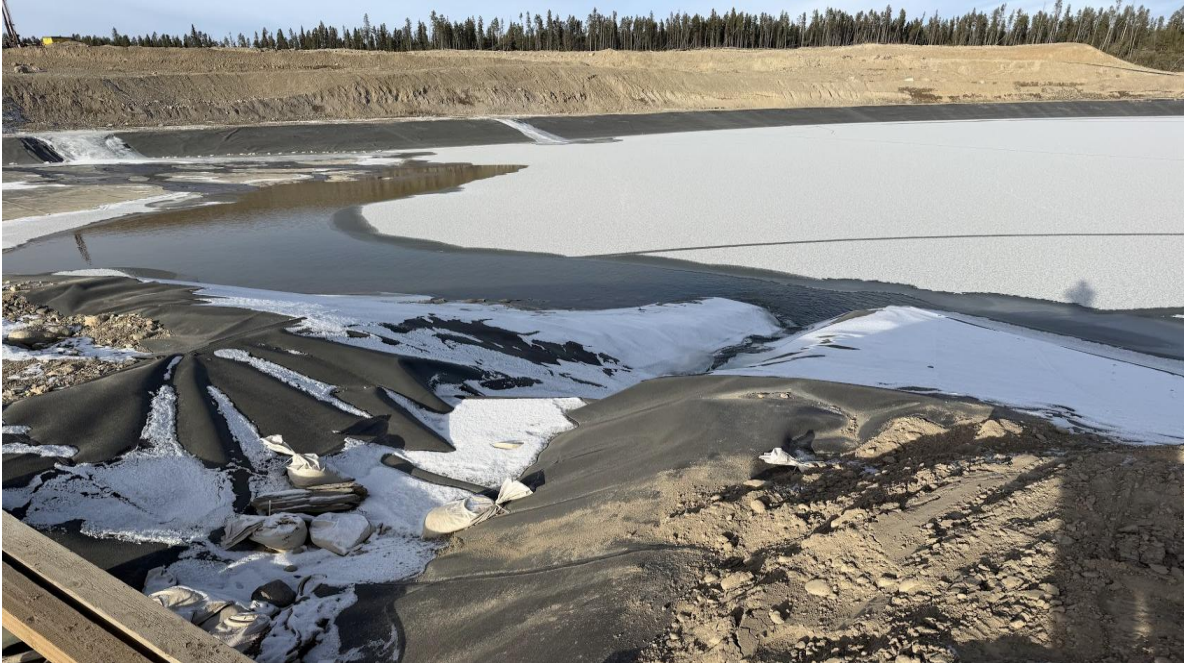
PHOTO 21 – TSF SCP spillway, looking northwest (Photo taken on November 28, 2025)
