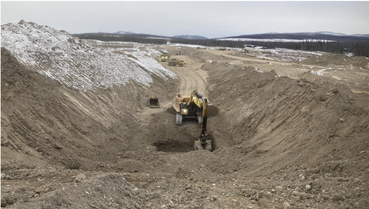
PHOTO 17 – MDC west cut-off trench excavation, looking west (Photo taken on November 28, 2025)
