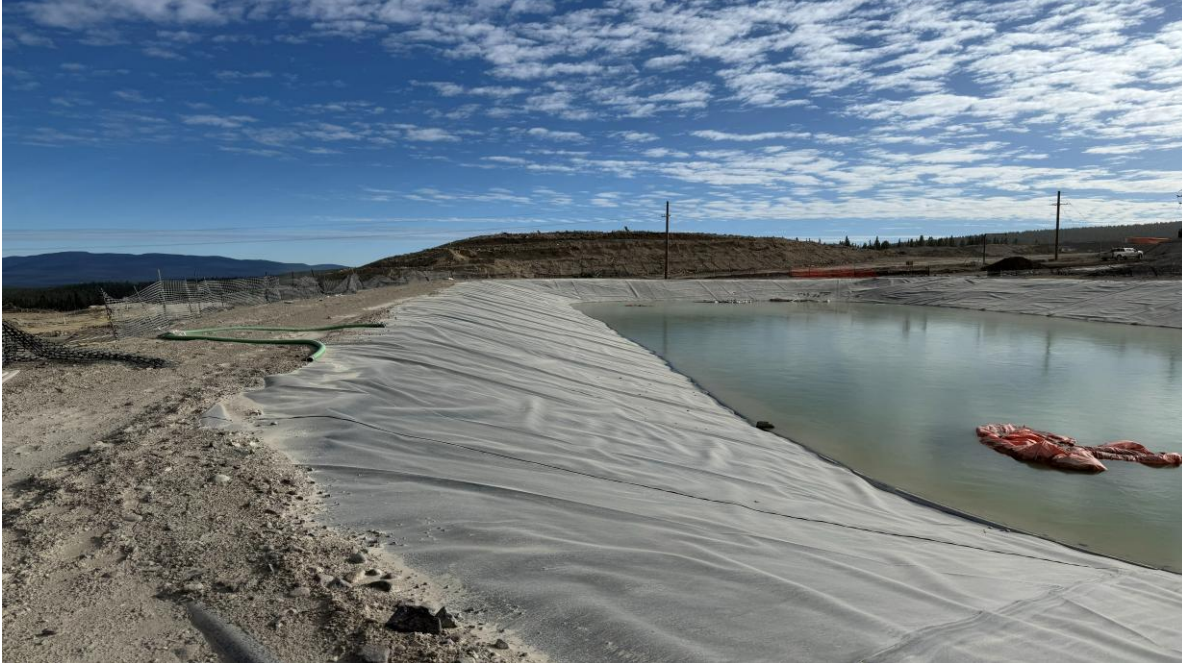
PHOTO 9 – SCP fill crest upstream slope, looking east (Photo taken on October 13, 2025)
