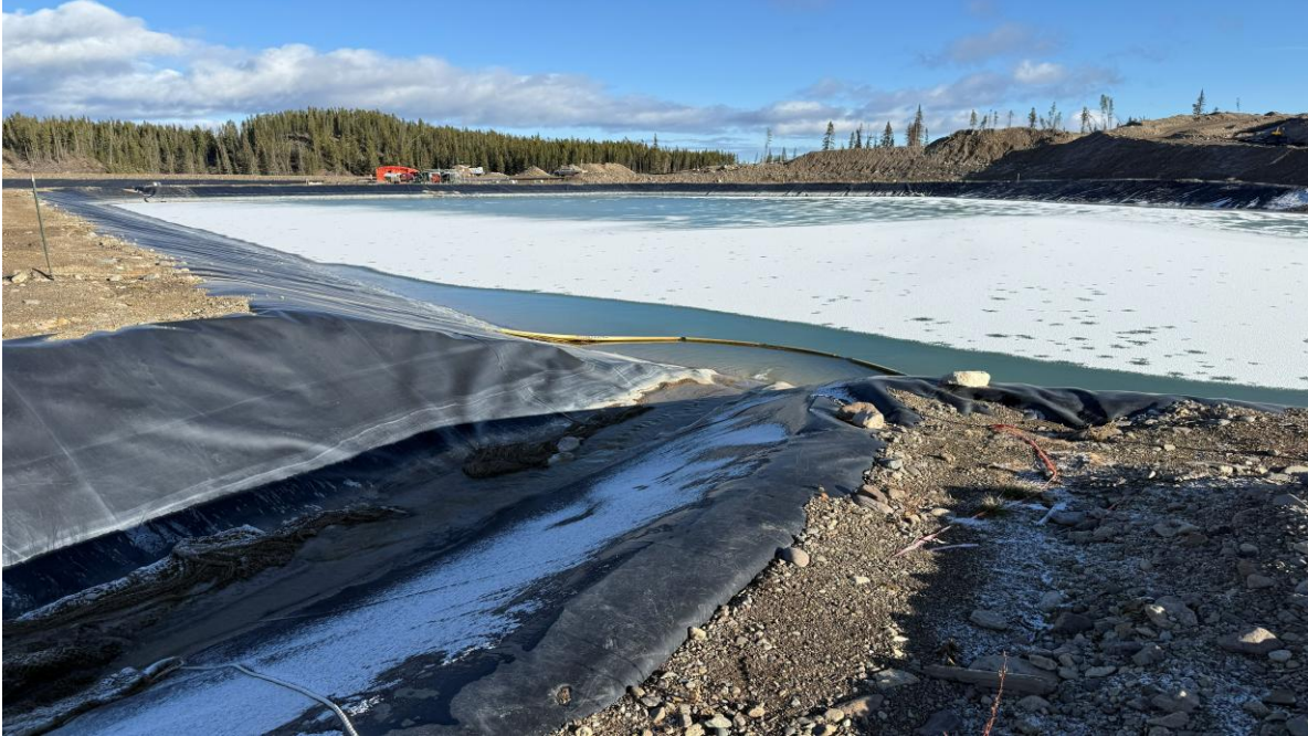
PHOTO 35 – TSF SCP inlet channel outlet, looking northeast (Photo taken on November 11, 2025)
