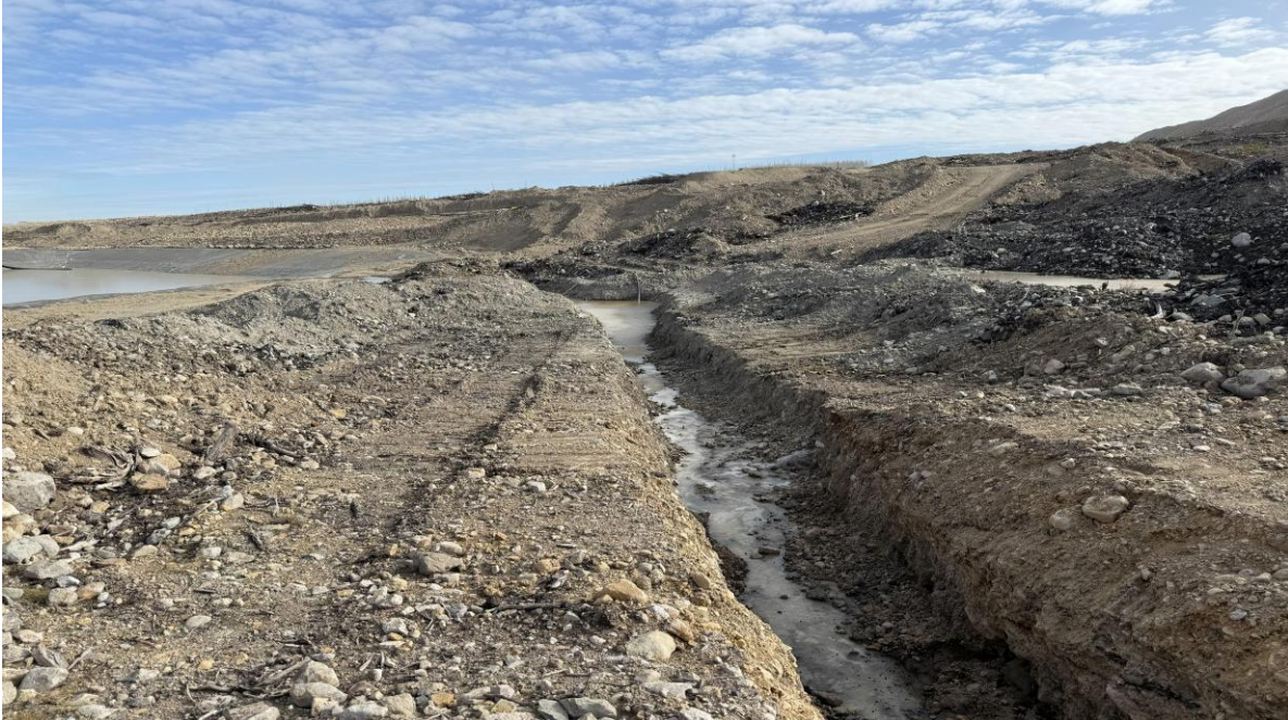
PHOTO 9 – LGO CP south interception ditch, looking east (Photo taken on October 13, 2025)
