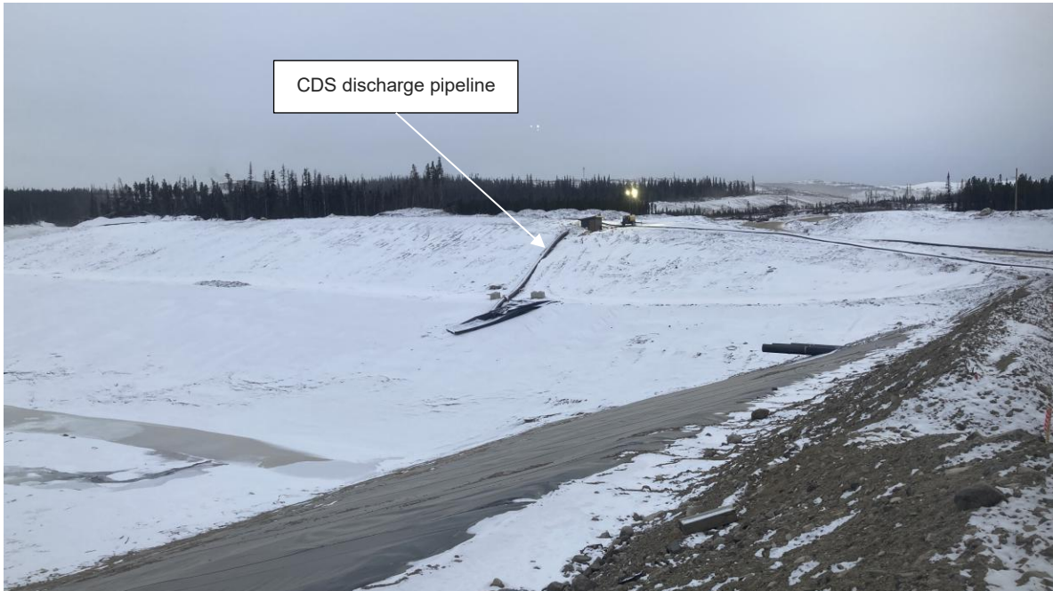
PHOTO 19 – CDS discharge pipeline, looking south (Photo taken on September 19, 2025)
