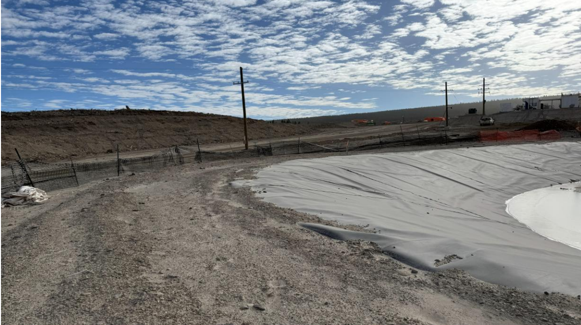
PHOTO 13 – PS SCP Pond and road (Photo taken on October 13, 2025)
