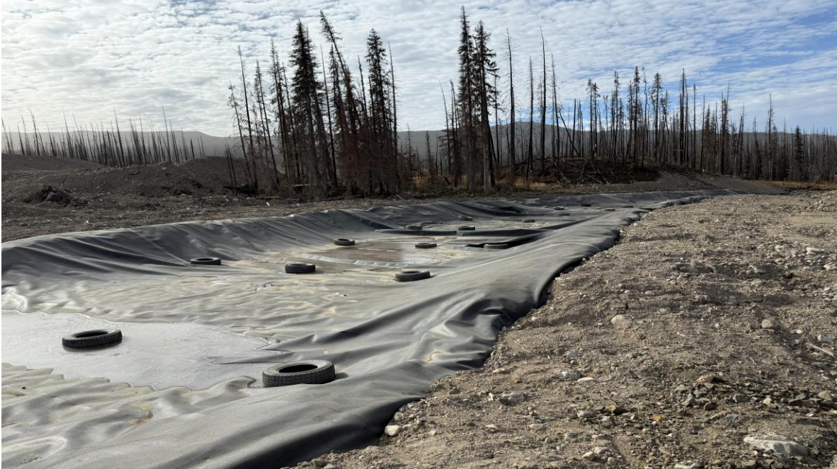
PHOTO 15 – LGO CP spillway, looking west from right side of spillway prior to liner replacement (Photo taken on October 13, 2024)
