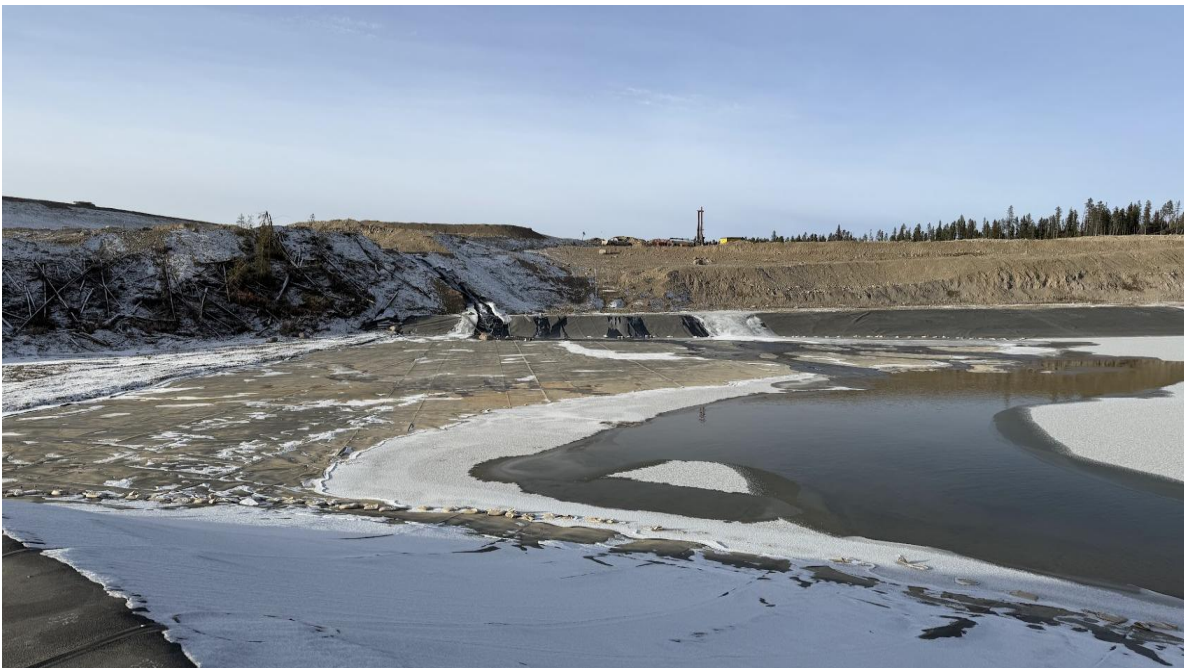
PHOTO 20 – IECD basin inlet, looking west (Photo taken on November 28, 2025)
