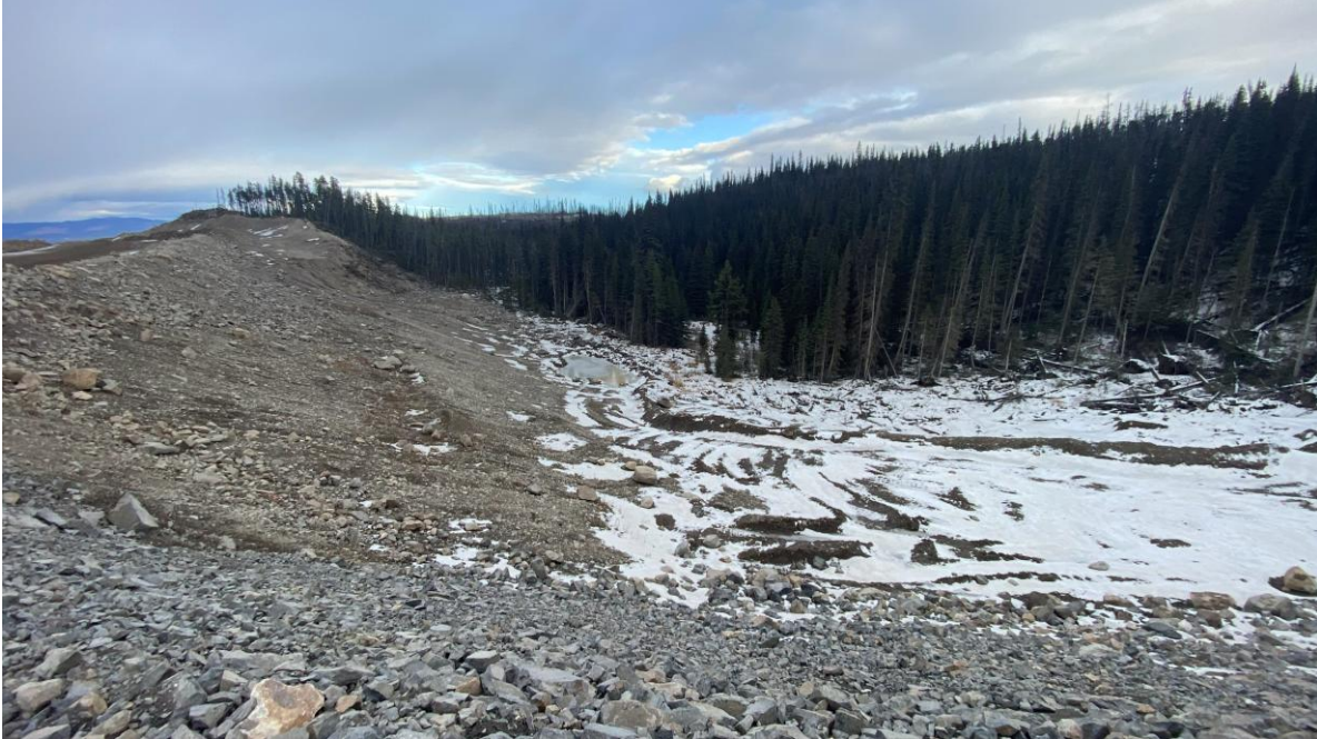
PHOTO 15 – East Berm haul road downstream slope, looking north (Photo taken on October 31, 2025)
