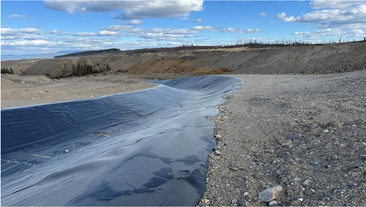
PHOTO 7 – Spillway looking north from just down-channel of the inlet, looking down-channel (northeast) (Photo taken on October 27, 2025)
