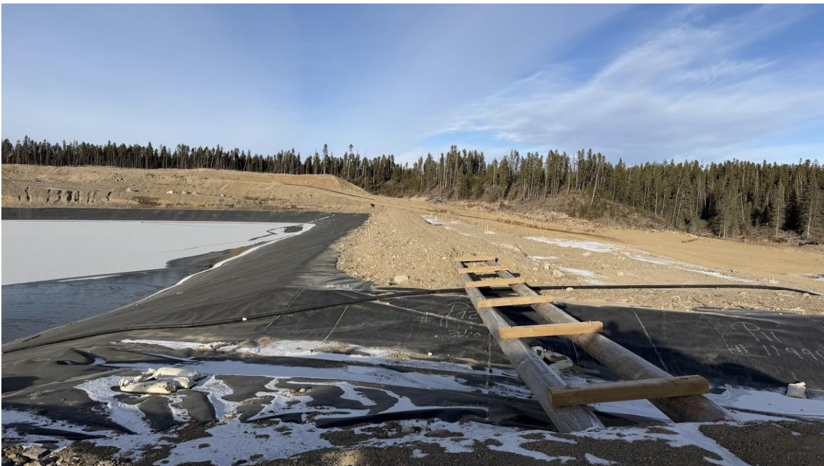
PHOTO 8 – IECD crest post remediation, looking northwest (Photo taken on November 28, 2025)
