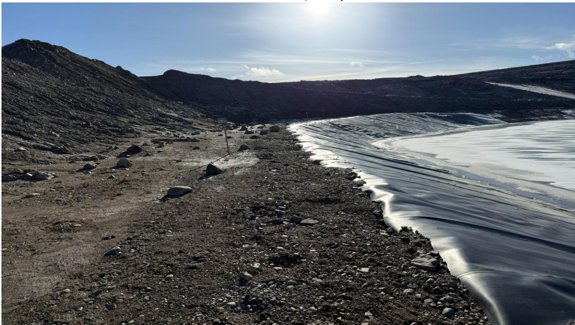
PHOTO 28 – TSF SCP east cut crest and upstream slope, looking south (Photo taken on November 11, 2025)
