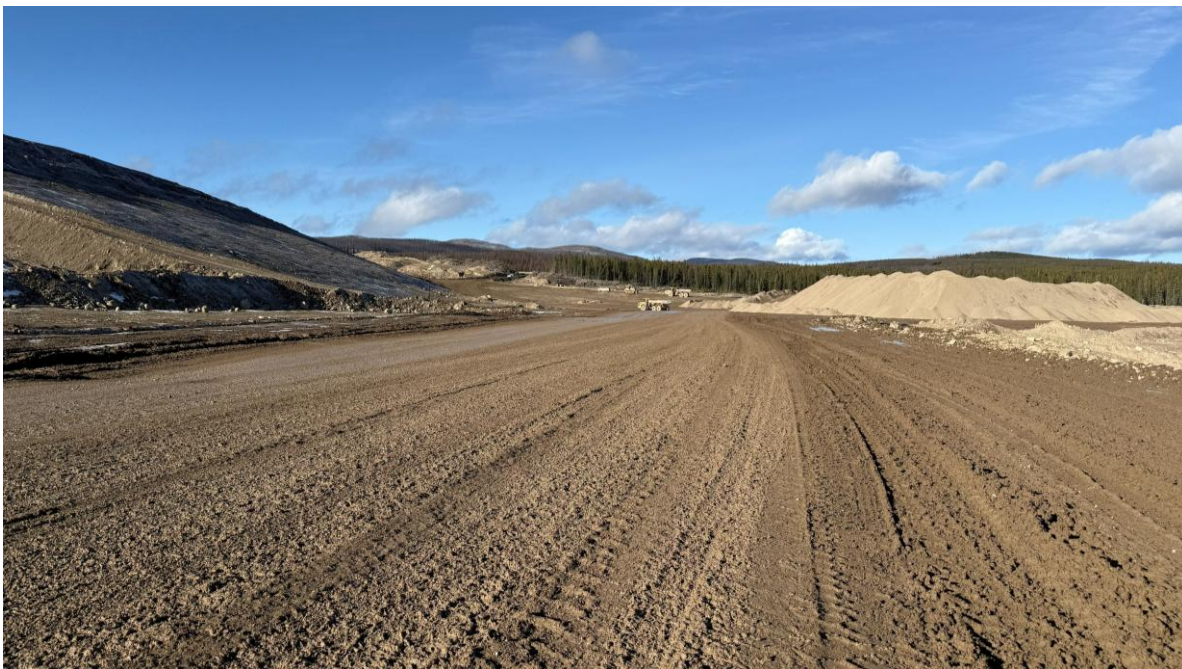
PHOTO 22 – MDC downstream buttress crest surface, looking northeast (Photo taken on November 11, 2025)
