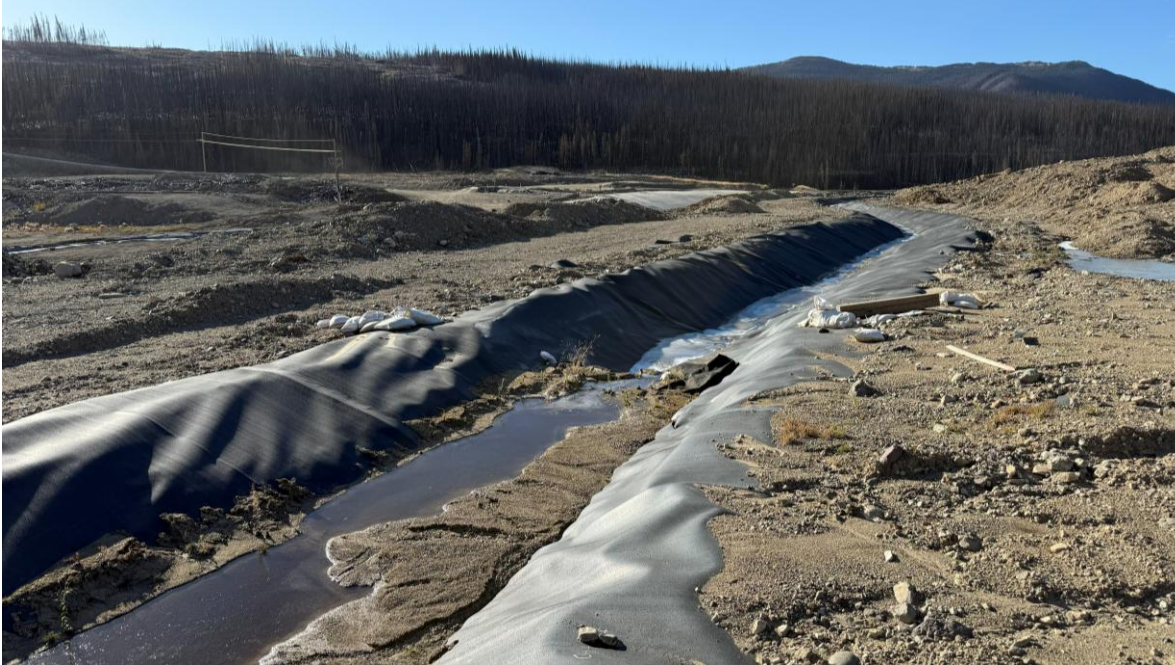
PHOTO 19 – Sediment accumulation in the NCC, looking south (Photo taken on October 13, 2025)
