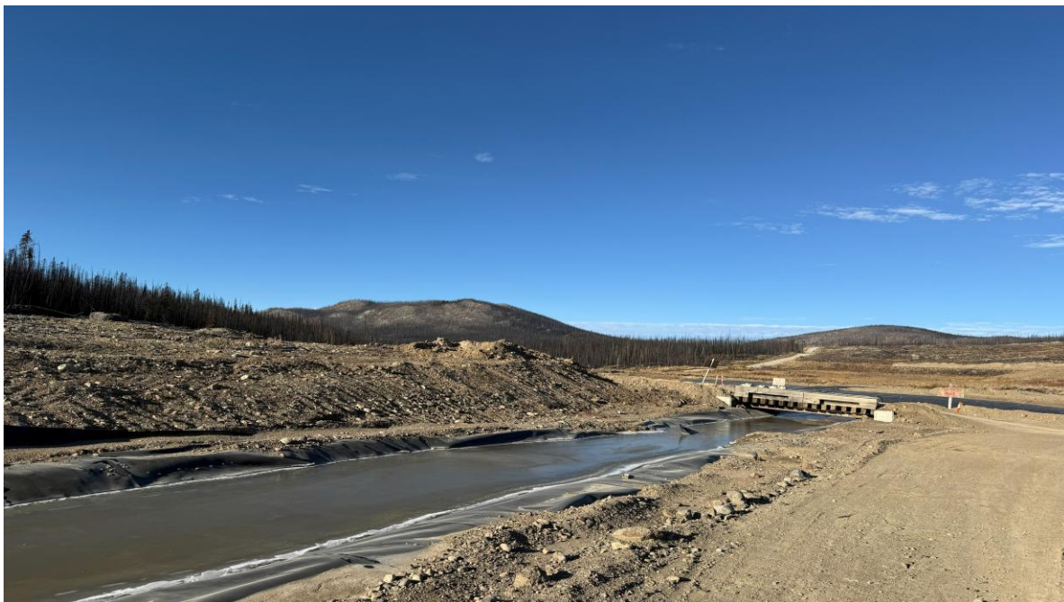
PHOTO 16 – SCC near its outlet, looking west (Photo taken on October 13, 2025)
