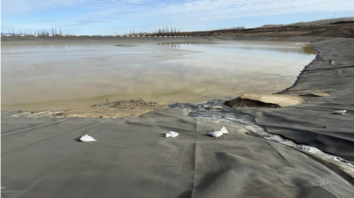
PHOTO 11 – LGO CP sediment accumulation at the WCC inlet, looking east (Photo taken on October 13, 2025)
