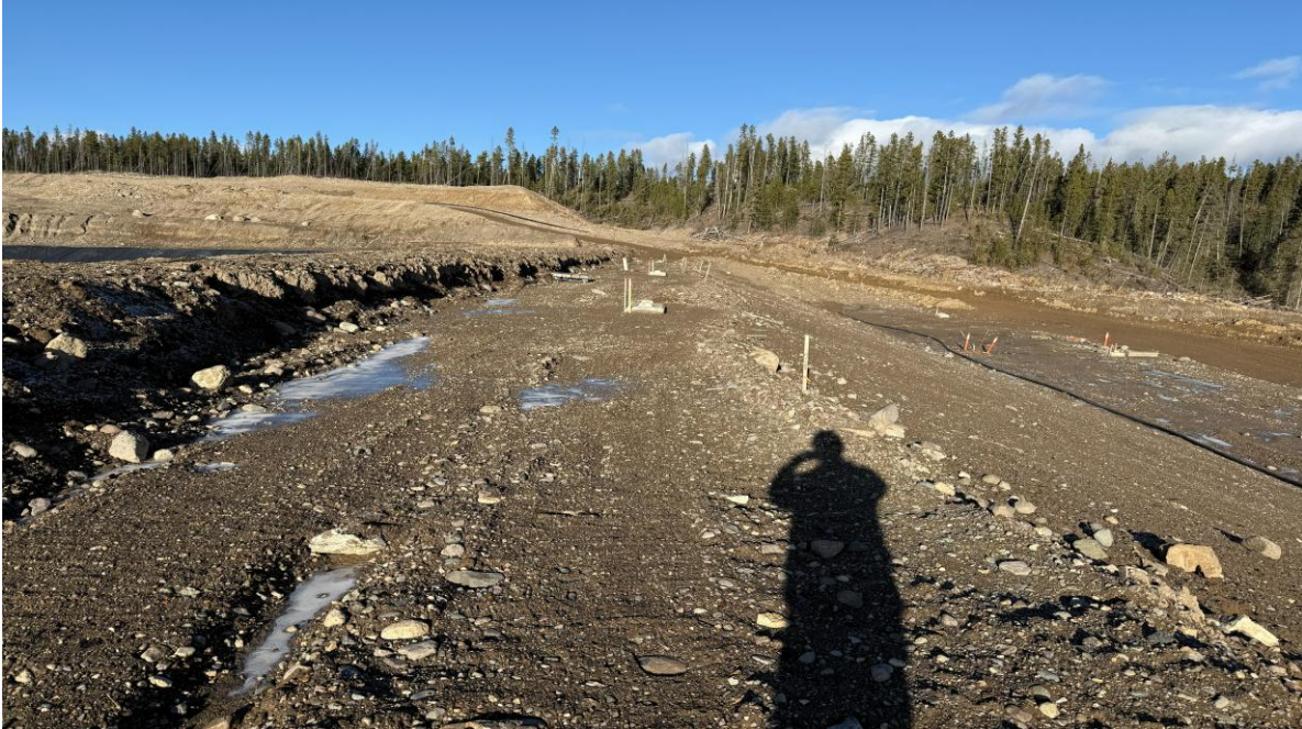
PHOTO 7 – IECD crest post remediation, looking northwest (Photo taken on November 11, 2025)
