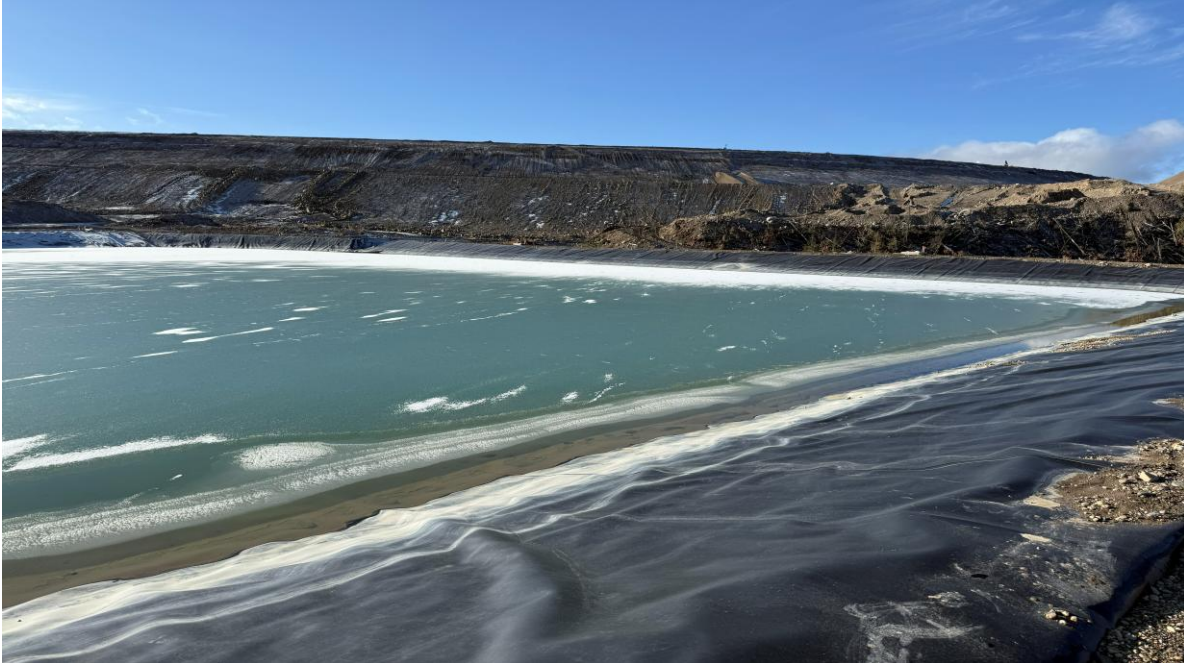
PHOTO 27 – TSF SCP east cut crest upstream slope, looking northwest (Photo taken on November 11, 2025)
