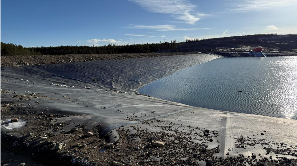
PHOTO 9 – IECD upstream slope, looking southeast (Photo taken on November 11, 2025)
