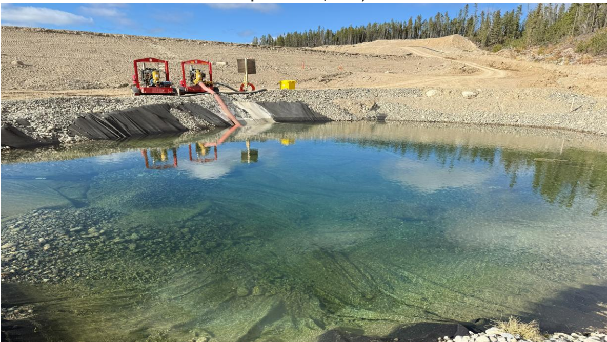
PHOTO 16 – IECD seepage collection sump, looking southwest (Photo taken on October 12, 2025)
