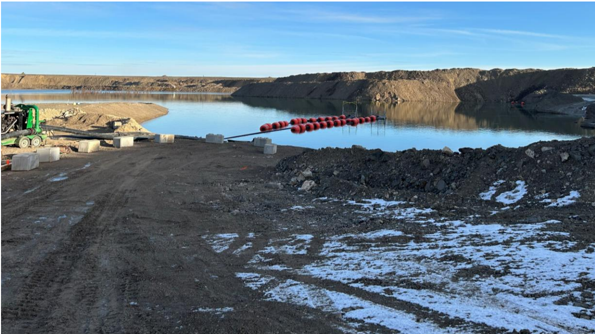
PHOTO 8 – Reclaim water system intake and supernatant pond, looking north (Photo taken on November 3, 2025)
