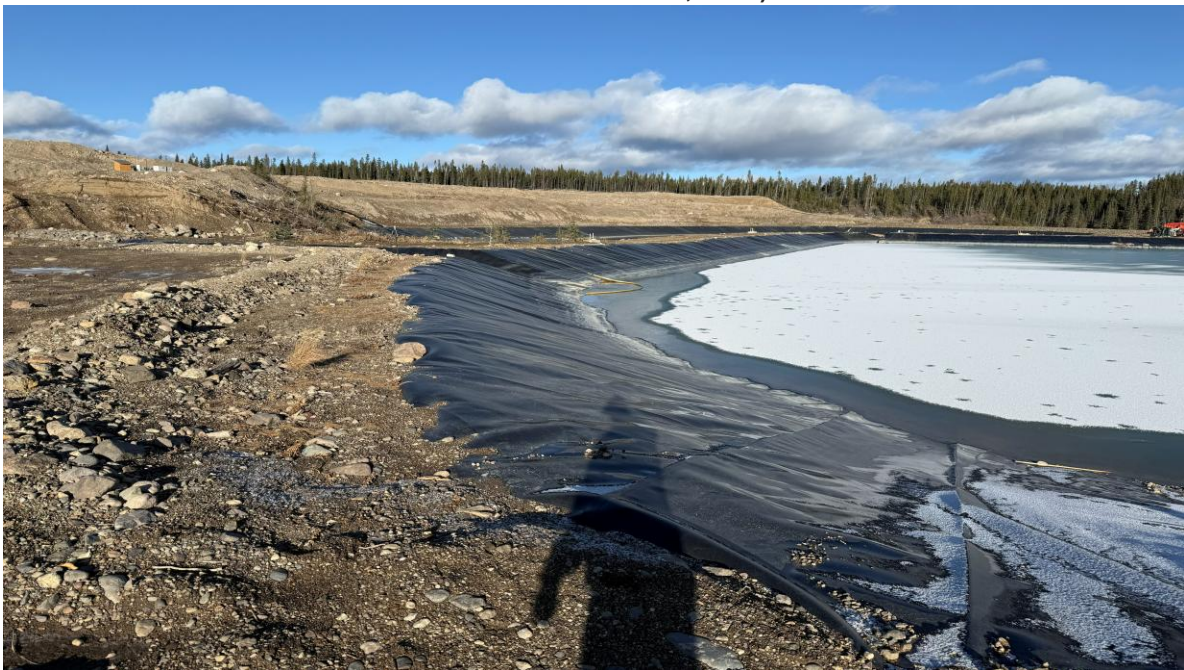
PHOTO 34 – TSF SCP southwest crest upstream slope, looking northwest (Photo taken on November 11, 2025)
