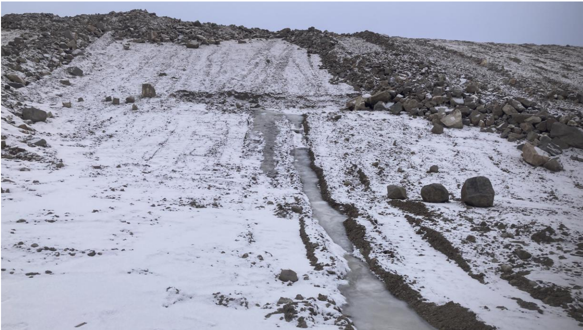
PHOTO 25 – Drainage channel excavated to convey the seepage downstream towards the east foundation drain, looking southwest (Photo taken on November 28, 2025)
