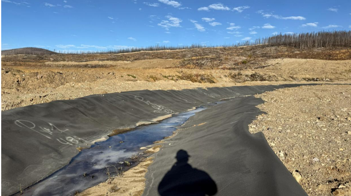
PHOTO 21 – NCC, looking south (Photo taken on October 13, 2025)
