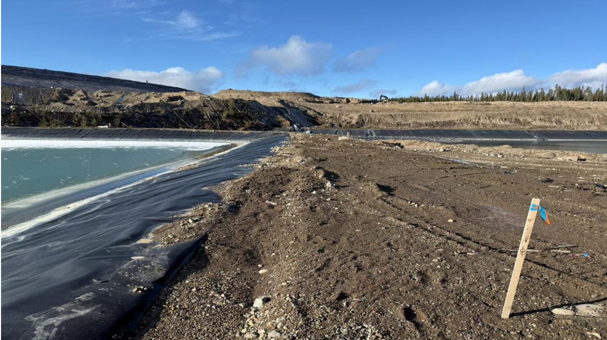
PHOTO 23 – TSF SCP north crest and liner anchor trench depression, looking west (Photo taken on November 11, 2025)
