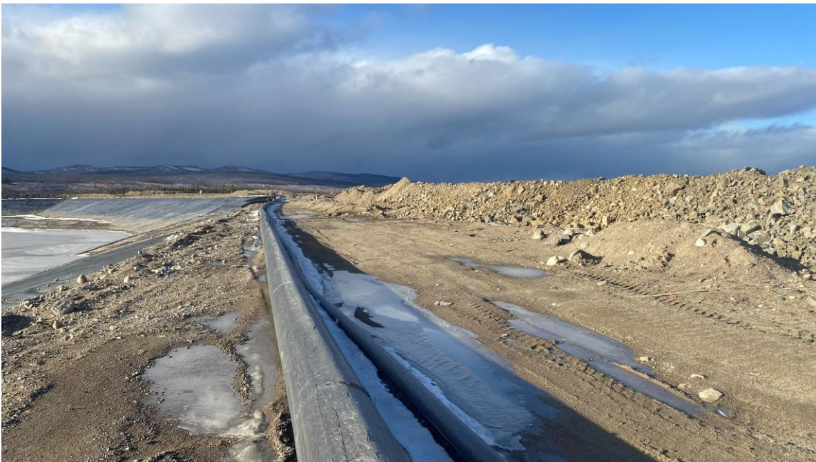
PHOTO 2 – North Berm crest and pipeline, looking northwest (Photo taken on October 31, 2025)
