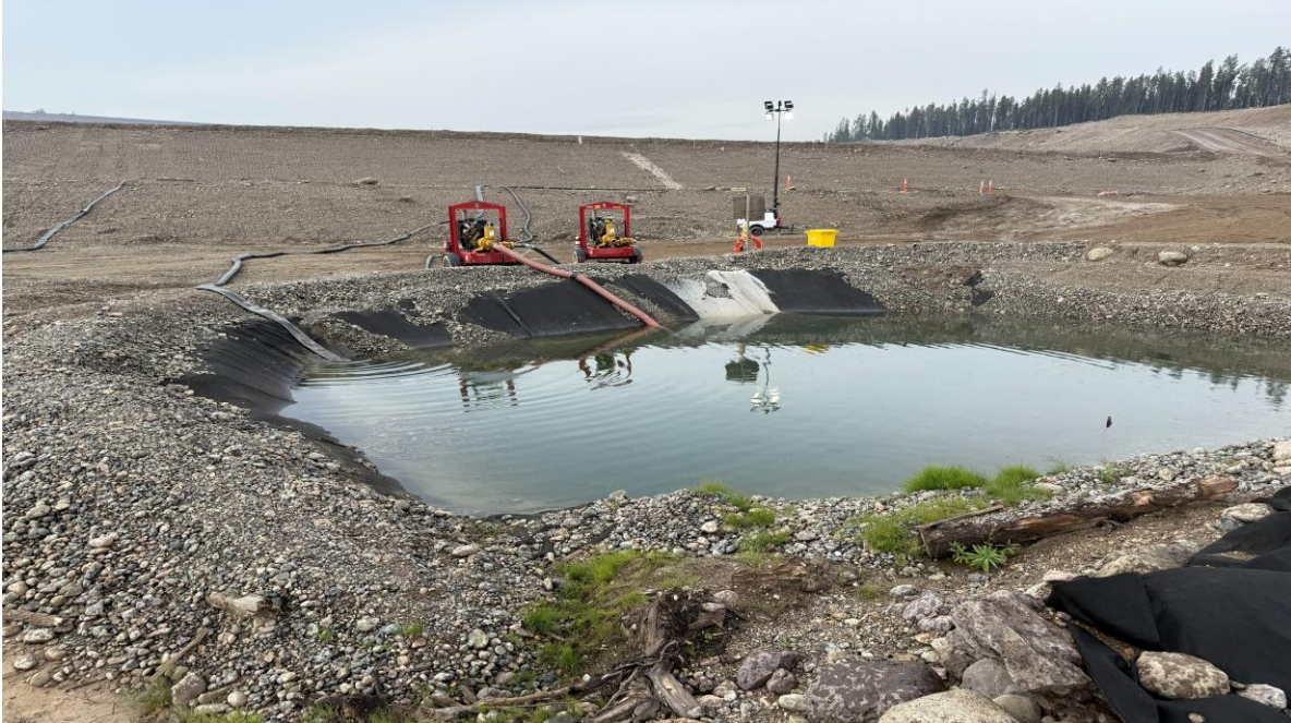
PHOTO 15 – IECD seepage collection sump, looking southwest (Photo taken on September 13, 2025)
