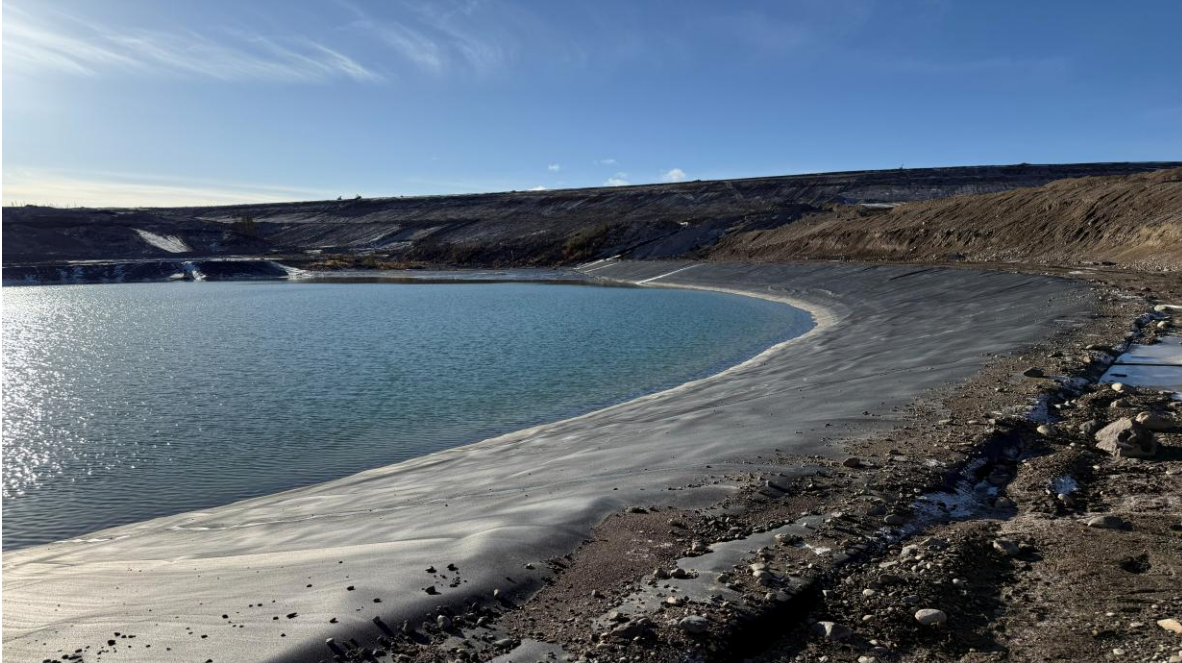
PHOTO 17 – IECD north and west cut slopes, looking south (Photo taken on November 11, 2025)
