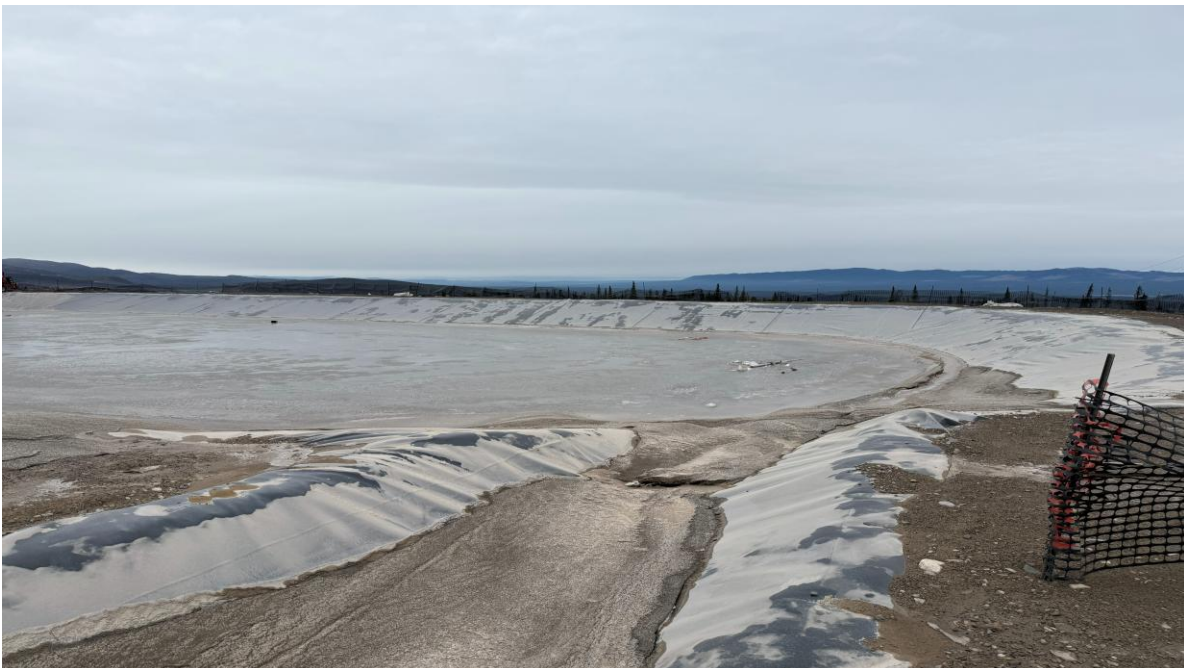
PHOTO 14 – SCC inlet to the SCP, looking north (Photo taken on November 12, 2025)
