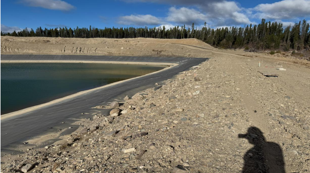
PHOTO 5 – IECD crest, looking northwest (Photo taken on October 12, 2025)
