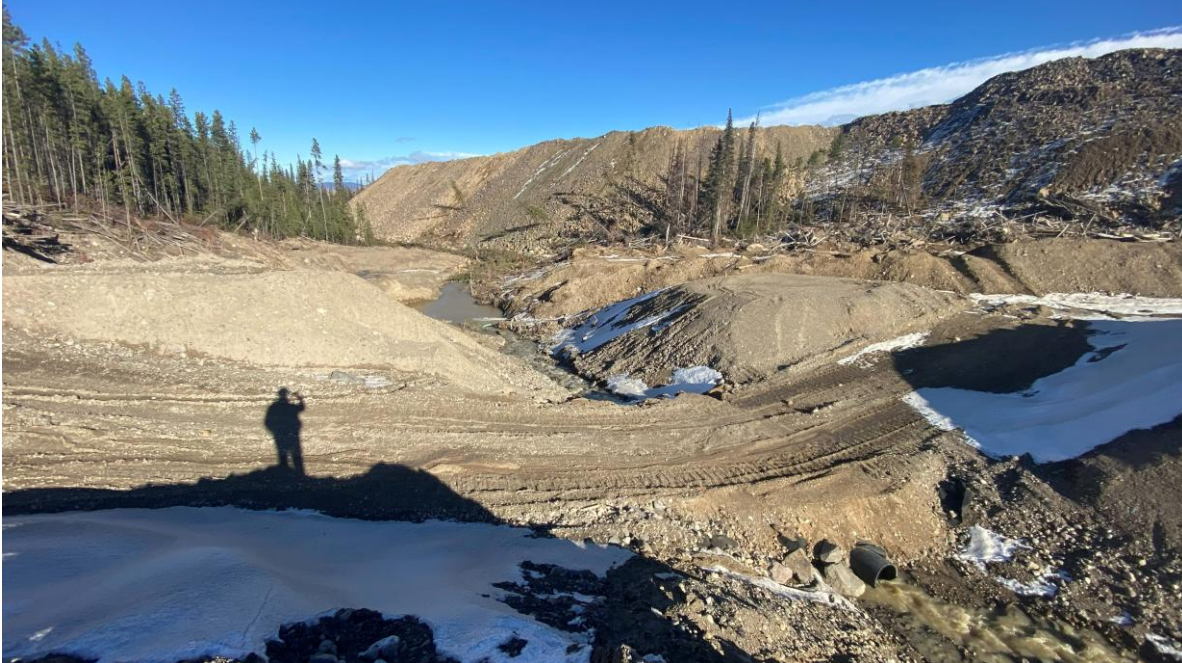
PHOTO 9 – Culvert crossing of historic Mine Area Creek downstream of the spillway outlet, looking north (Photo taken on October 31, 2025)
