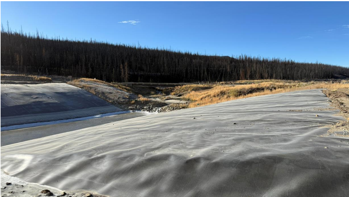
PHOTO 2 – CWTP inlet looking upstream (southwest) from the NCC outlet (Photo taken on November 28, 2025)
