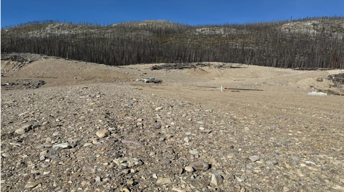
PHOTO 5 – Upstream slope and crest looking west (Photo taken on October 13, 2025)
