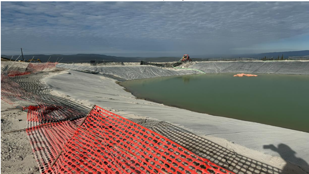
PHOTO 4 – SCP cut slope upstream slope, NCC inlet, and spillway, looking west (Photo taken on October 13, 2025)
