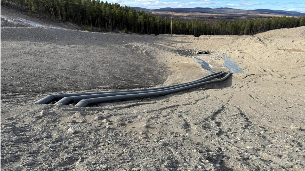
PHOTO 23 – West Berm Outlet Pipes along downstream slope, looking west (Photo taken on November 28, 2025)
