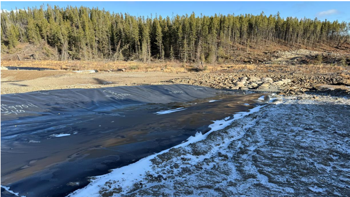
PHOTO 14 – IECD spillway outlet, looking north (Photo taken on November 11, 2025)
