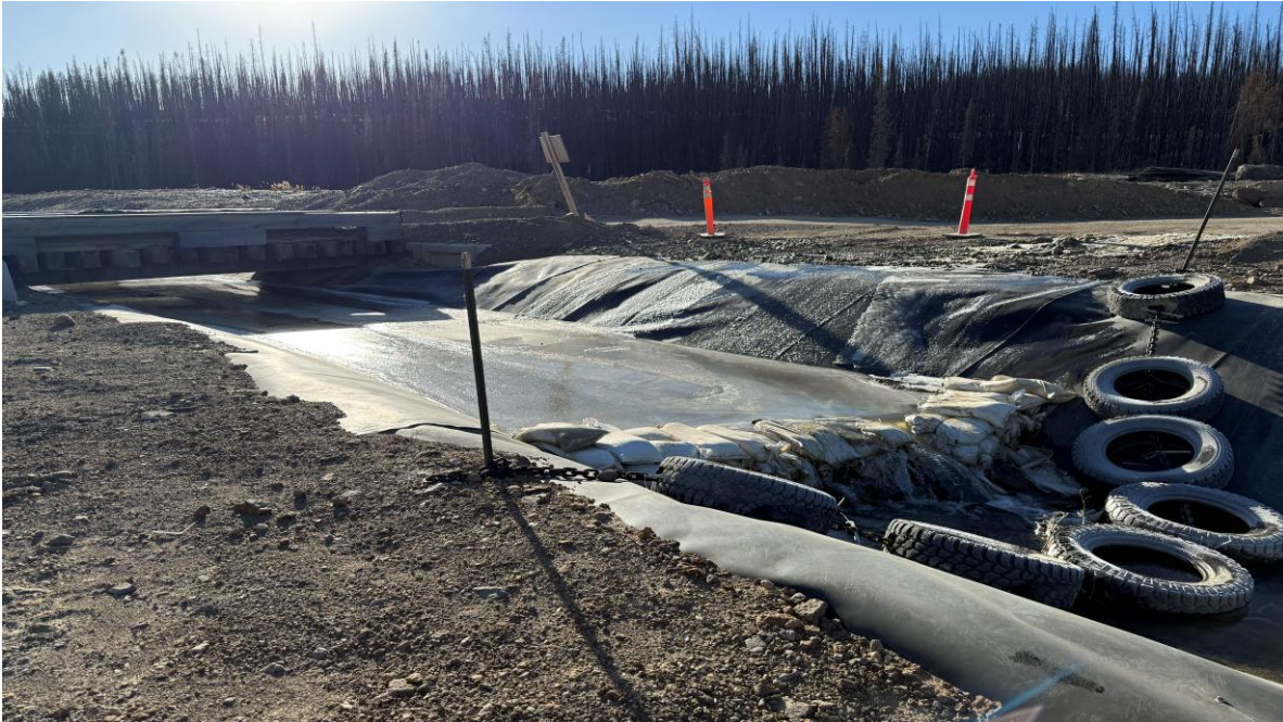
PHOTO 15 – Check dam established in SCC near the channel outlet, looking east (Photo taken on October 13, 2025)
