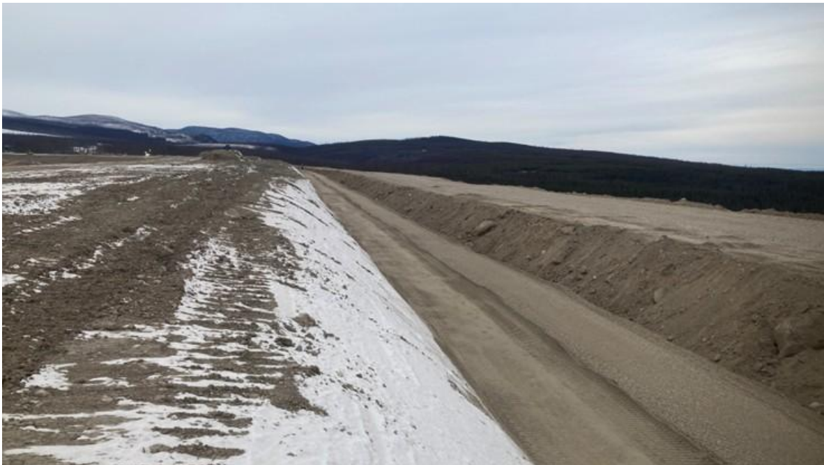
PHOTO 16 – MDC filter zones (Zones F and T) and downstream shell (Zone C) construction, looking northwest (Photo taken on November 28, 2025)
