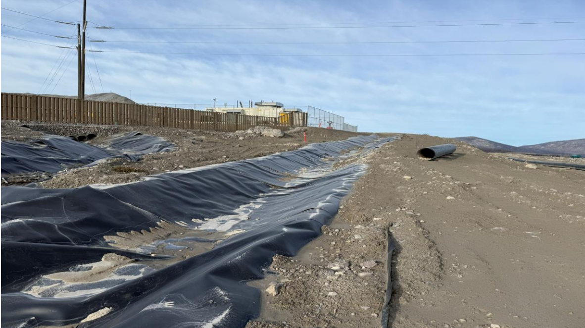
PHOTO 19 – NCC near its inlet looking up-channel, west (Photo taken on September 15, 2025)
