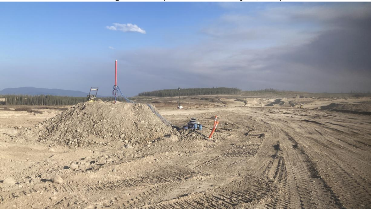
PHOTO 36 – MDC-S0-PZ3 inclinometer being raised during active crest construction (Photo taken on September 7, 2025)
