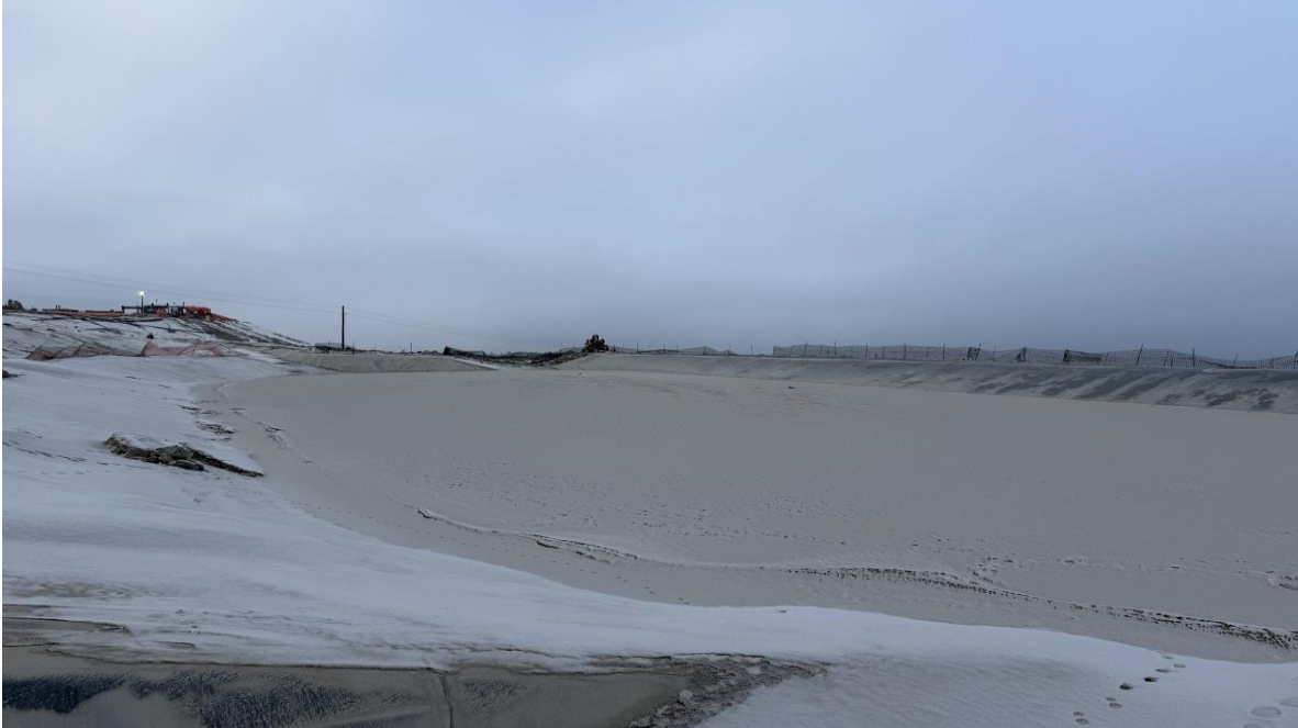
PHOTO 1 – SCP, looking west (Photo taken on November 28, 2025)
