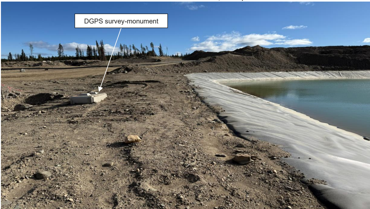
PHOTO 24 – TSF SCP north crest, looking east (Photo taken on October 12, 2025)
