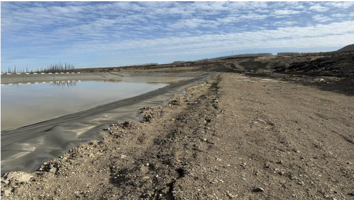
PHOTO 8 – LGO CP south cut crest and minor anchor backfill settling, looking east (Photo taken on October 13, 2025)
