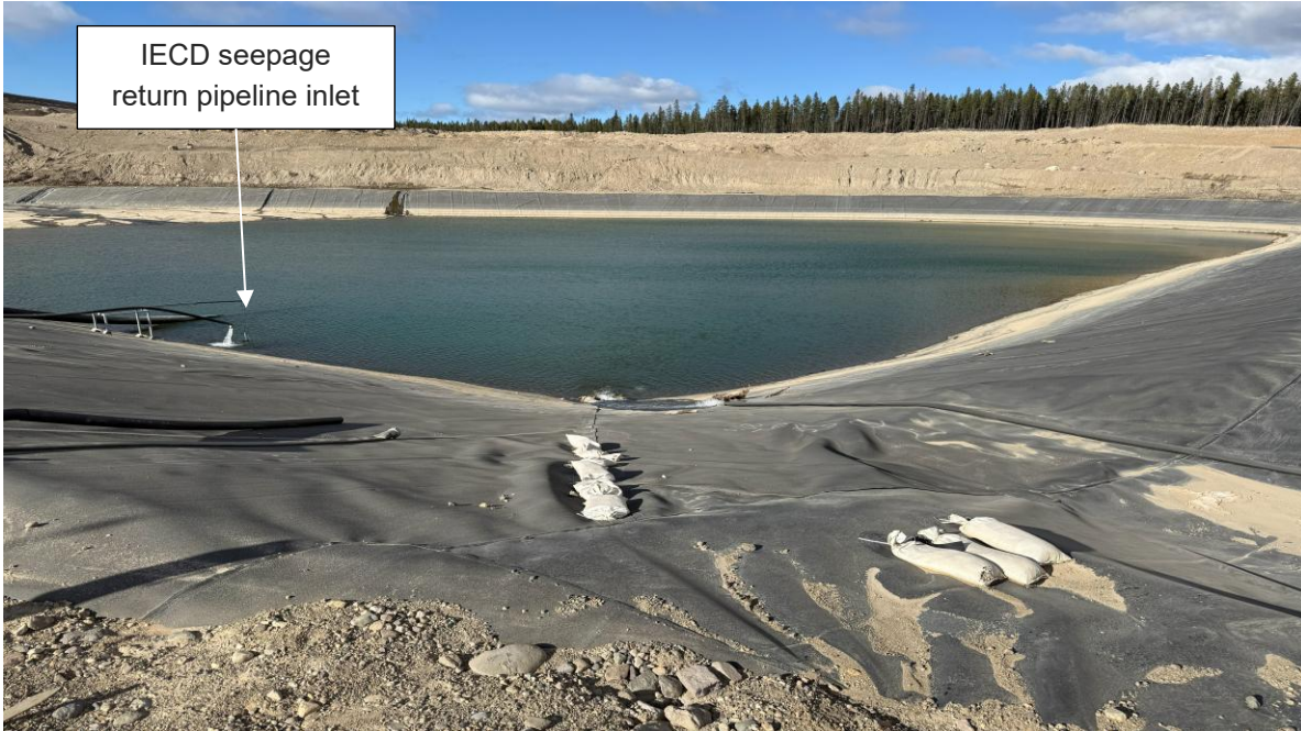
PHOTO 3 – IECD upstream slope at the spillway and pond, looking northwest (Photo taken on October 12, 2025)
