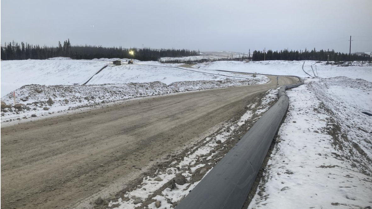
PHOTO 21 – West Berm crest, looking south (Photo taken on November 28, 2025)
