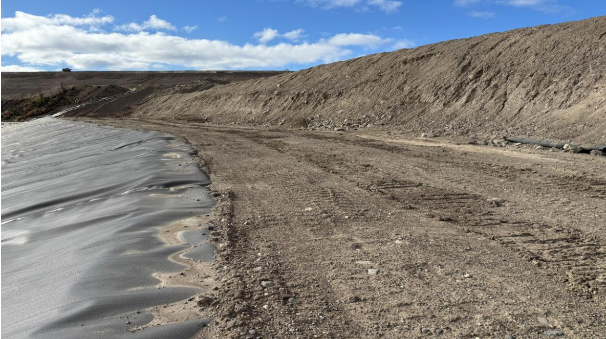
PHOTO 19 – IECD west cut bench crest, looking south (Photo taken on October 15, 2025)
