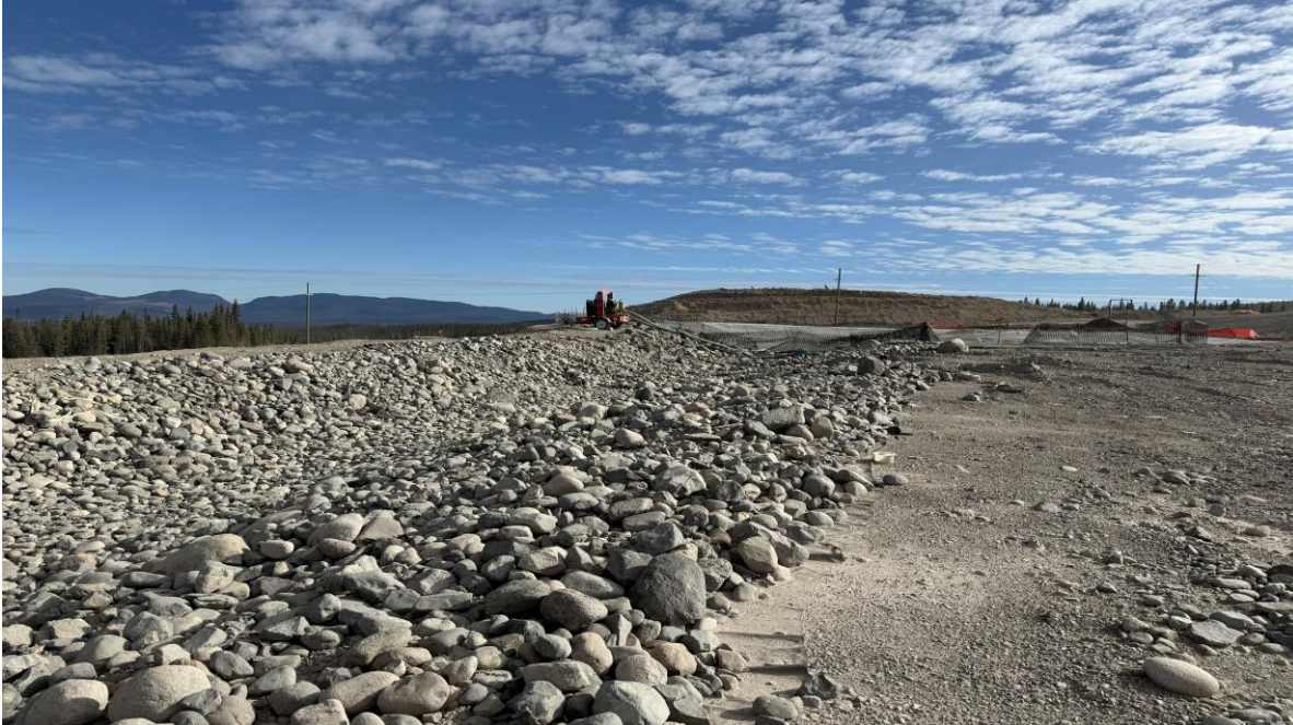
PHOTO 7 – SCP spillway rip rap, looking southeast (Photo taken on October 13, 2025)
