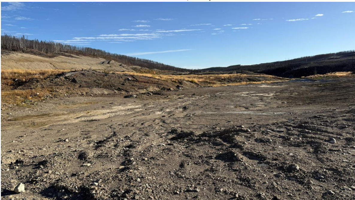
PHOTO 8 – CWTP downstream shell zone, looking northeast (Photo taken on October 13, 2025)
