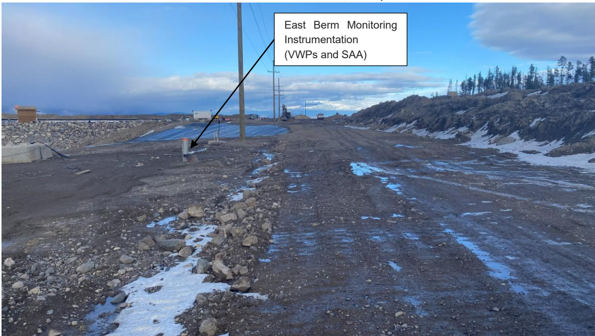
PHOTO 12 – East Berm crest, looking north (Photo taken on October 31, 2025)
