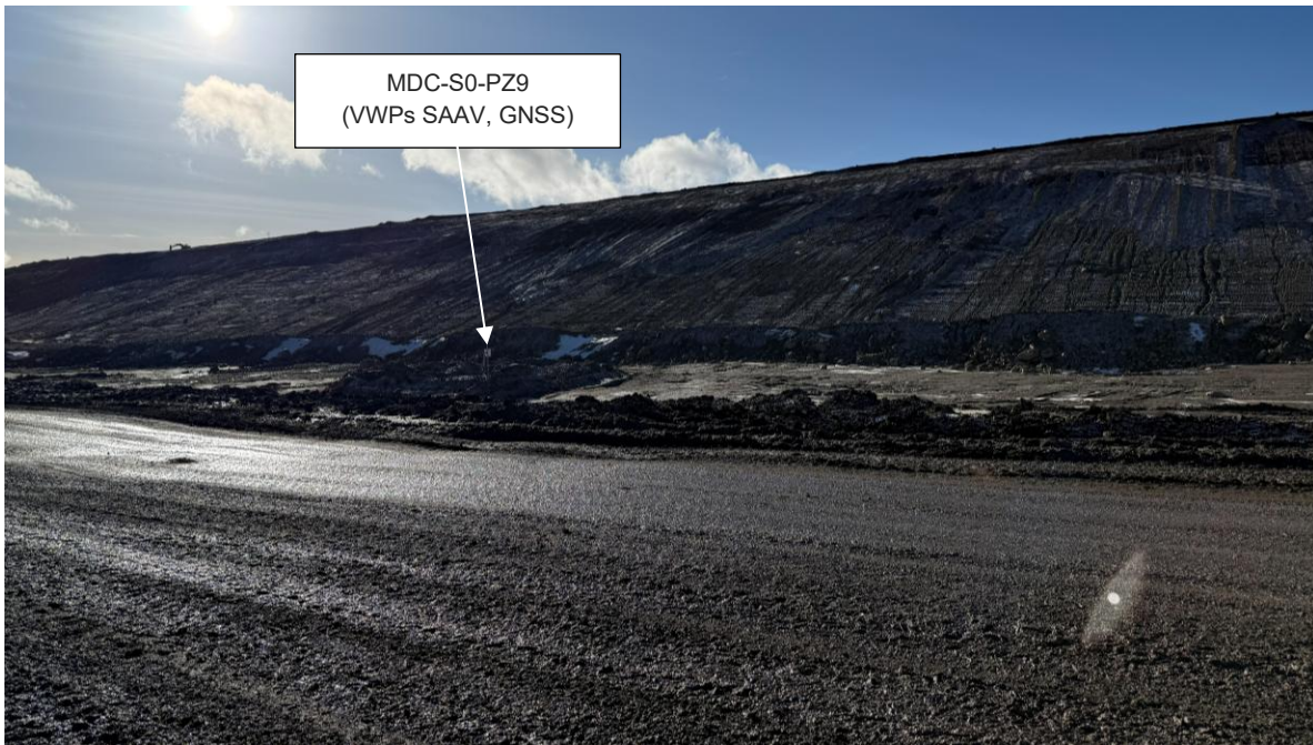
PHOTO 21 – MDC downstream buttress crest and shell zone downstream slope and instrumentation at MDC-S0-PZ9, looking south (Photo taken on November 11, 2025)
