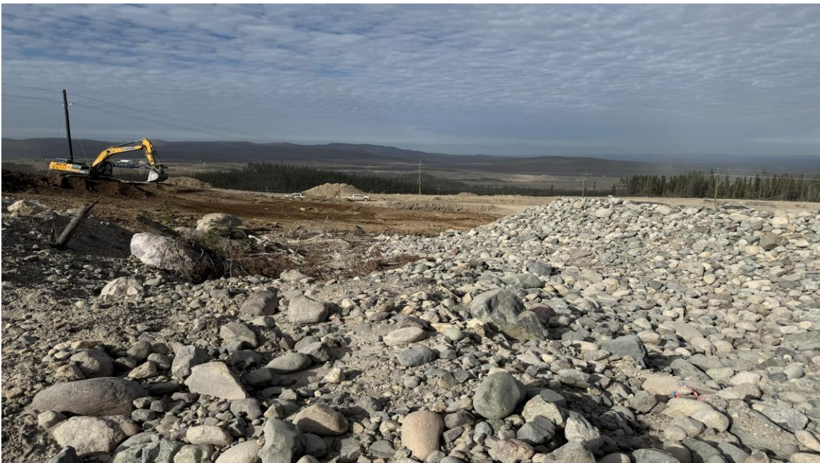
PHOTO 8 – SCP spillway outlet, looking northwest (Photo taken on October 13, 2025)
