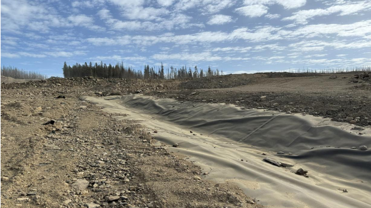
PHOTO 23 – Upstream extent of WCC lining (Photo taken on October 13, 2025)
