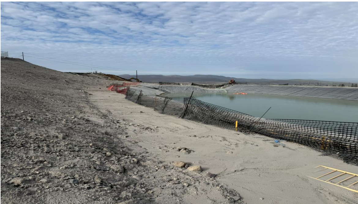
PHOTO 2 – SCP cut slope crest, looking west (Photo taken on October 13, 2025)
