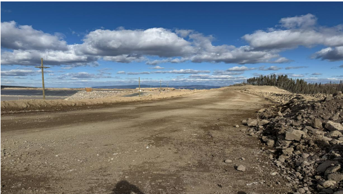
PHOTO 14 – East Berm haul road, looking north (Photo taken on October 11, 2025)
