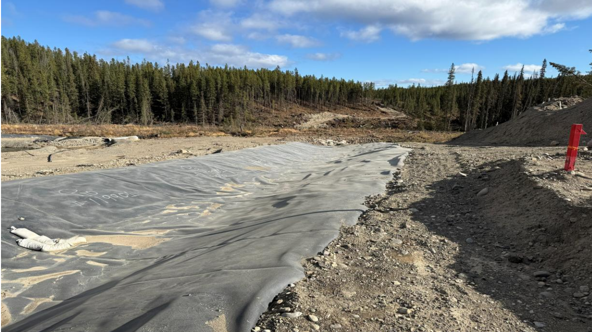
PHOTO 13 – IECD spillway, looking northeast (Photo taken on October 12, 2025)
