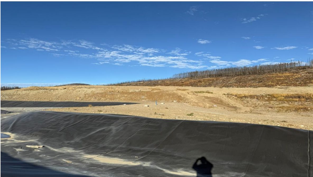
PHOTO 10 – CWTP spillway, looking northwest (Photo taken on October 13, 2025)
