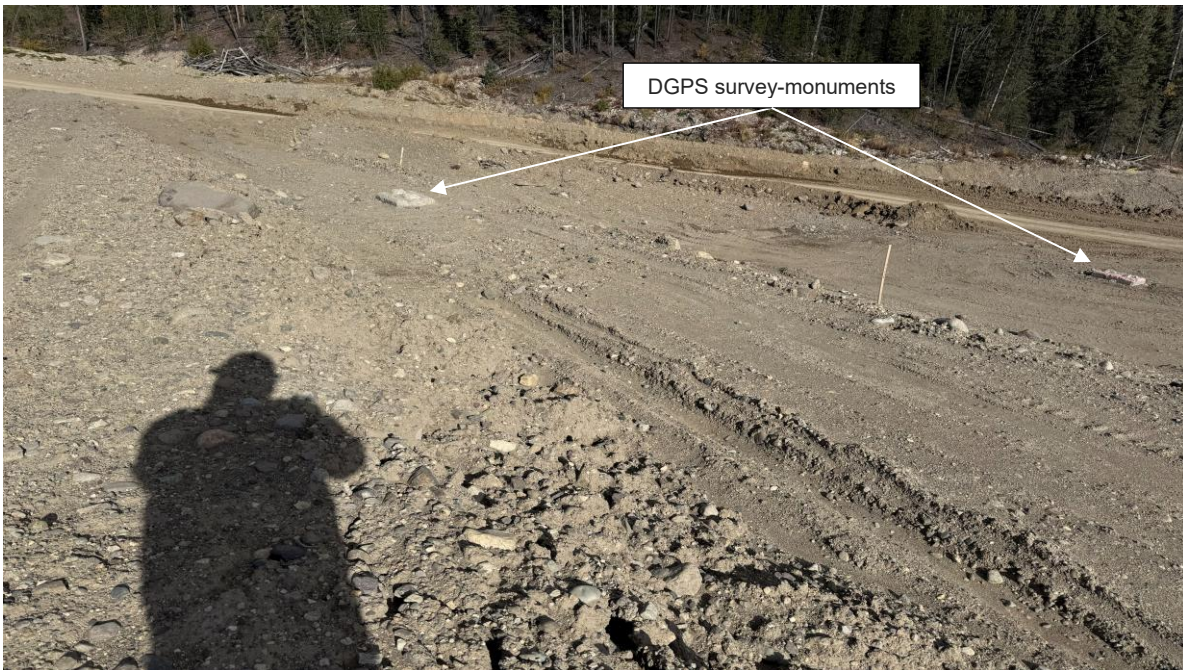
PHOTO 6 – IECD crest, looking north (Photo taken on October 12, 2025)
