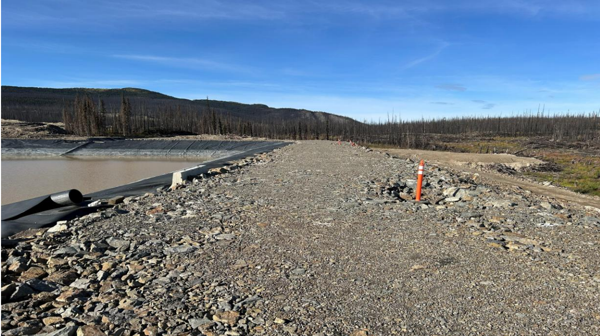
PHOTO 3 – LGO CP northwest crest, looking southwest (Photo taken on September 19, 2025)
