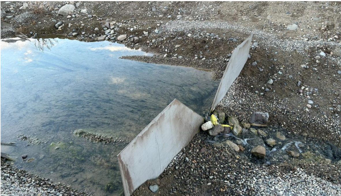
PHOTO 30 – Central foundation drain weir and organic growth (Photo taken on November 3, 2025)
