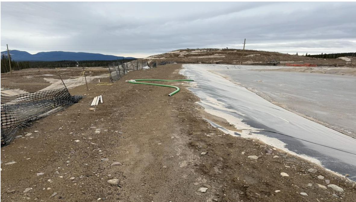
PHOTO 10 – SCP fill crest, looking east (Photo taken on November 12, 2025)
