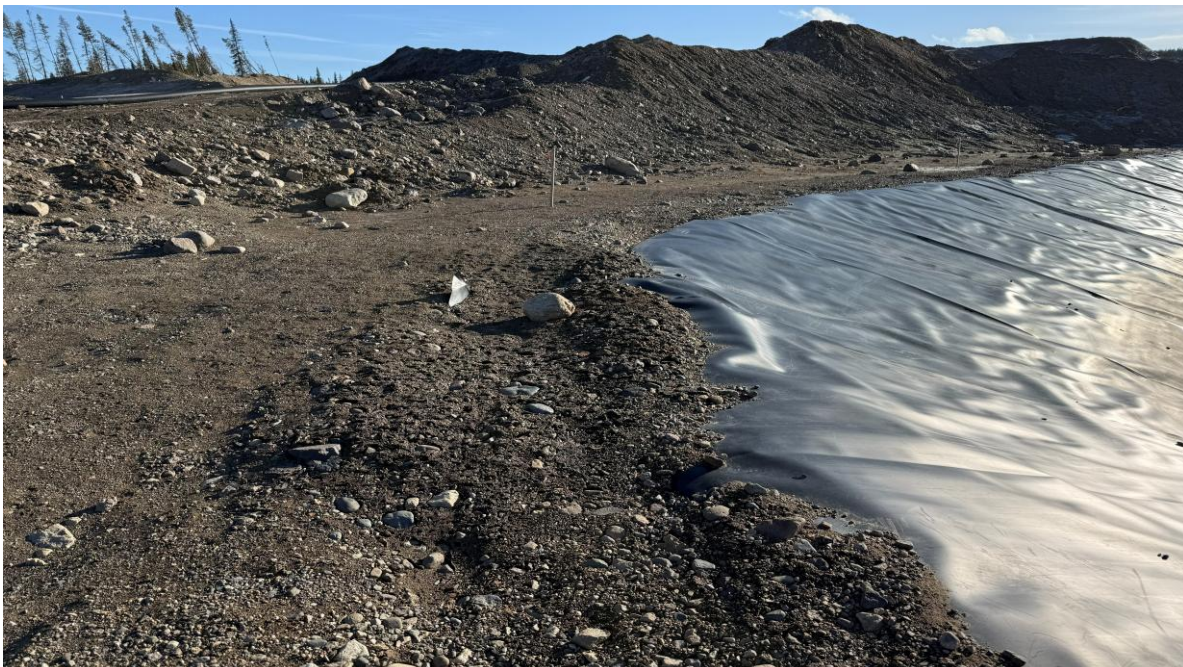
PHOTO 26 – TSF SCP crest at the northeast corner, looking east (Photo taken on November 28, 2025)
