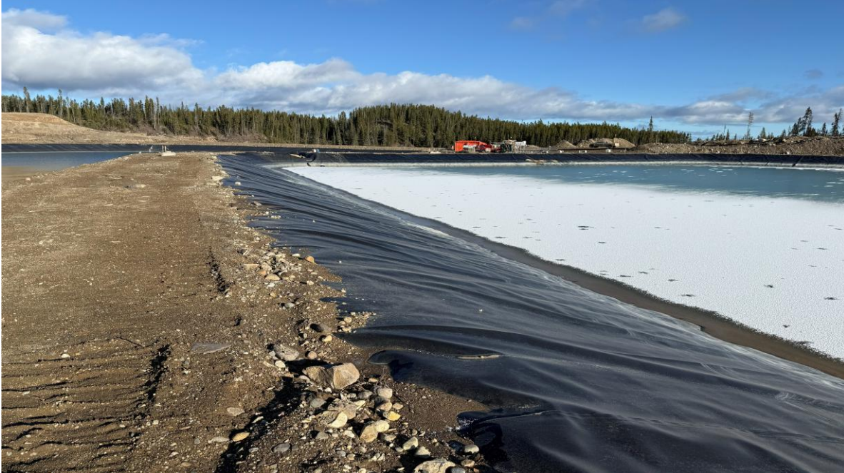
PHOTO 39 – TSF SCP west crest and upstream slope, looking north (Photo taken on November 11, 2025)
