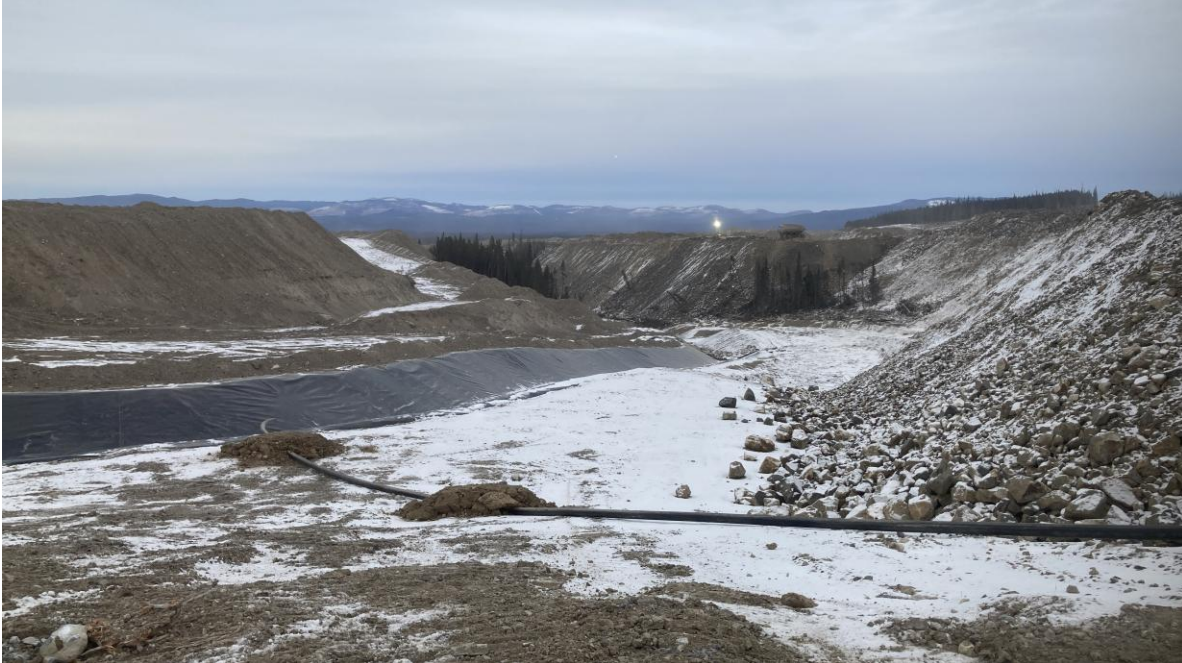
PHOTO 5 – Spillway and North Berm downstream buttress, and IEC pumpback drain line, looking north (Photo taken on November 11, 2025)
