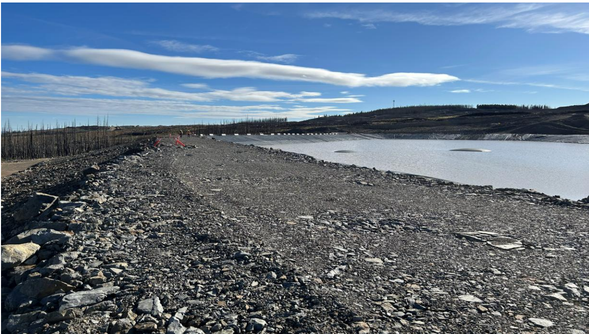
PHOTO 4 – LGO CP northwest crest, looking northeast (Photo taken on September 19, 2025)
