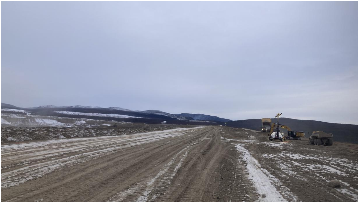
PHOTO 13 – MDC crest, looking northwest (Photo taken on November 28, 2025)
