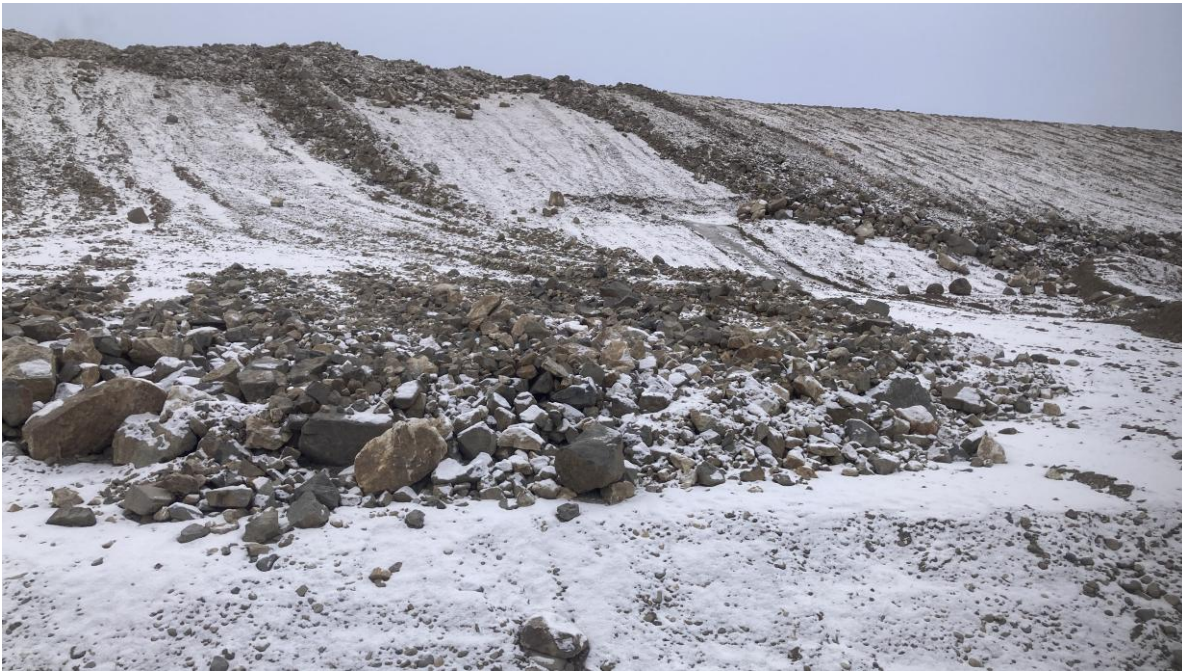
PHOTO 23 – Downstream buttress downstream slope surface erosion protection with NAG waste rock, looking west (Photo taken on November 28, 2025)
