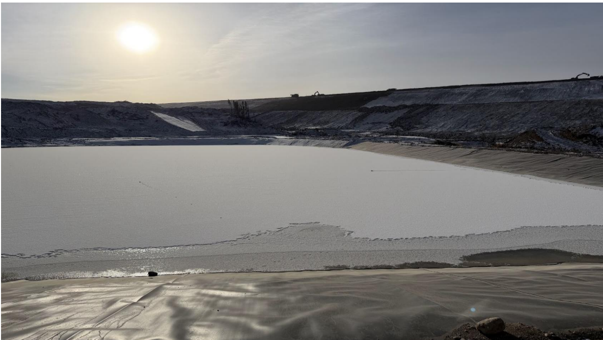
PHOTO 22 – TSF SCP looking south (Photo taken on November 28, 2025)
