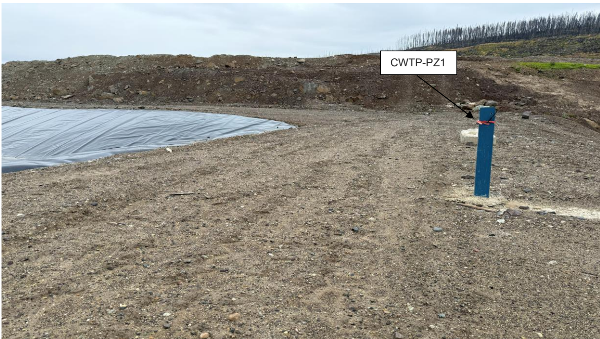
PHOTO 26 – CWTP berm crest and instrumentation (VWPs), looking northwest (Photo taken on September 14, 2025)
