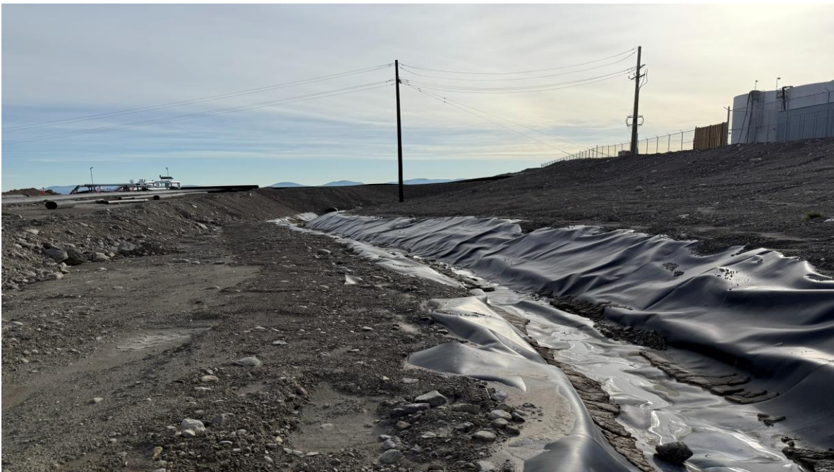
PHOTO 18 – NCC looking down-channel, looking east (September 15, 2025)
