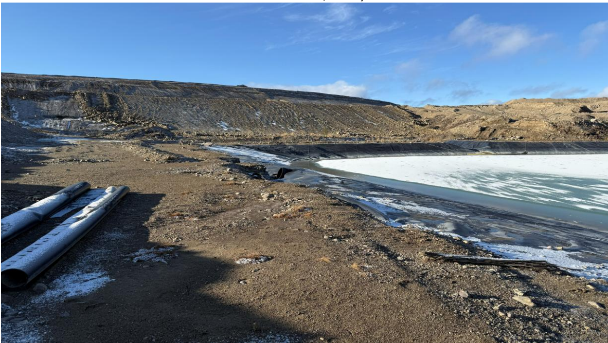
PHOTO 32 – TSF SCP southeast cut crest, looking southwest (Photo taken on November 11, 2025)
