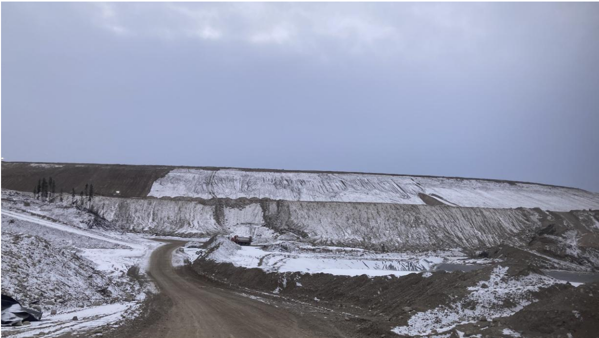
PHOTO 18 – Downstream slopes of MDC and Stage 1 buttress, looking southwest (Photo taken on November 11, 2025)
