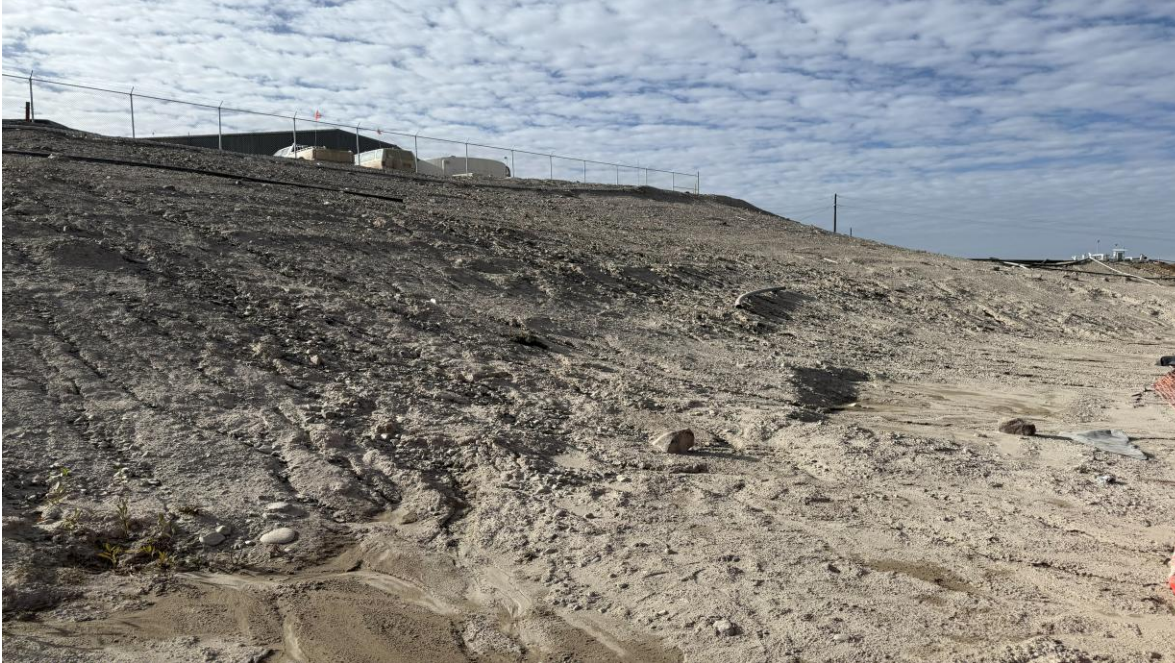
PHOTO 3 – SCP cut slope above crest erosion, looking southwest (Photo taken on October 13, 2025)
