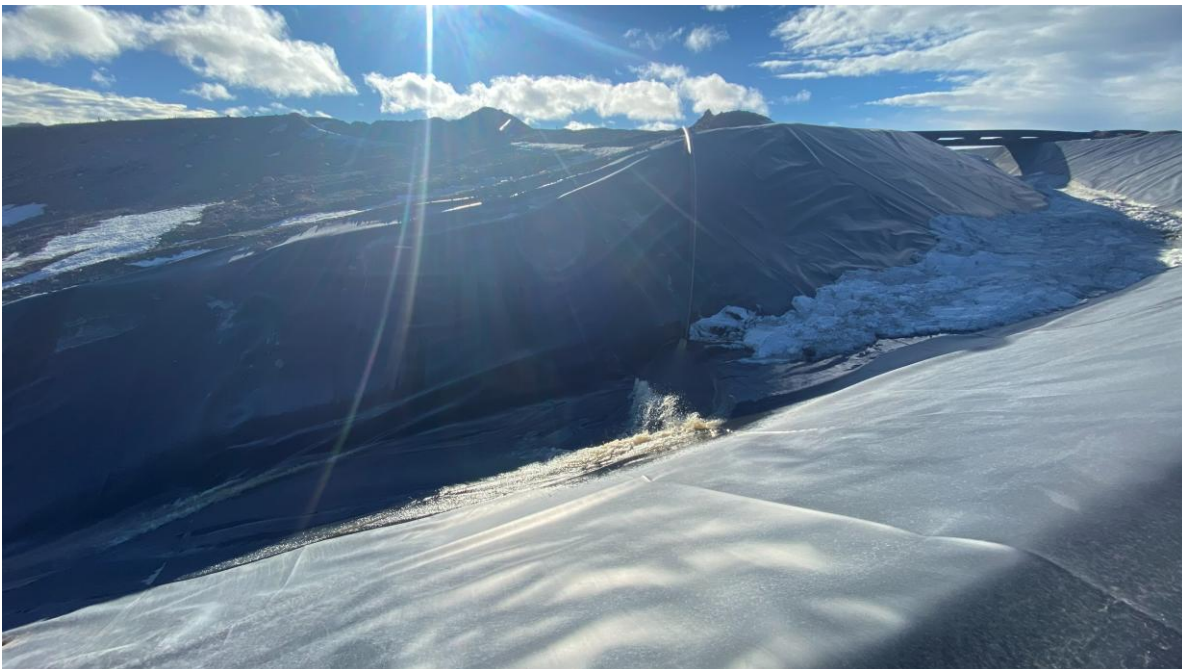
PHOTO 6 – Spillway just down-channel of inlet, looking up-channel (south) (Photo taken on October 31, 2025)
