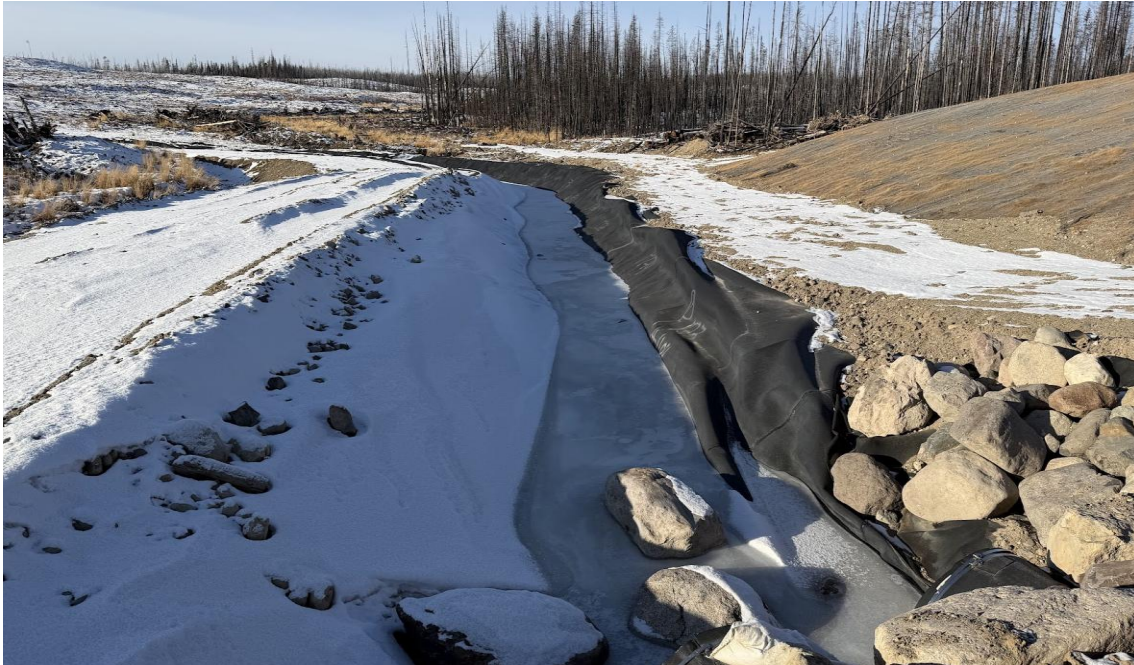
PHOTO 23 – NDC upstream of C-trail crossing, looking west (Photo taken on November 28, 2025)
