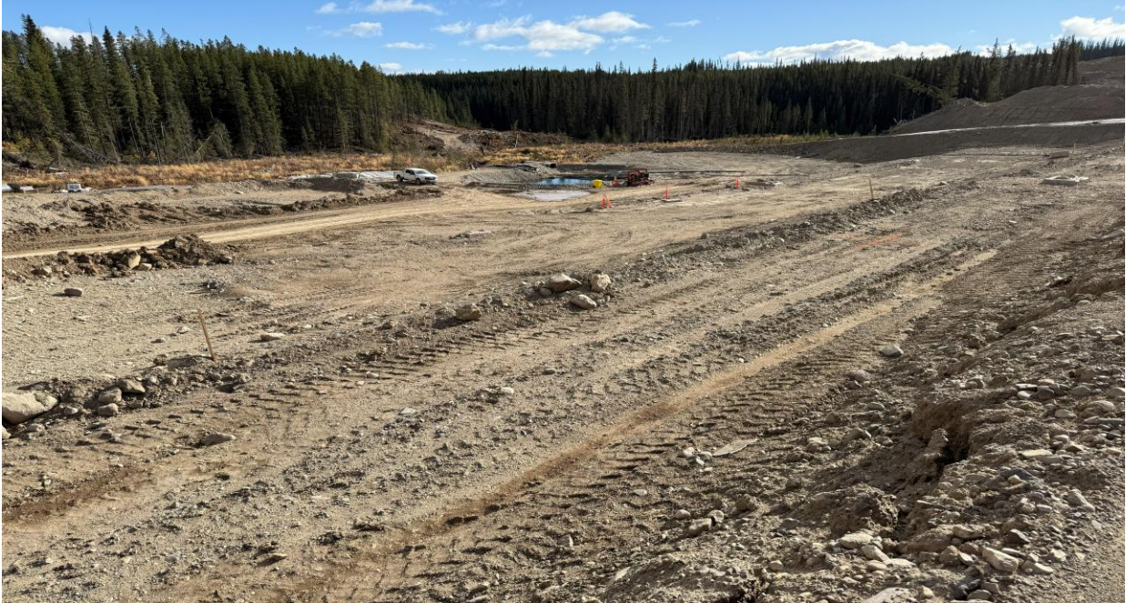
PHOTO 11 – IECD downstream bench, looking southeast (Photo taken on October 12, 2025)
