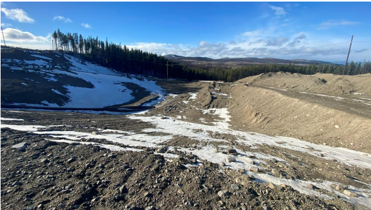
PHOTO 22 – West Berm downstream slope, looking west (Photo taken on October 31, 2025)
