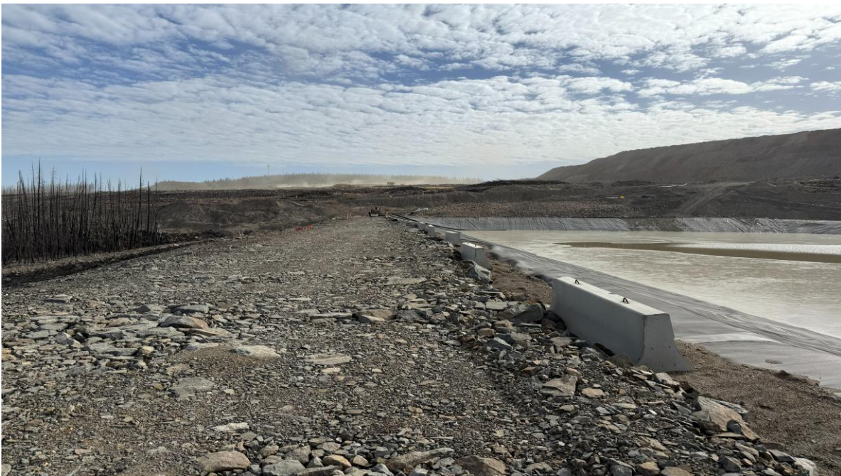
PHOTO 2 – LGO CP northeast crest, looking southeast (Photo taken on October 13, 2025)
