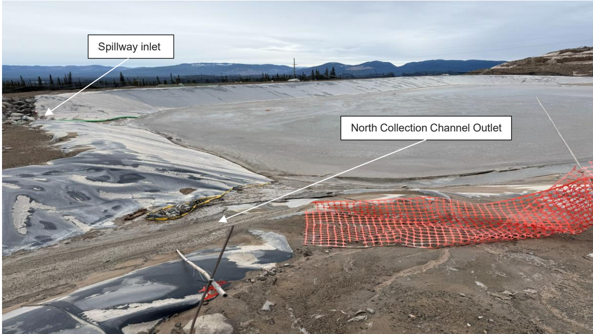
PHOTO 5 – SCP spillway inlet and NCC inlet, looking northeast (Photo taken on November 12, 2025)
