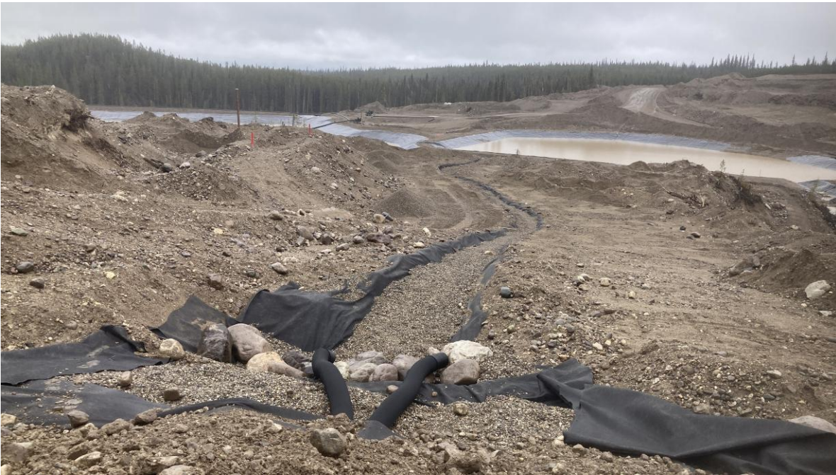
PHOTO 35 – Downstream channel of the west foundation drain outlet towards the IECD, looking northeast (Photo taken on May 17, 2025)
