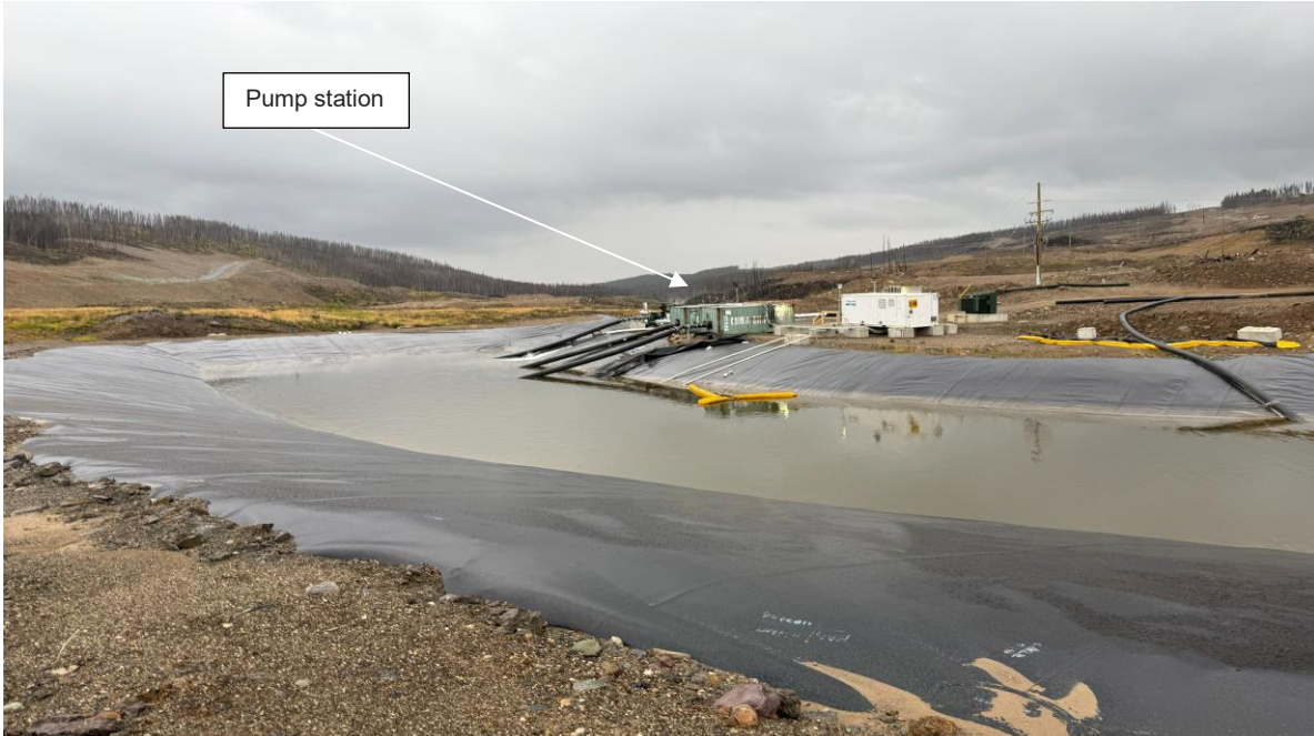
PHOTO 3 – CWTP basin slopes and CDS pump station, looking northwest (Photo taken on September 14, 2025)
