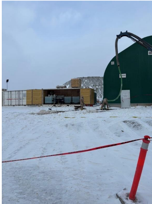
Photo 5: Cleanup (Vac Truck) photo (12/6/2025)
