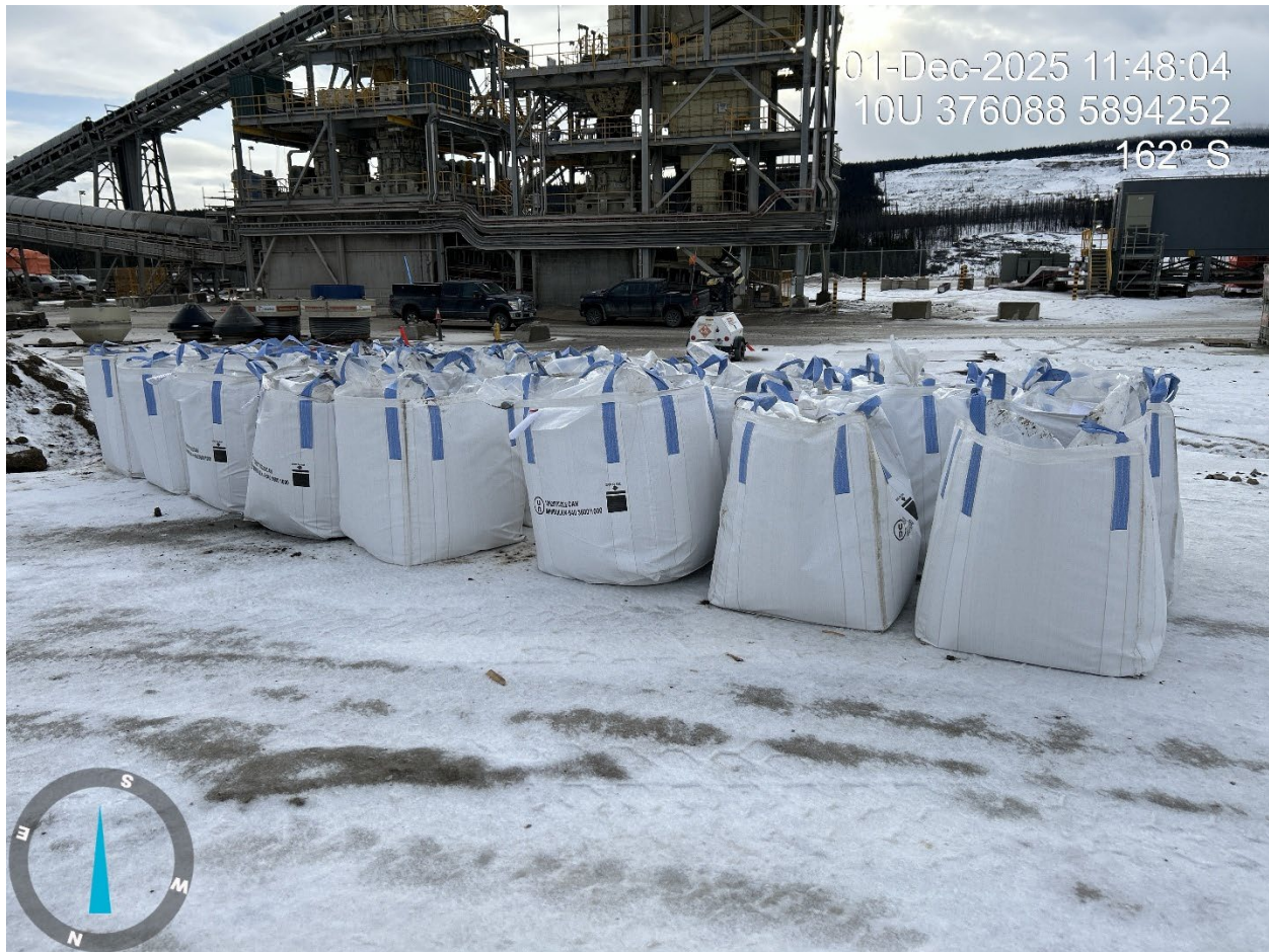
Image 6: Lined bags containing contaminated material prior to transfer to hazardous containment area for holding.
