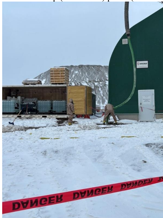
Photo 6: Cleanup (Vac Truck) photo (12/6/2025)
