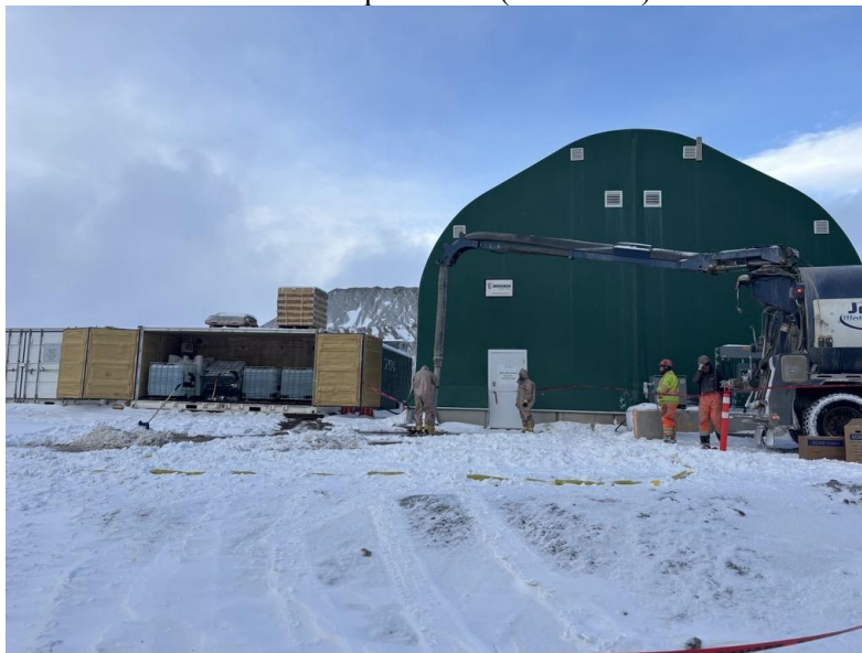
Photo 4: Cleanup (Vac Truck) photo (12/6/2025)
