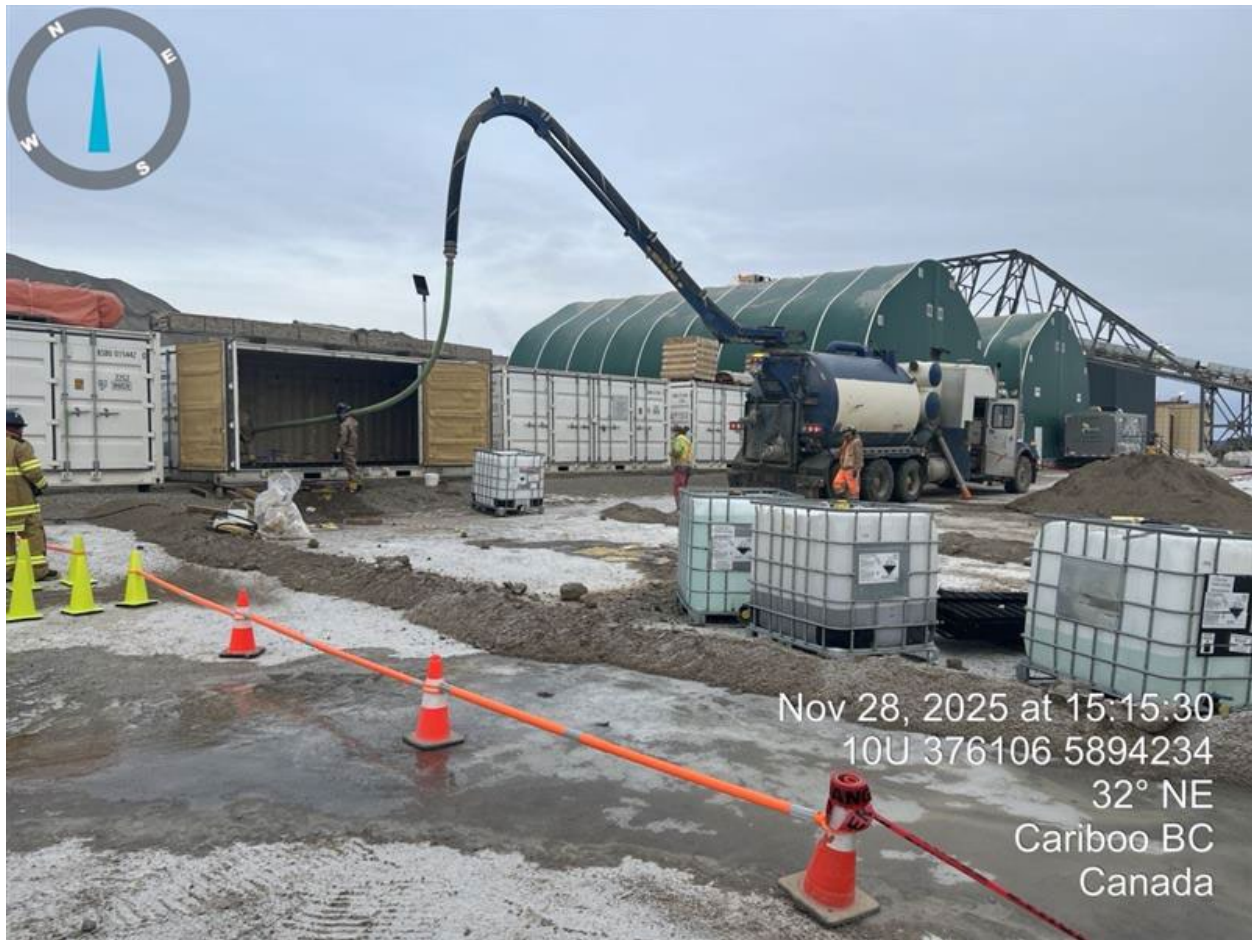
Image 4: Clean up of caustic soda within sea-canister with containment.
