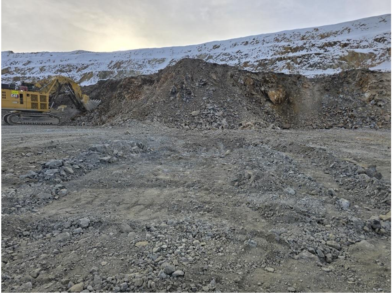
Photo 3: After image of cleaned up spill area (in daylight)
