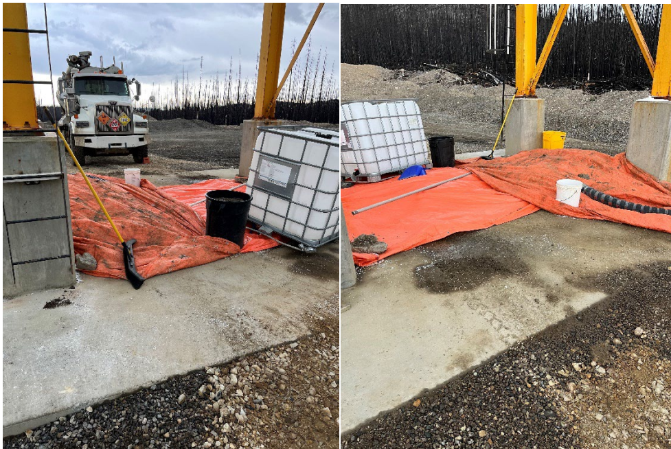
Photos 2 & 3: Spill Cleanup In Progress
