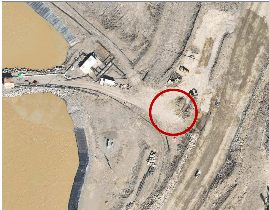
Photo 8: Drone Photo of Spill Location at WMP Booster 1
