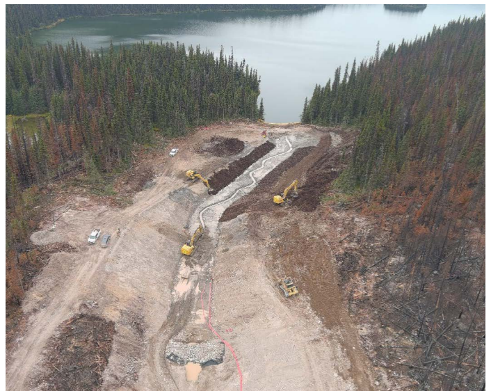
Construction of the stream connecting Lake 15 and Lake 16
