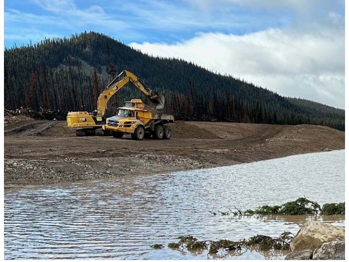
Water in the new stream connecting Lake 15 and Lake 16
