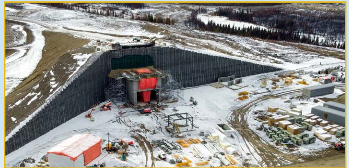
Primary Crusher Vault and Mechanically Stabilized Earth (MSE) Wall - April 2024
